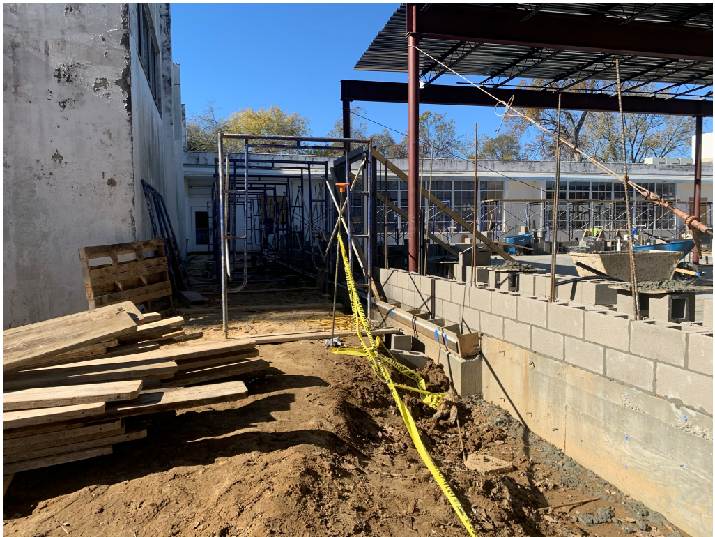
Figure 2 – CMU installation is ongoing
