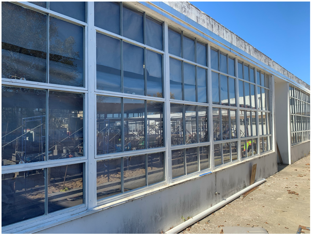
Figure 7 – SE side of Existing Glazing Installed
