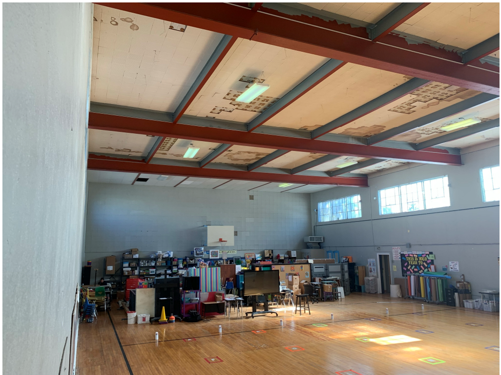
Figure 8 – Gymnasium Ceiling Removed
