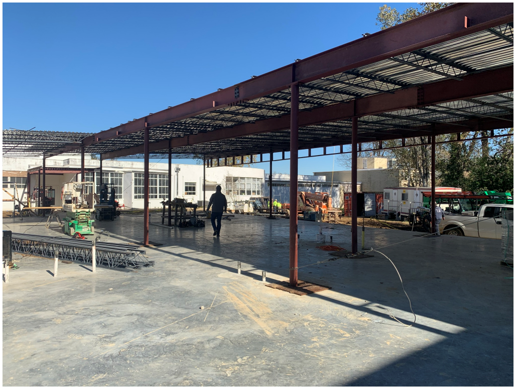
Figure 5 – Remainder of Steel work is awaiting CMU block installation
