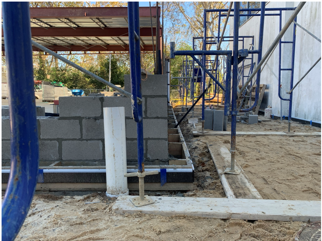
Figure 6 – West Corner of Addition
