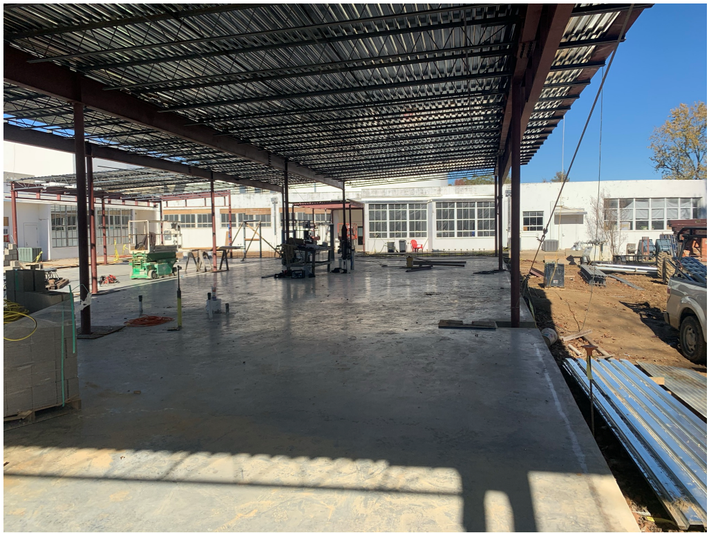
Figure 3 – Roof Decking installed over ceiling joists
