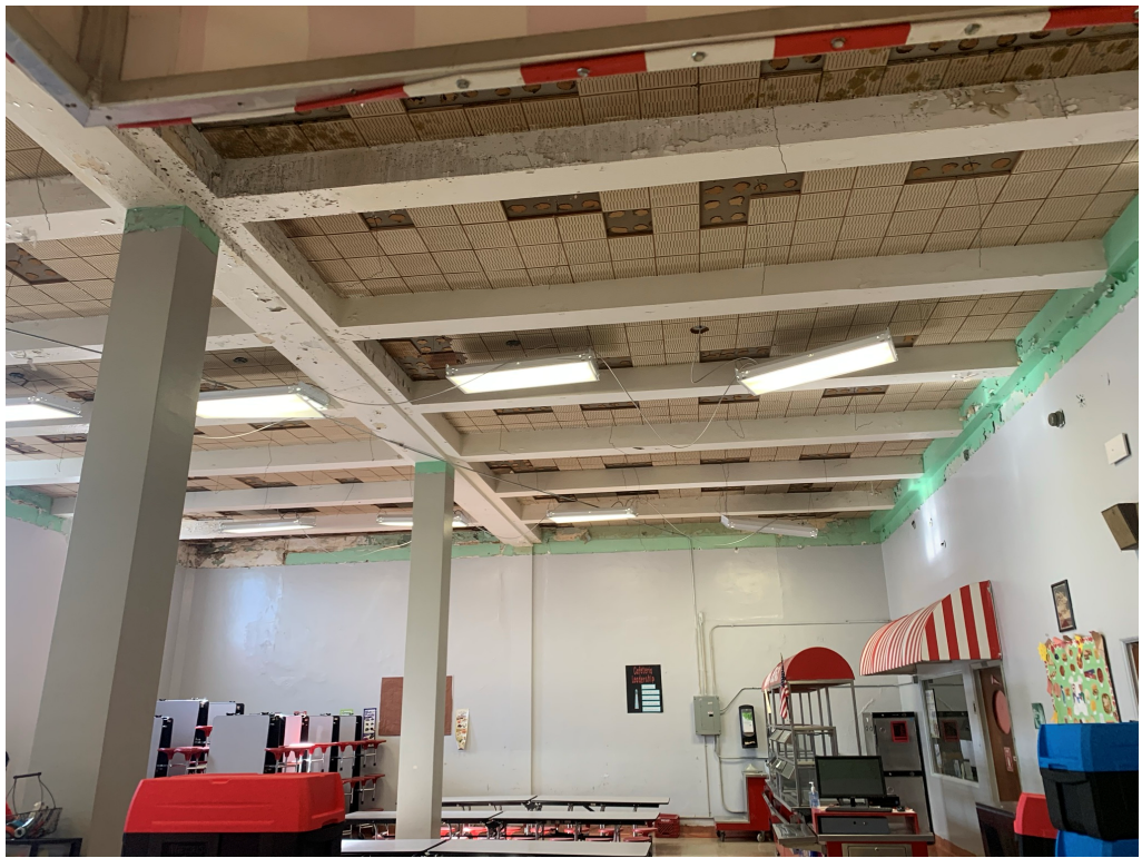
Figure 9 – Cafeteria Ceiling Removed
