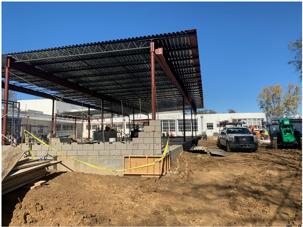
Figure 1 – South Corner of Addition
