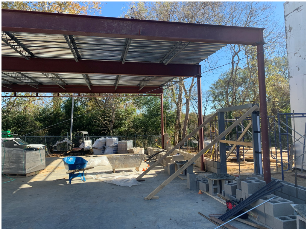
Figure 4 – Remainder of Steel work is awaiting CMU block installation
