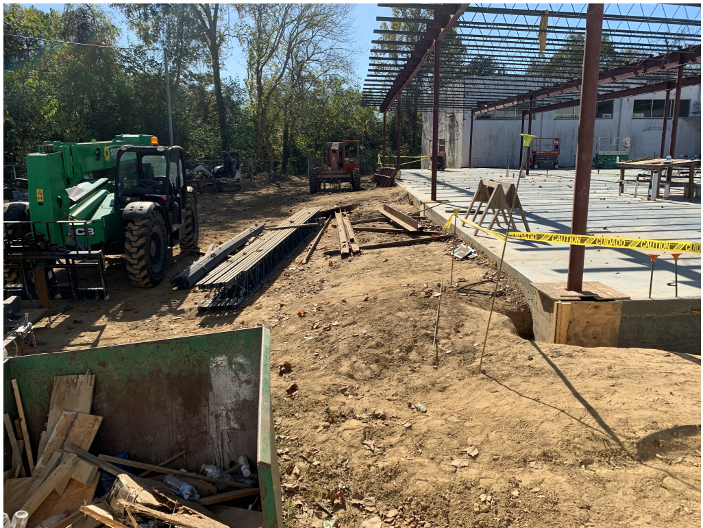
Figure 4 – Steel Erected over Newly poured Slab
