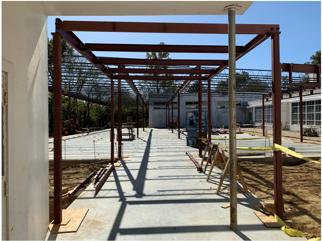
Figure 1 – Entry to New Addition Through Passage 116
