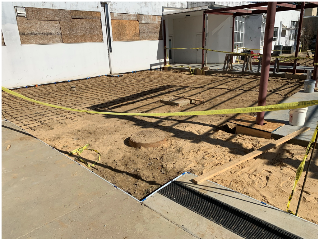
Figure 12 – Select Fill Installed at To-Be Location of New Sidewalks
