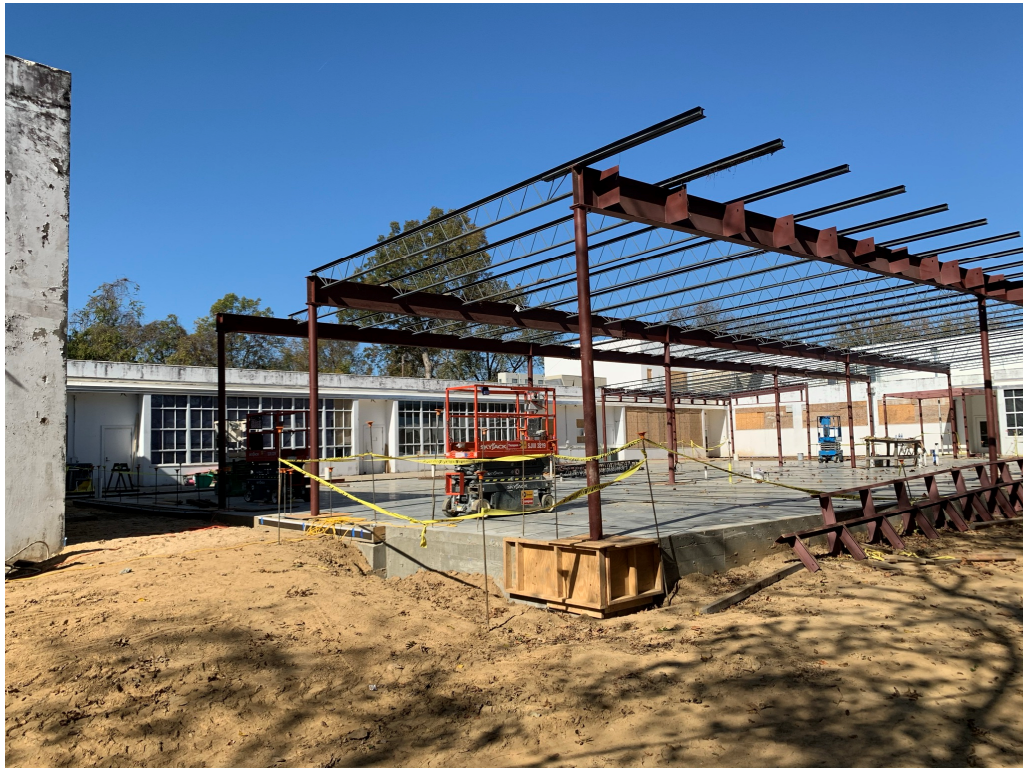
Figure 7 – Steel Erected over Newly poured Slab
