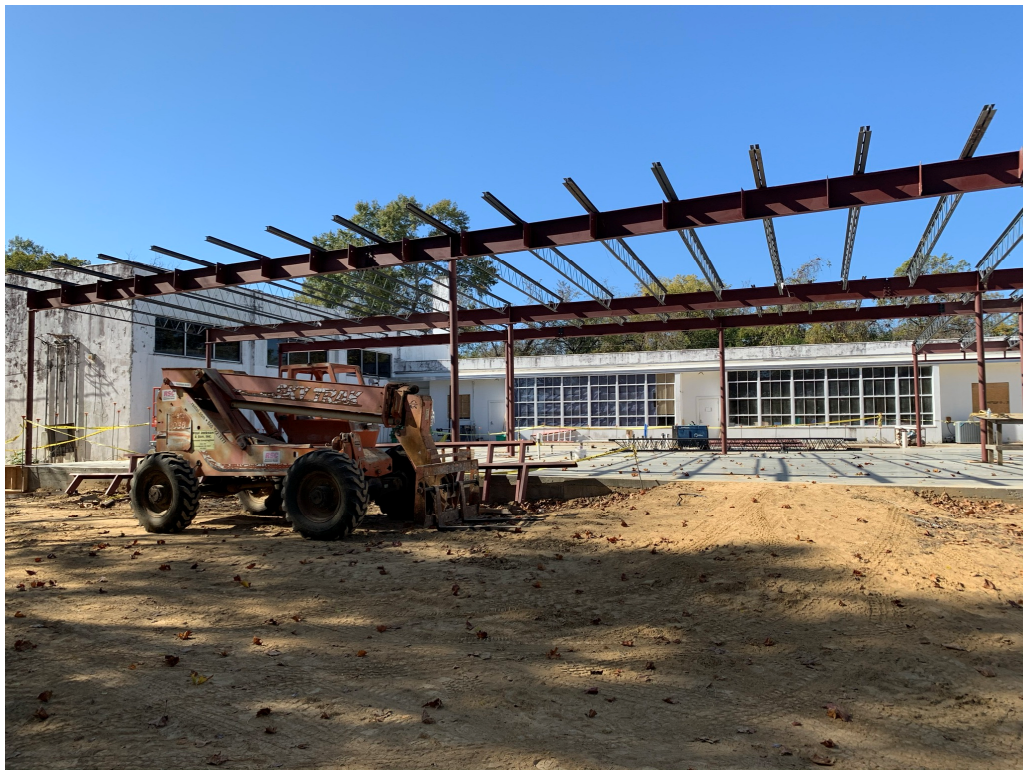
Figure 6 – Steel Erected over Newly poured Slab
