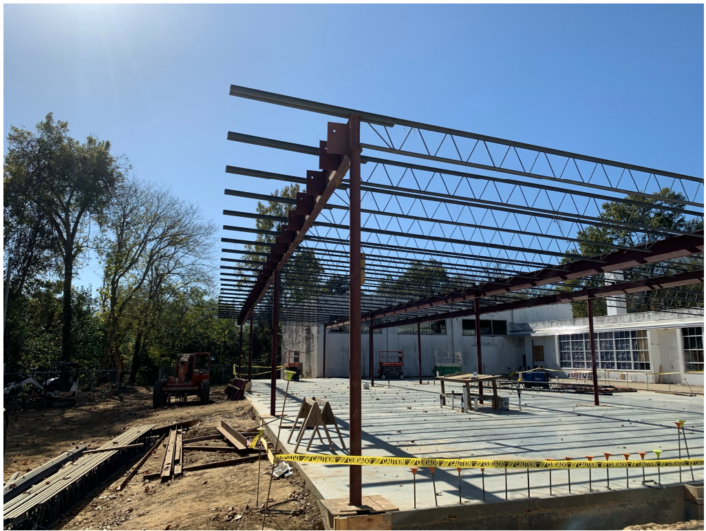
Figure 3 – Steel Erected over Newly poured Slab
