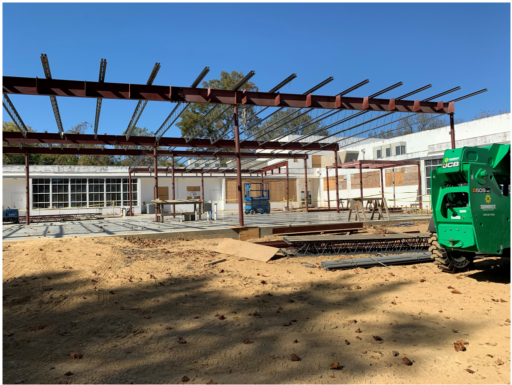
Figure 5 – Steel Erected over Newly poured Slab
