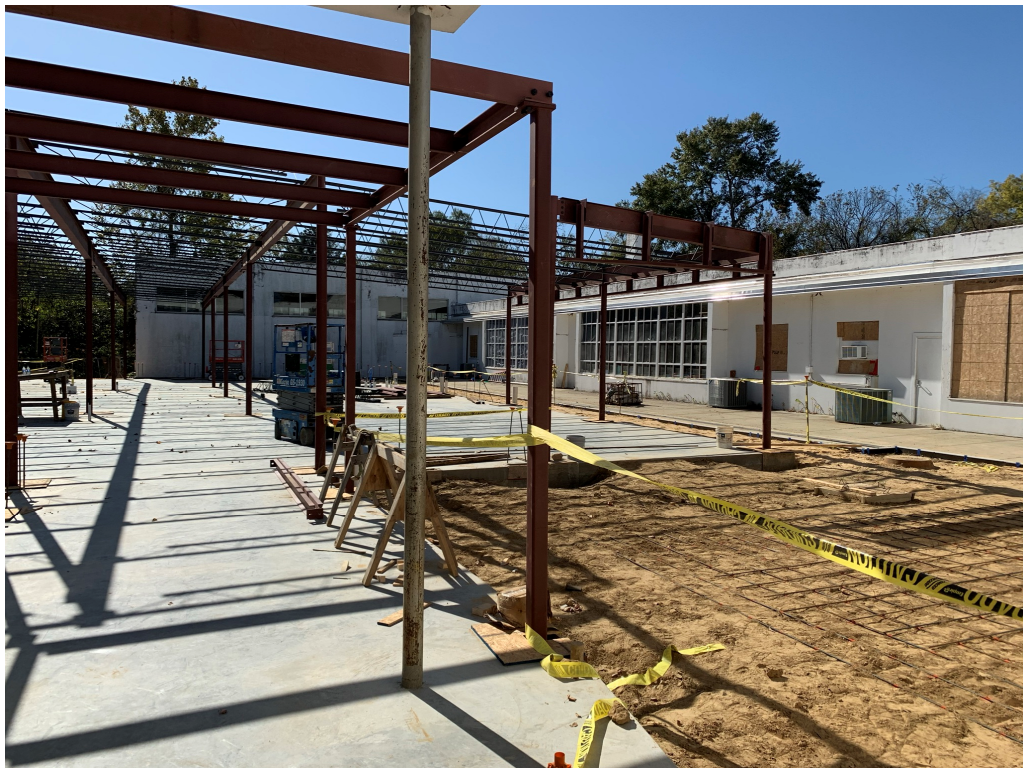
Figure 2 – Steel Erected over Newly poured Slab
