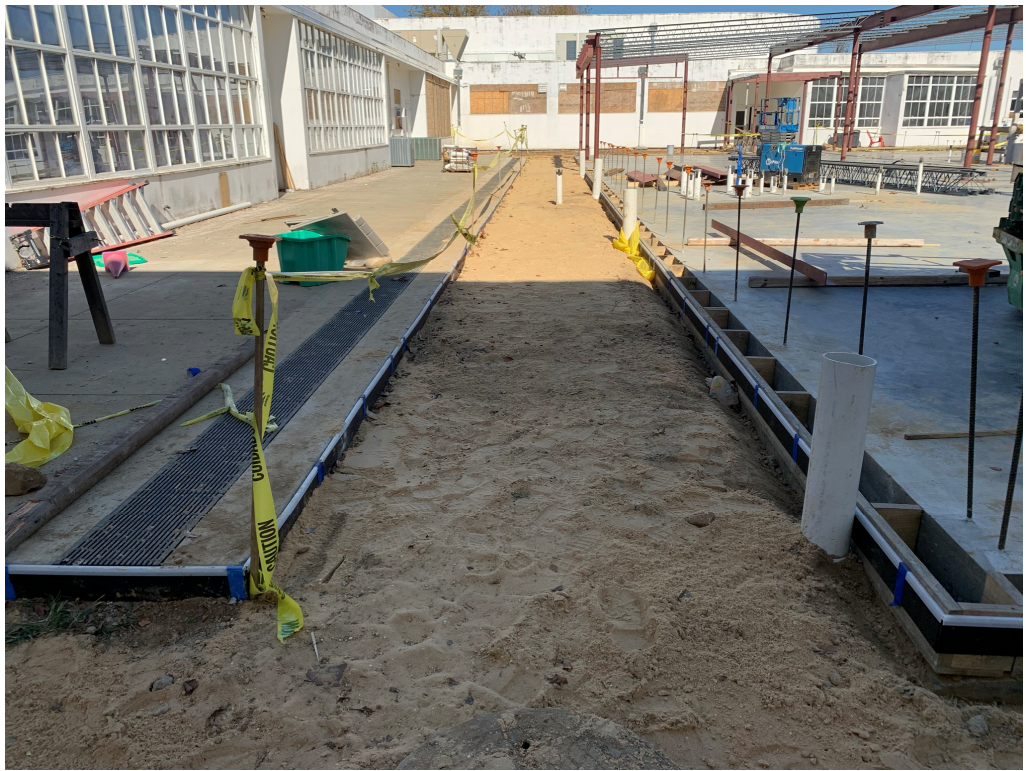
Figure 9 – Select Fill Installed at To-Be Location of New Sidewalks
