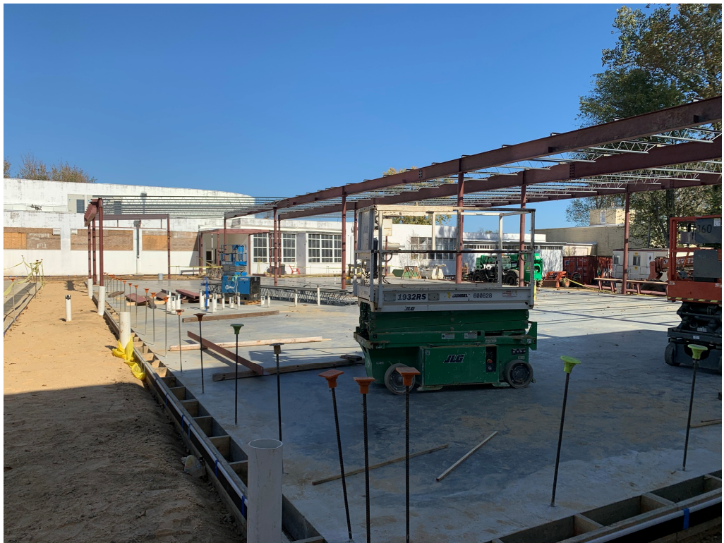
Figure 10 – Steel Erection is Ongoing
