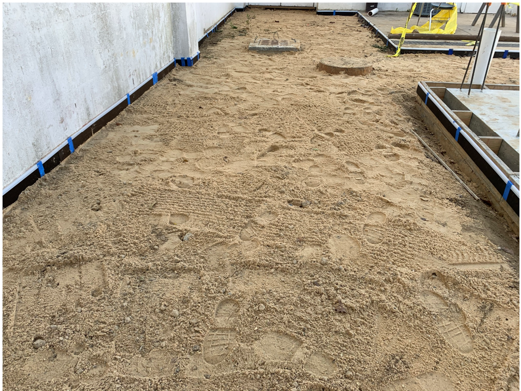
Figure 8 – Select Fill Installed at To-Be Location of New Sidewalks
