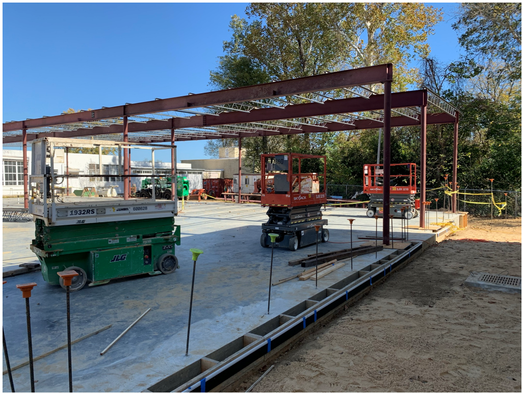
Figure 11 – Steel Erection is Ongoing
