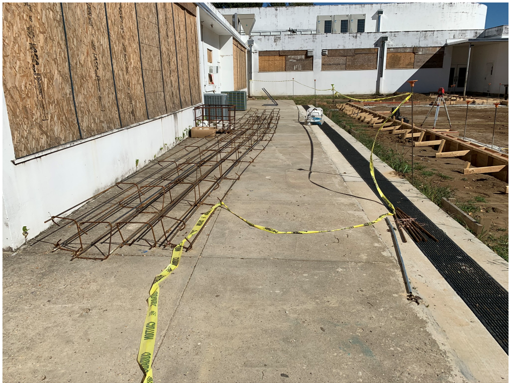
Figure 8 – Rebar Tied and Ready for Install
