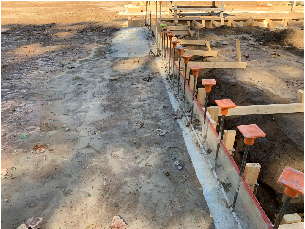
Figure 4 – Formed Up Footings
