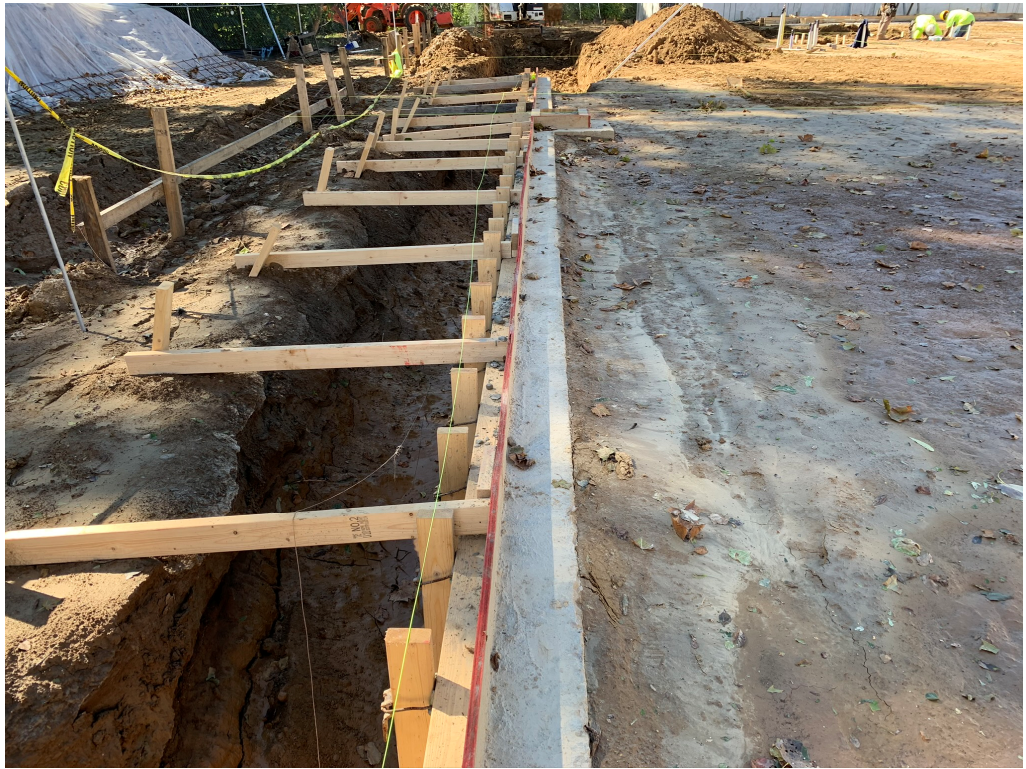
Figure 3 – Formed Up Footings
