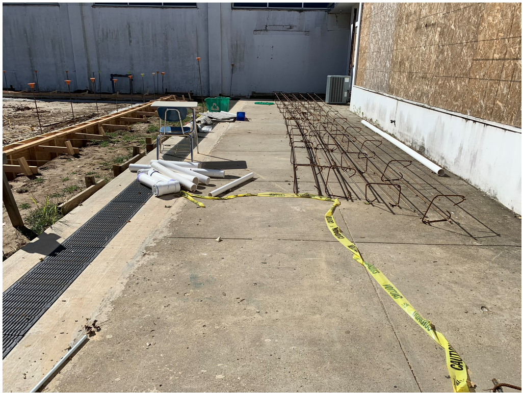
Figure 7 – Rebar Tied and Ready for Install
