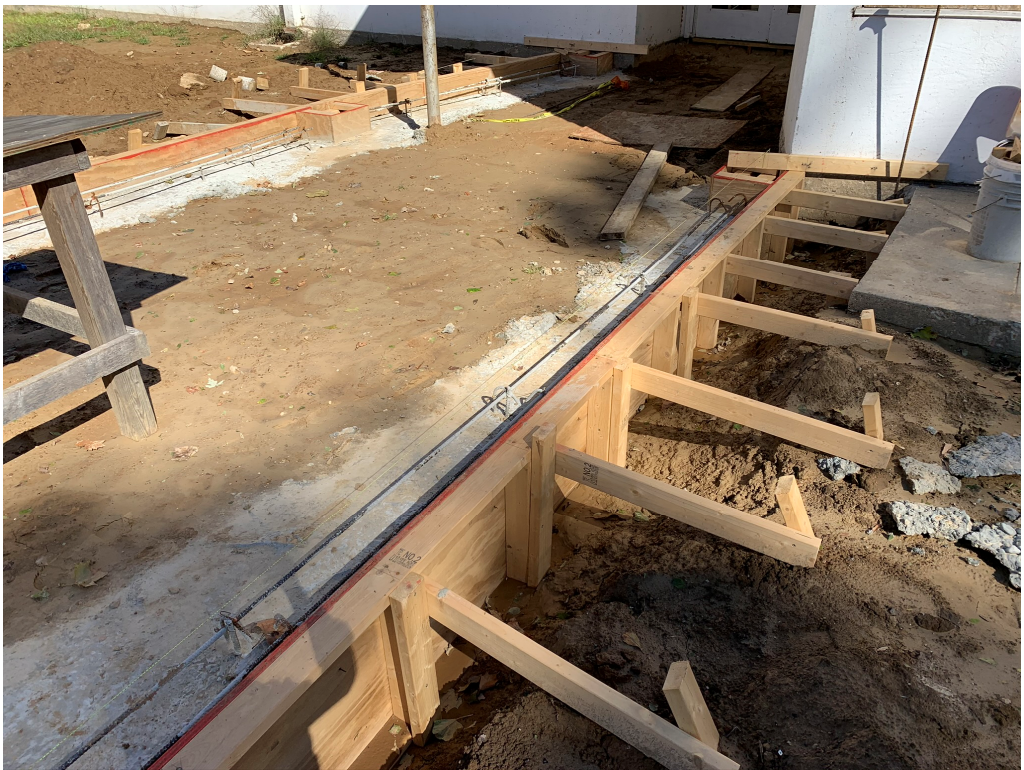
Figure 6 – Formed Up Footings
