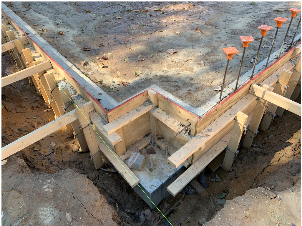
Figure 2 – Formed Up Footings
