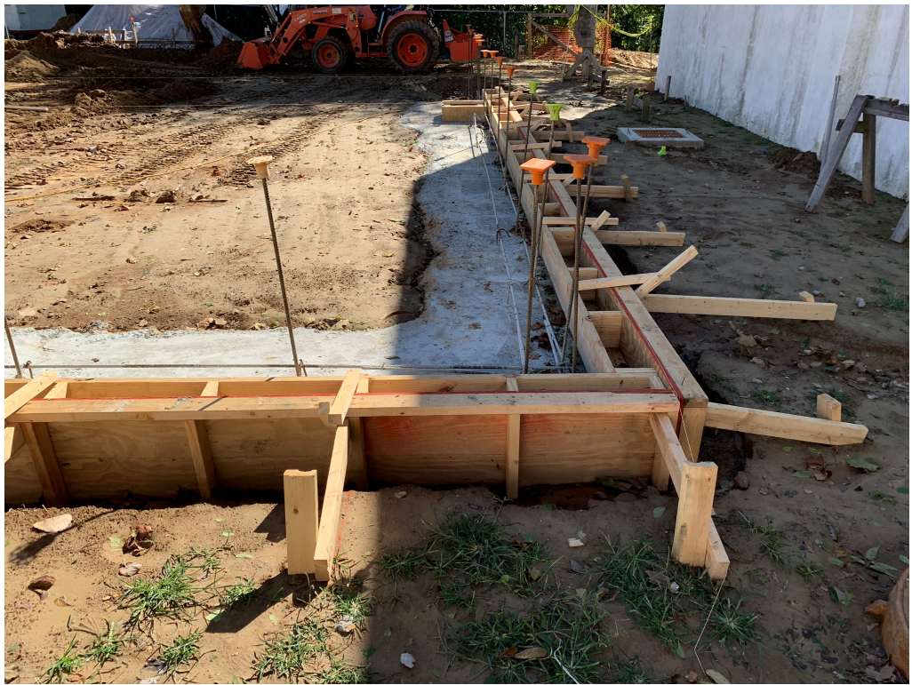
Figure 9 – Formed Up Footings
