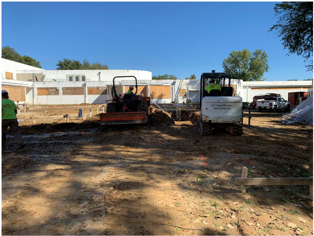
Figure 1 – Dirt Work at Slab
