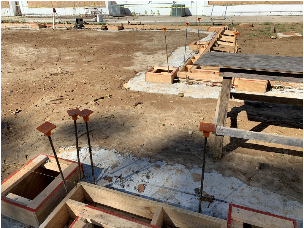
Figure 5 – Formed Up Footings
