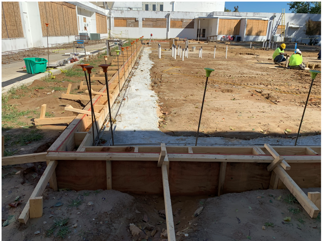
Figure 10 – Formed Up Footings
