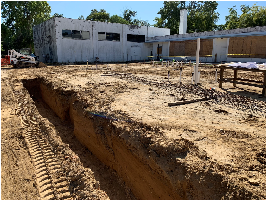
Figure 8 – Footing Trenches
