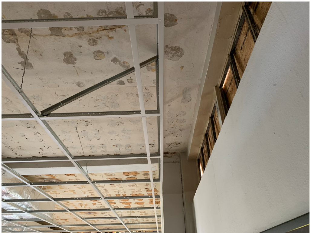
Figure 6 – Grid Install with Reveal for Glazing
