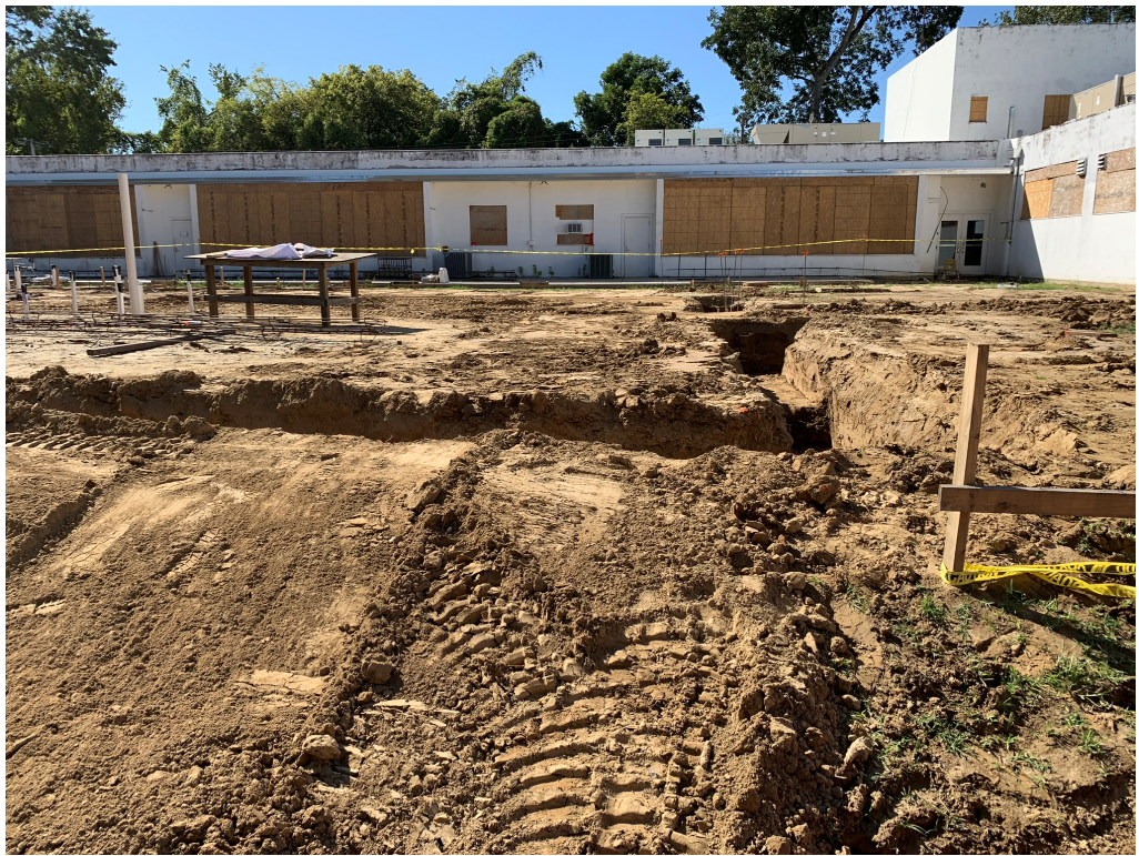
Figure 7 – Footing Trenches
