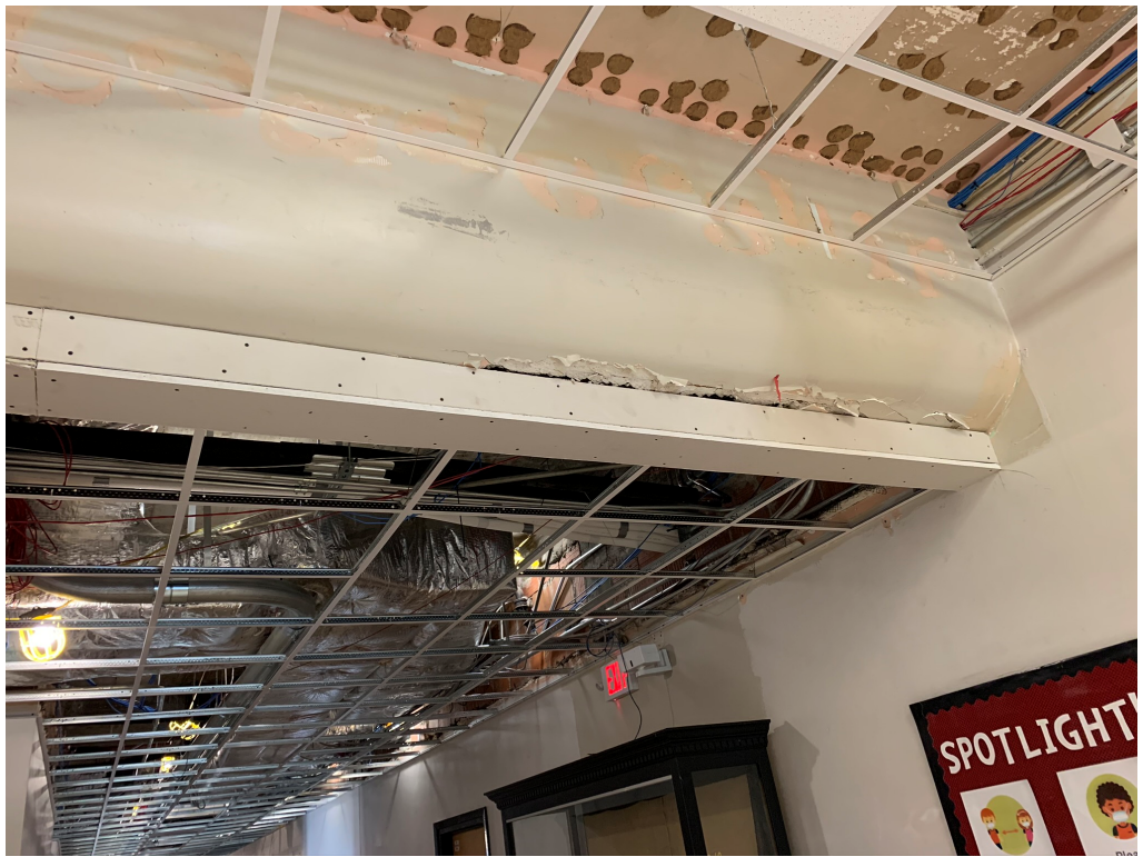
Figure 13 – Grid Install @ Furr-Down
