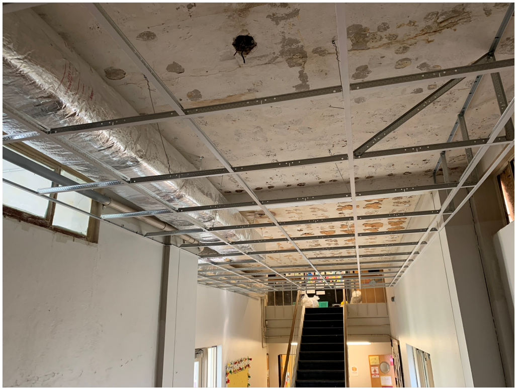
Figure 5 – Grid Install
