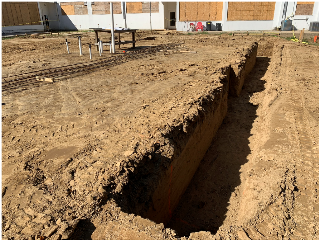
Figure 9 – Footing Trenches
