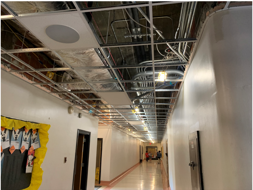
Figure 2 – Grid Install
