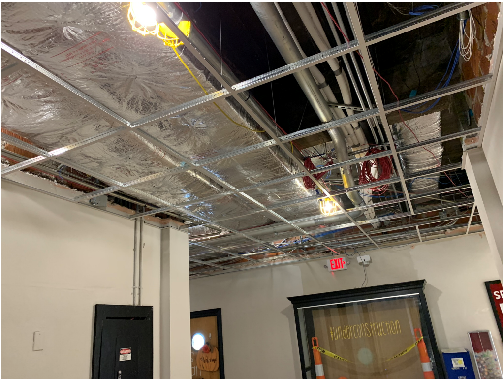
Figure 12 – Grid Install at Hallway Junction
