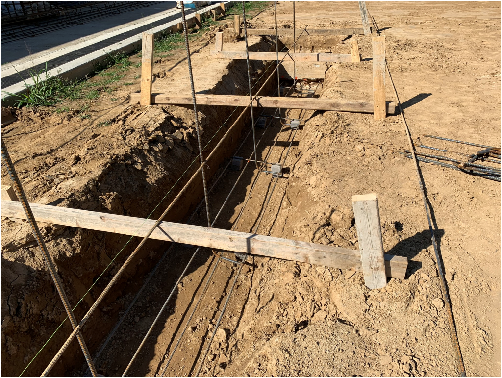
Figure 11 – Footing Trenches
