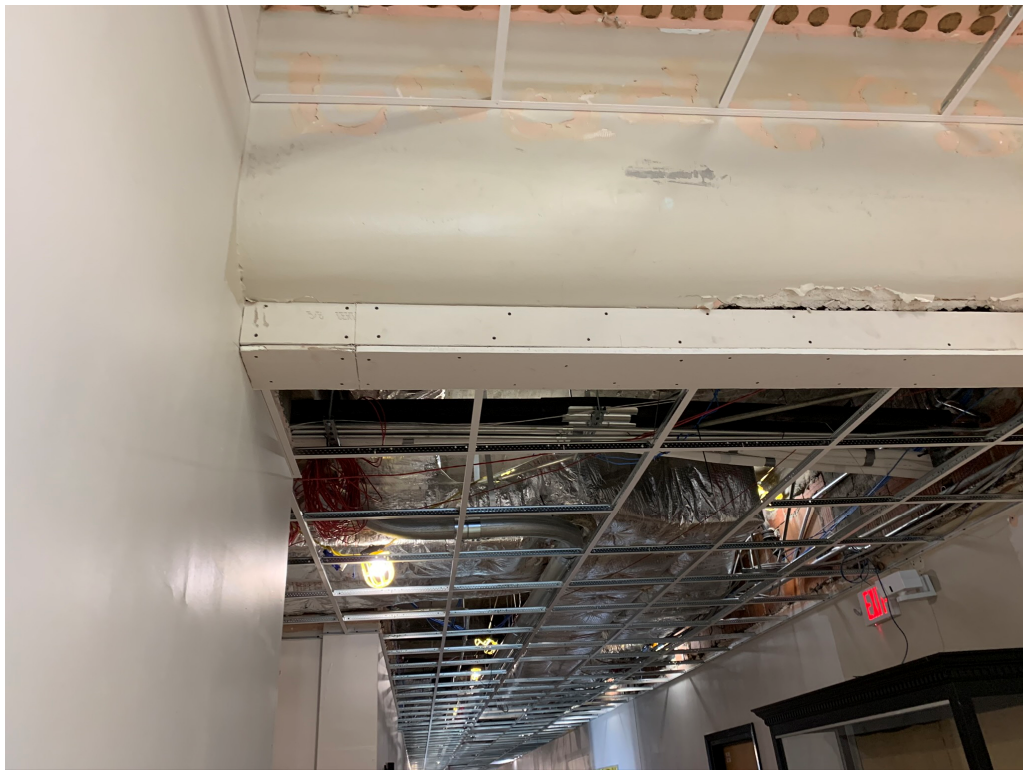
Figure 14 – Grid Install @ Furr-Down
