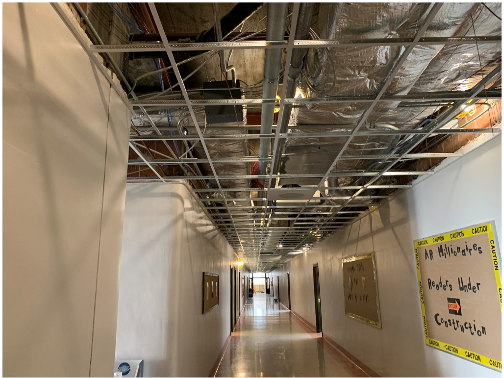
Figure 15 – Grid Install
