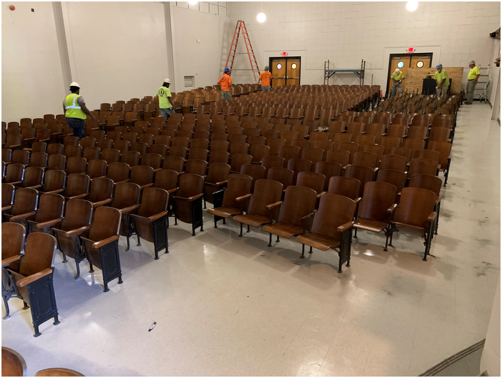
Figure 1 – Auditorium Seating Installation
