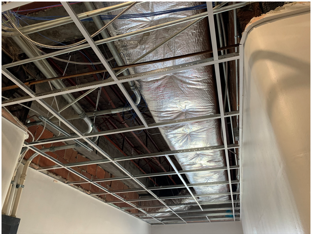
Figure 16 – Grid Install
