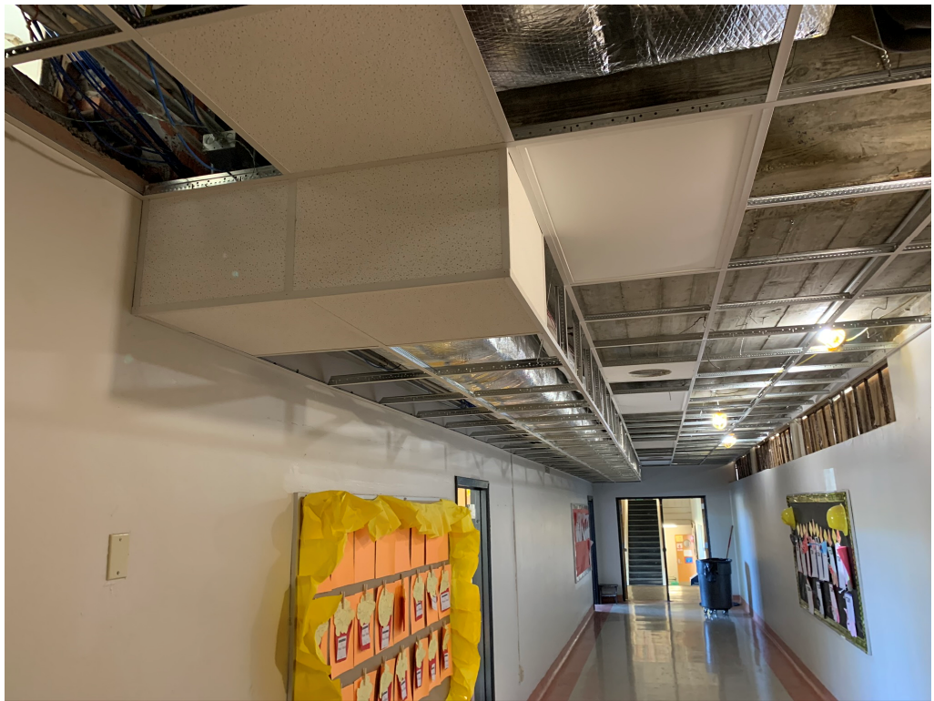
Figure 4 – Grid Install
