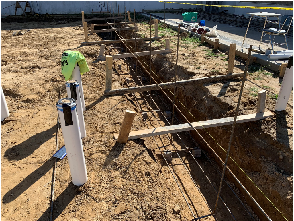
Figure 10 – Footing Trenches
