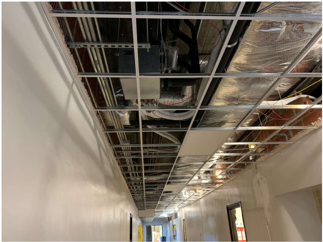
Figure 3 – Grid Install
