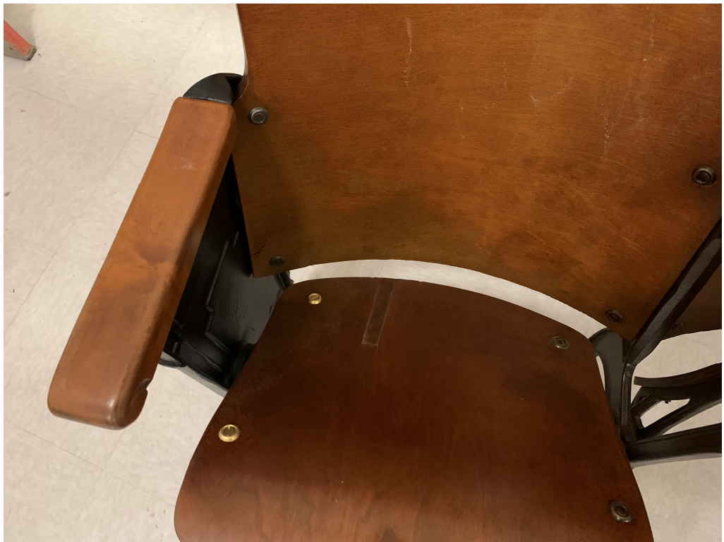
Figure 7 – Brass on New Fasteners Stand Out Brightly (should darken and dull over time)
