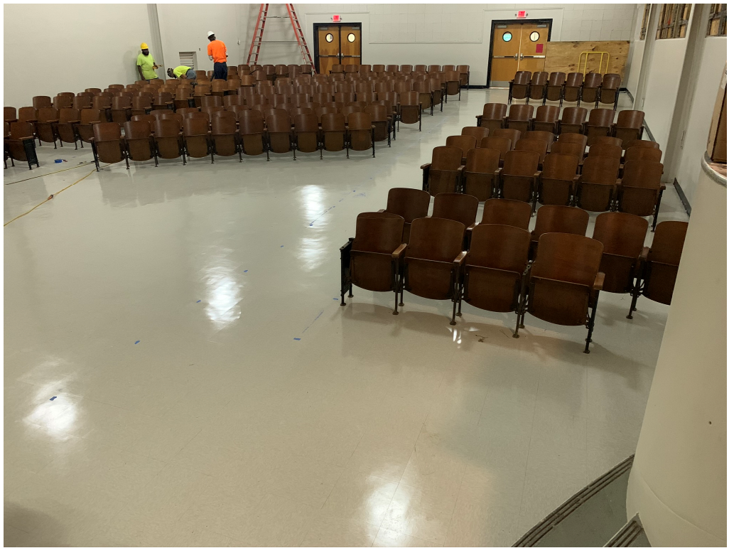
Figure 1 – Auditorium Seating Installation
