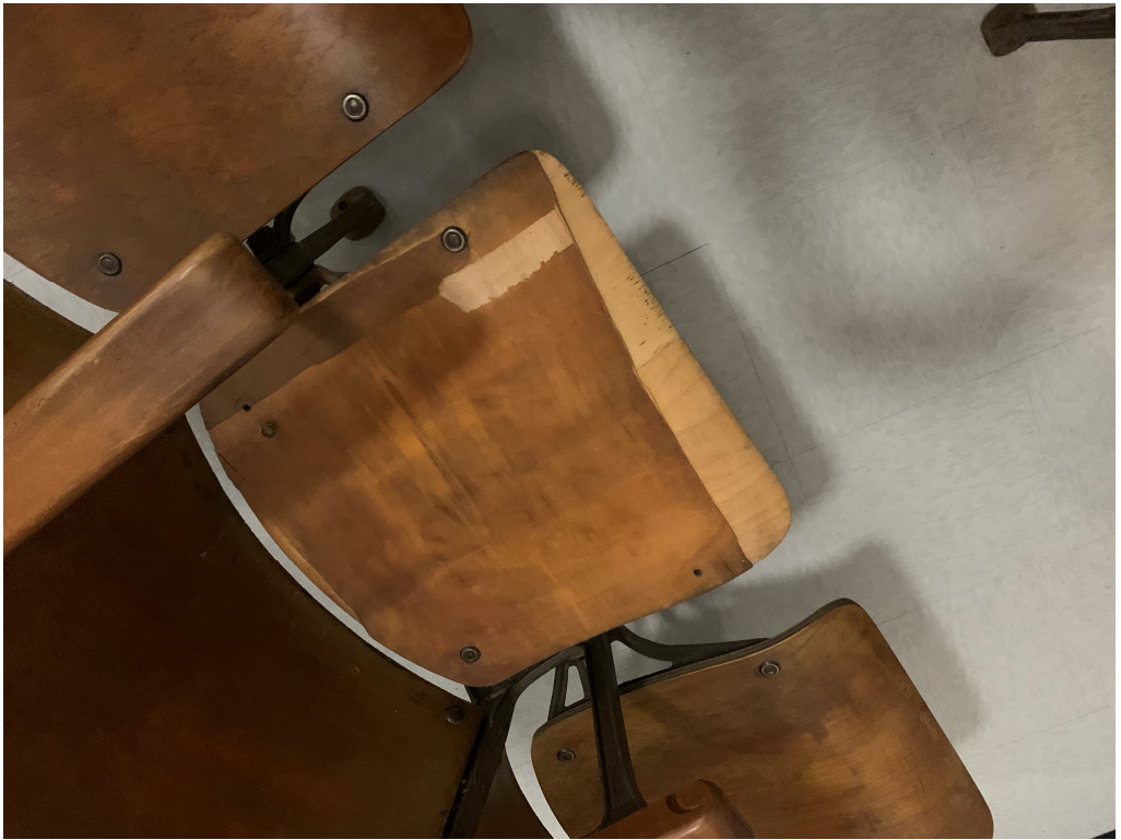
Figure 11 – Unfinished Seat to be replaced with Unused Rows
