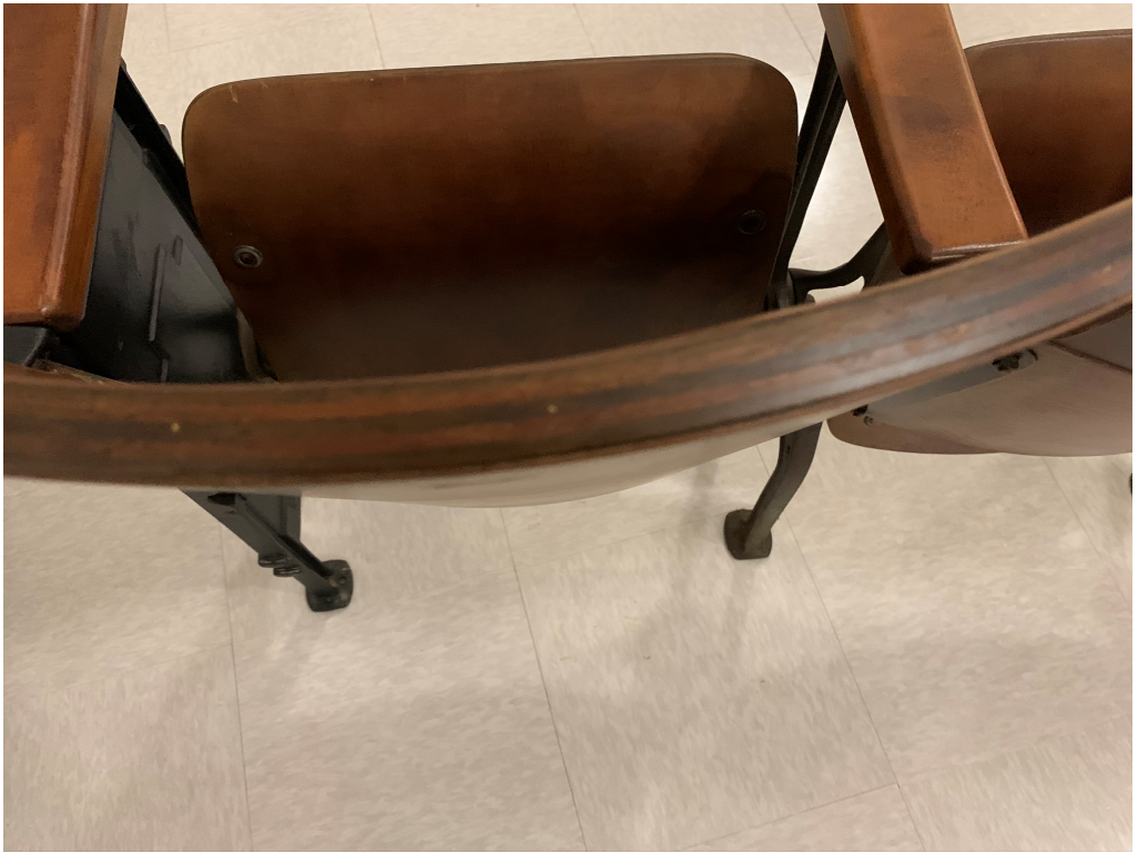
Figure 5 – Some Delamination needs to be Re-Adhered
