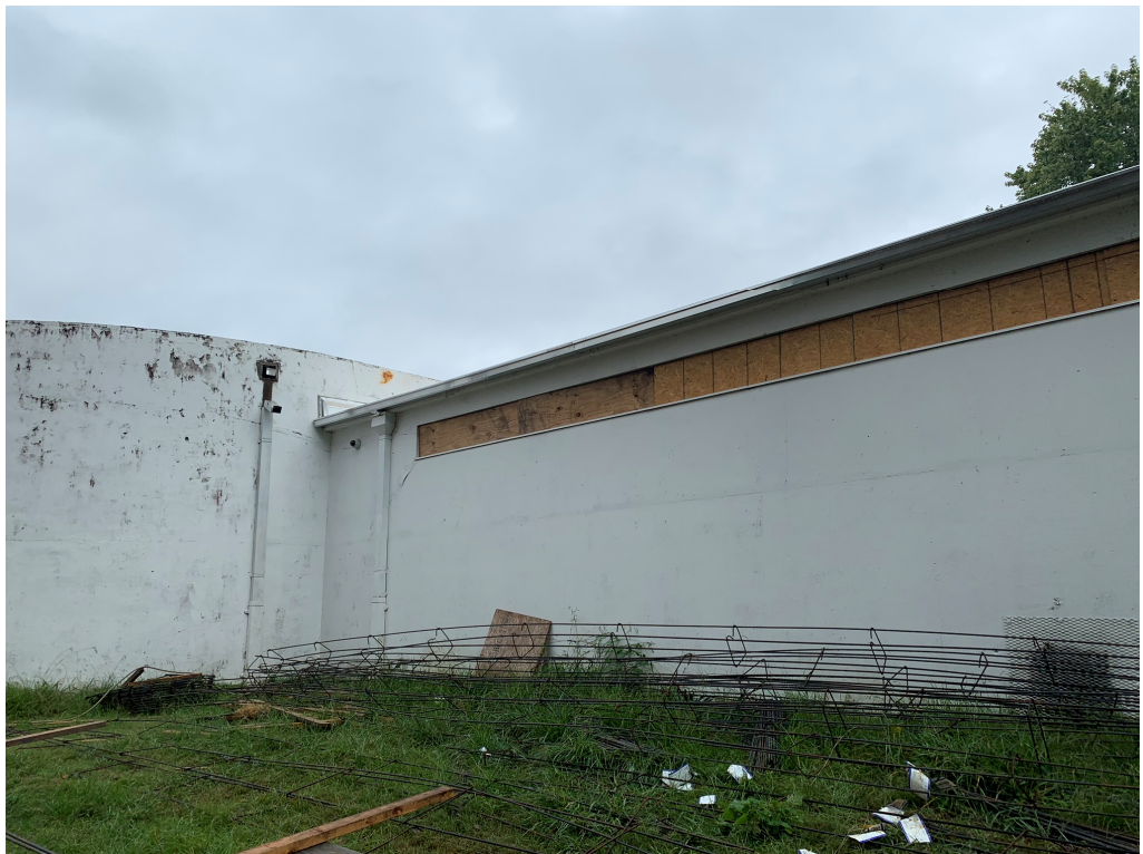
Figure 14 – New Gutter at Roof
