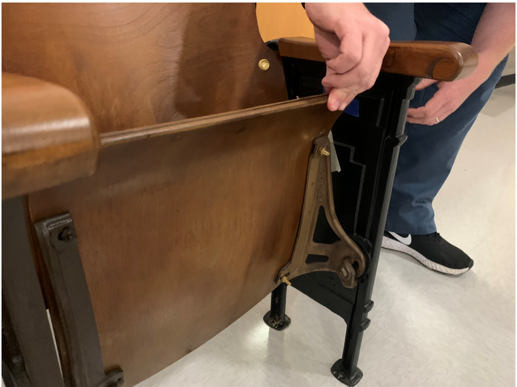
Figure 10 – End Hinge Brackets are Different Color than all others at every row
