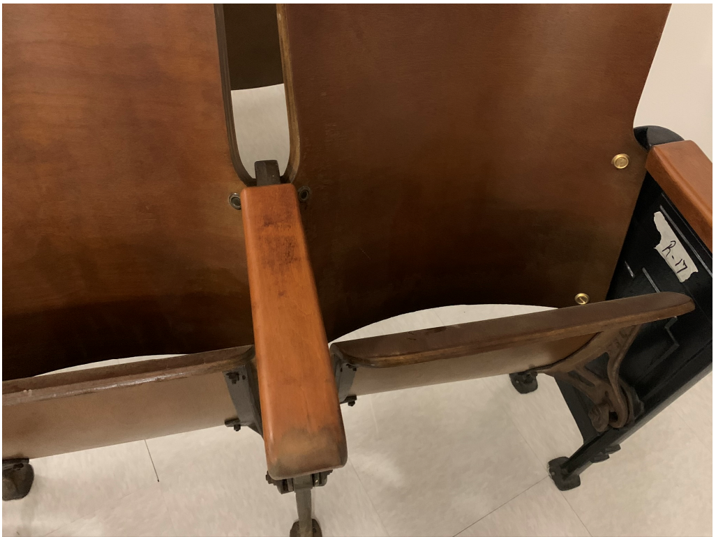
Figure 6 – Brass on New Fasteners Stand Out Brightly (should darken and dull over time)
