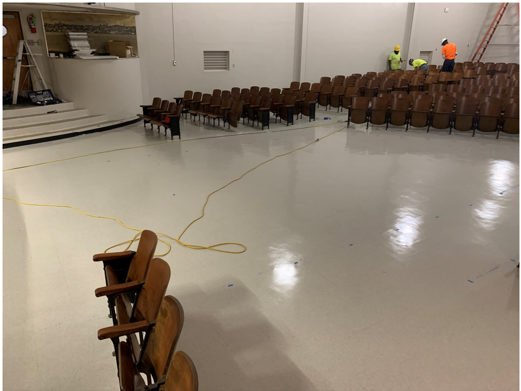
Figure 2 – Auditorium Seating Installation
