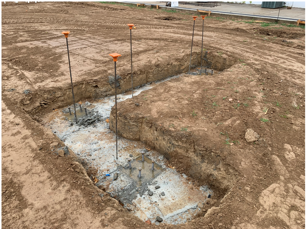
Figure 16 – Footing Concrete Installed
