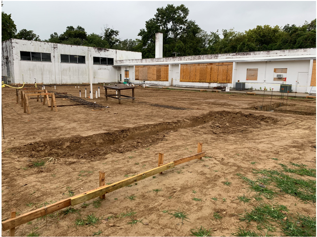
Figure 15 – Building Pad and Slab Layout
