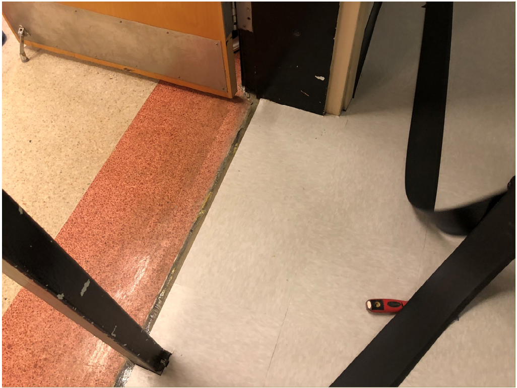
Figure 7 – Base Installing at Auditorium is nearing Completion
