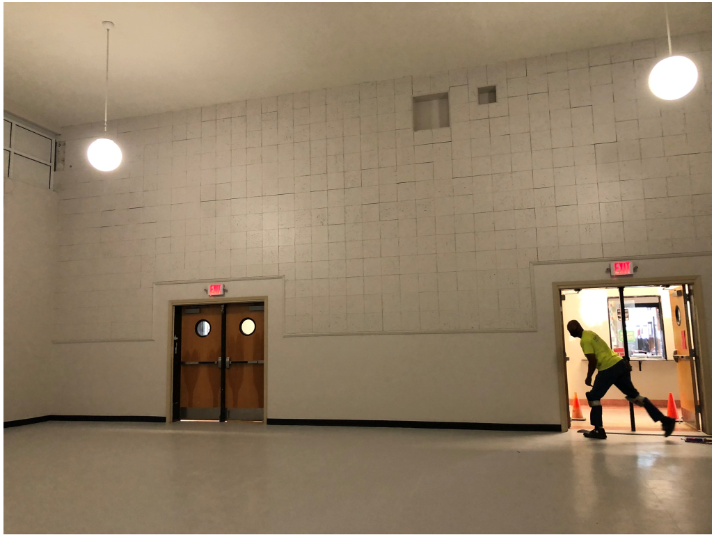
Figure 5 – Auditorium VCT Installed & Walls Painted
