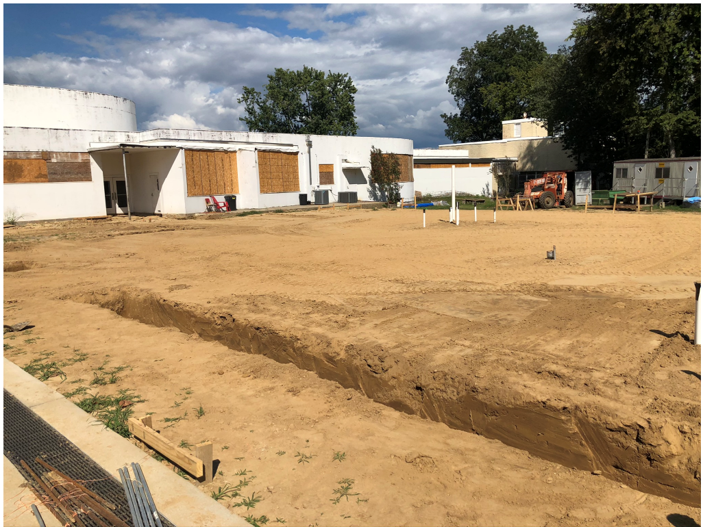
Figure 16 – Rear Addition Building Pad
