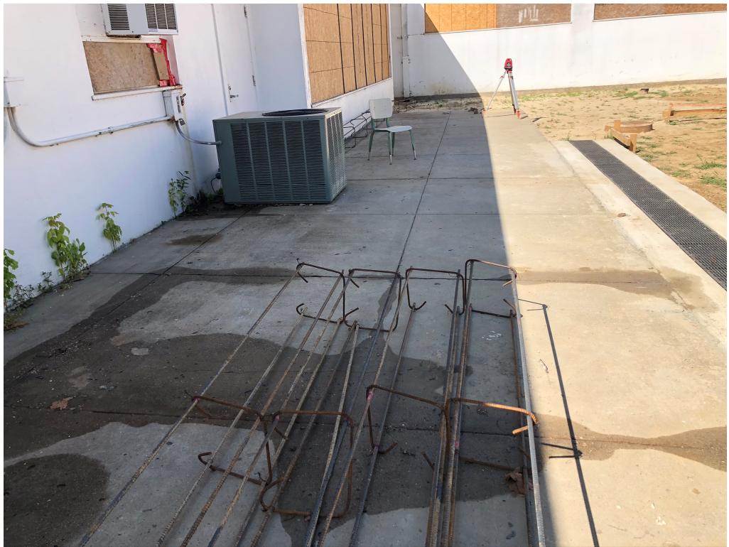
Figure 14 – Rebar Prepped for Installation at Footing Excavations
