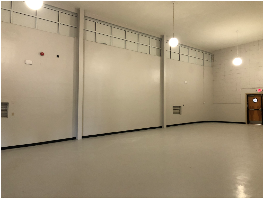
Figure 3 – Auditorium VCT Installed & Walls Painted
