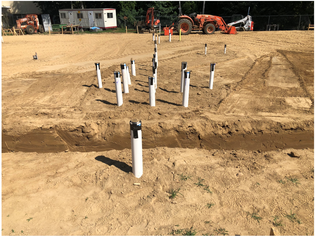
Figure 15 – Below Slab Drainage Prepped for Concrete Install
