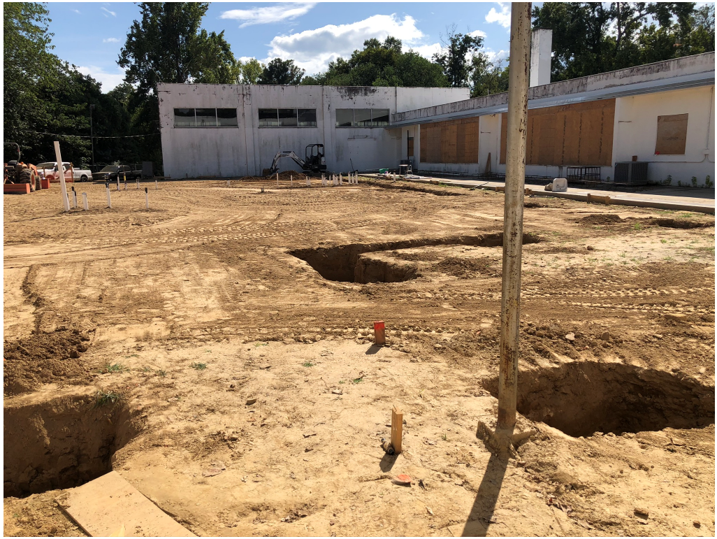
Figure 9 – Footing Excavation at Rear Addition
