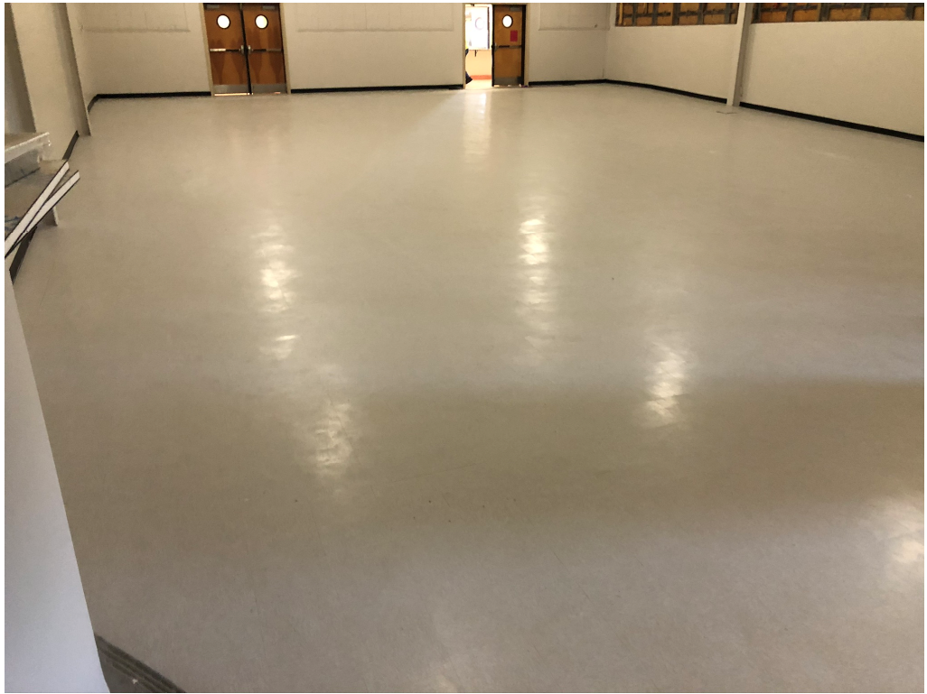
Figure 1 – Auditorium VCT Installed
