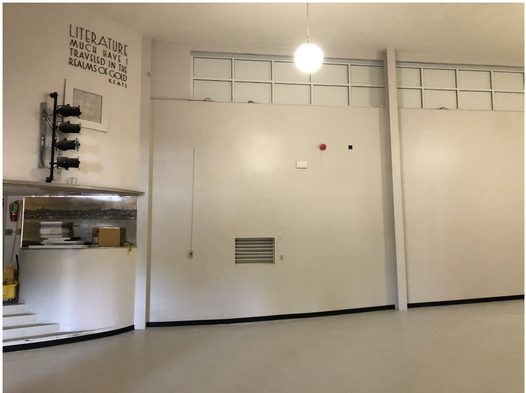
Figure 4 – Auditorium VCT Installed & Walls Painted
