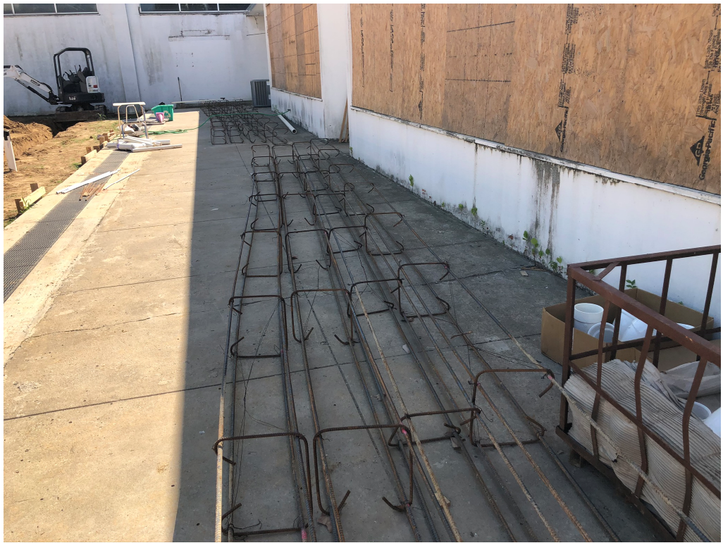
Figure 13 – Rebar Prepped for Installation at Footing Excavations
