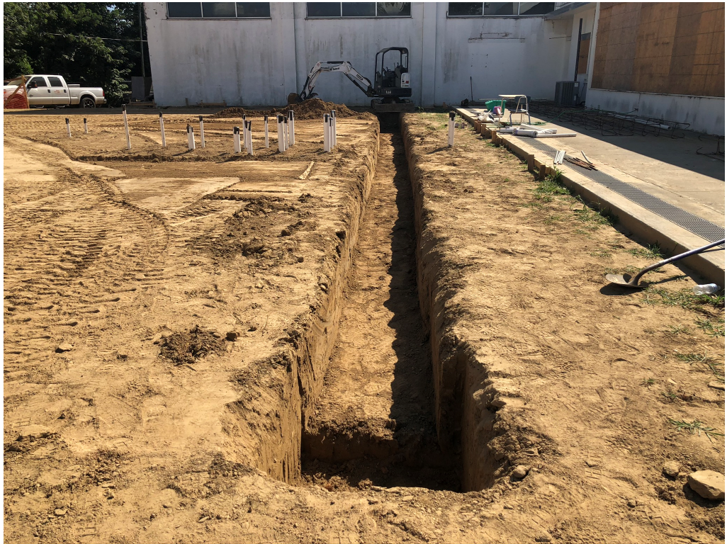
Figure 12 – Footing Excavation at Rear Addition
