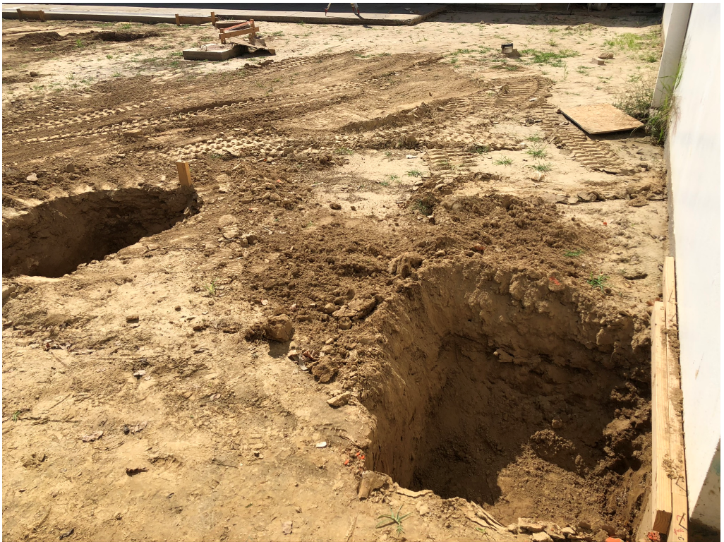
Figure 8 – Footing Excavation at Rear Addition
