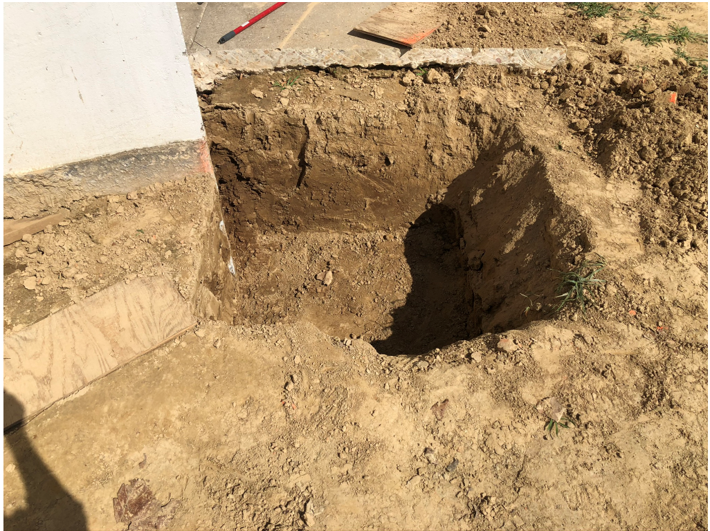
Figure 10 – Footing Excavation at Rear Addition
