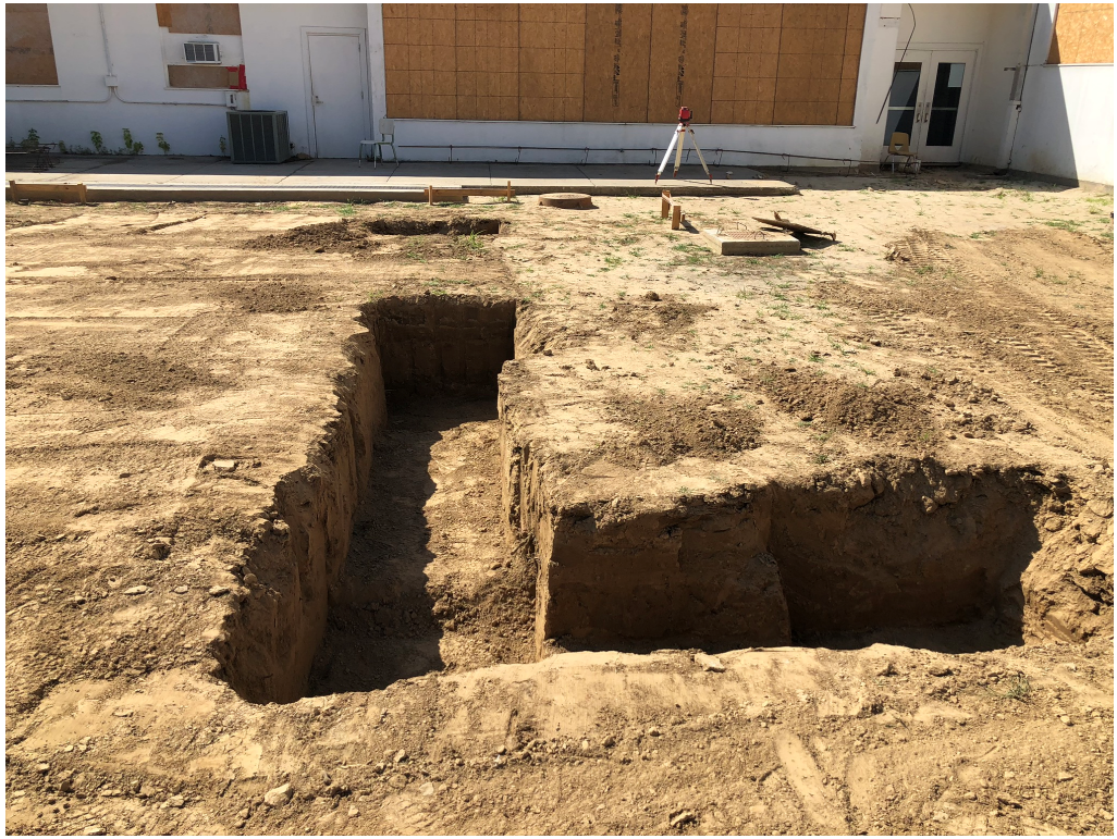
Figure 11 – Footing Excavation at Rear Addition
