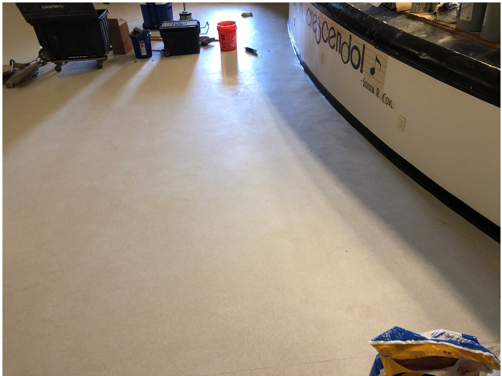
Figure 2 – Auditorium VCT Installed
