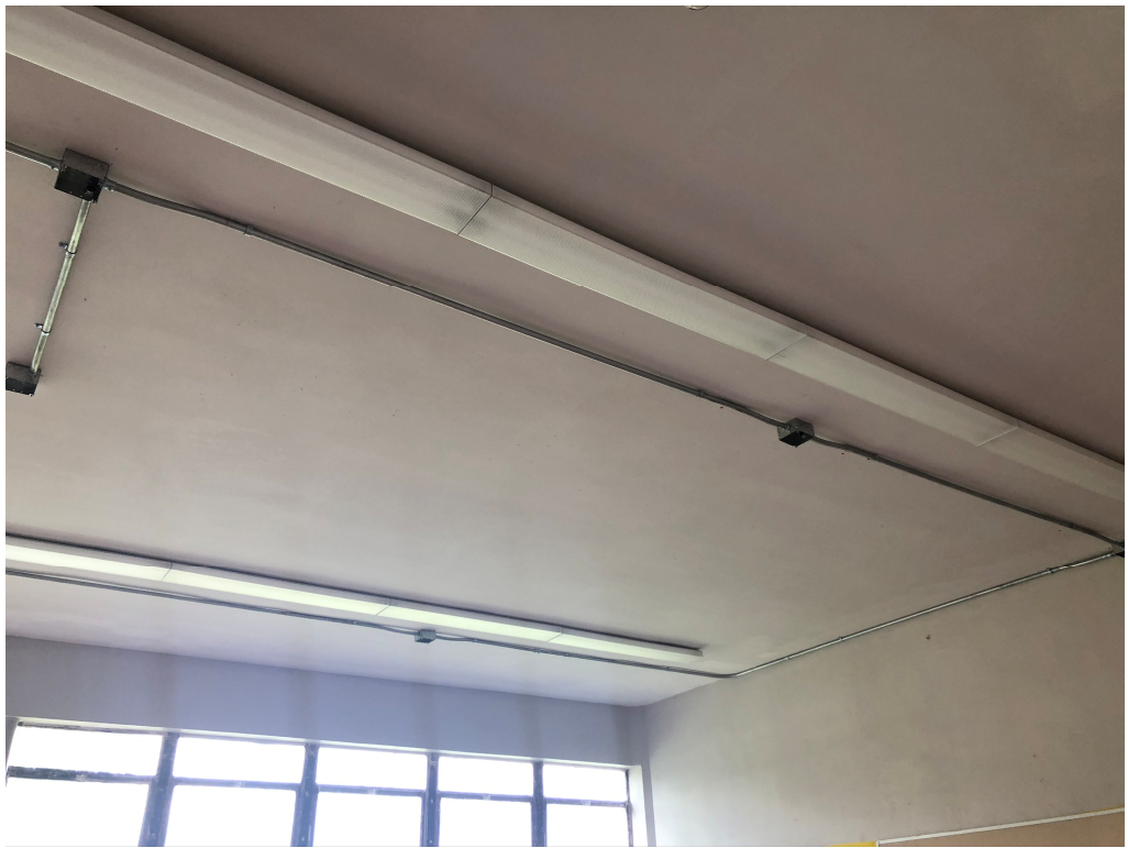
Figure 11 – Conduit Install at Ceiling in Some Rooms
