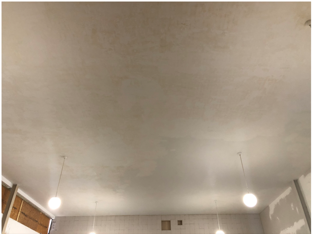
Figure 6 – Ceiling Prep at Auditorium
