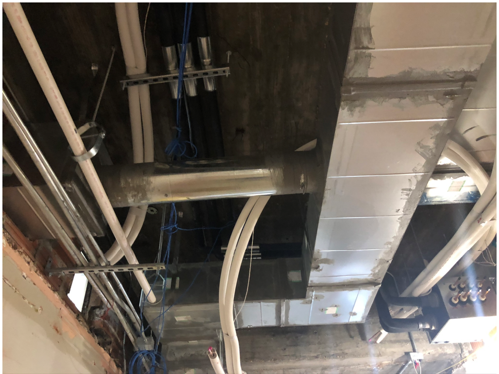
Figure 8 – Sealed Ducting
