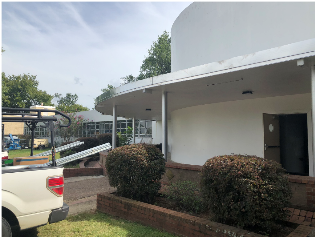
Figure 2 – Roof Edge Installed at Front Covering
