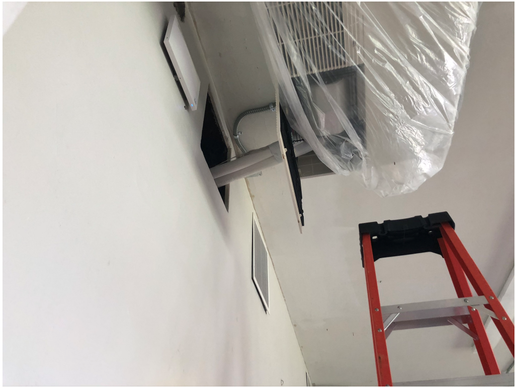
Figure 9 – HVAC Equipment Install Ongoing
