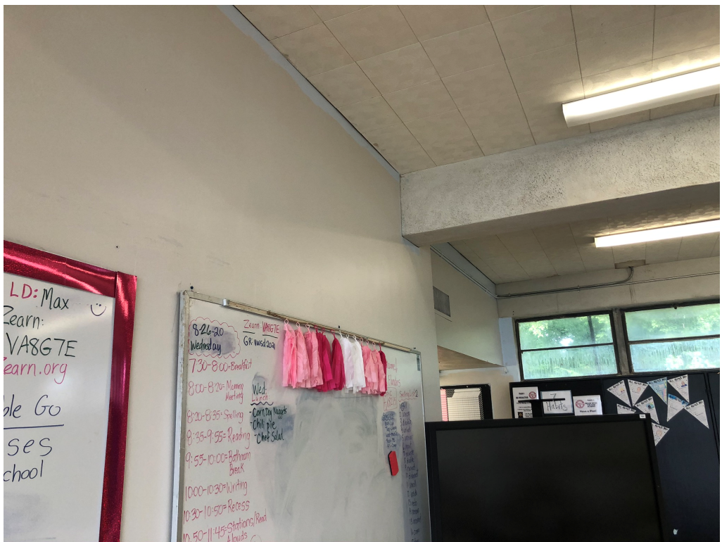
Figure 14 – Field Paint Applied; Awaiting Trim Out
