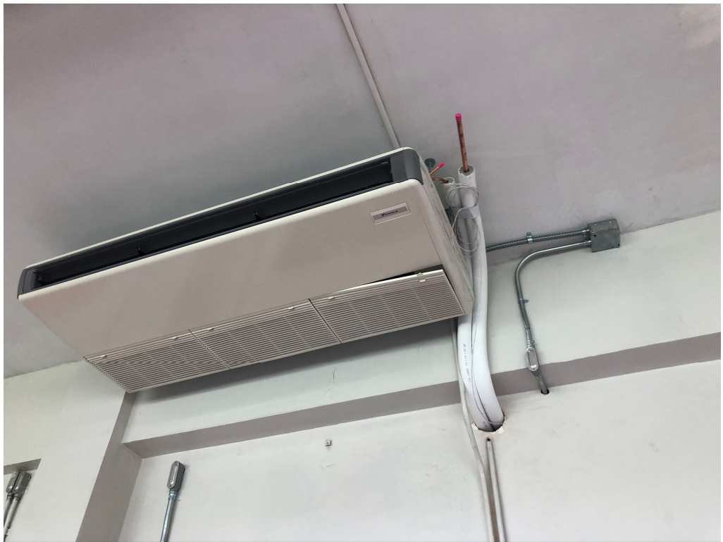
Figure 10 – HVAC Equipment Install Ongoing
