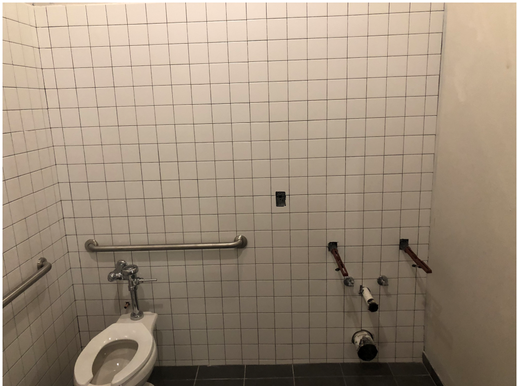
Figure 18 – Fixtures Partially Installed at ADA Bathroom
