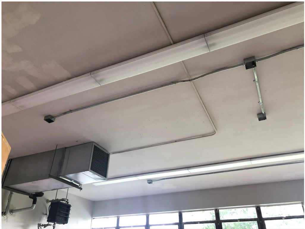
Figure 12 – Conduit Install at Ceiling in Some Rooms
