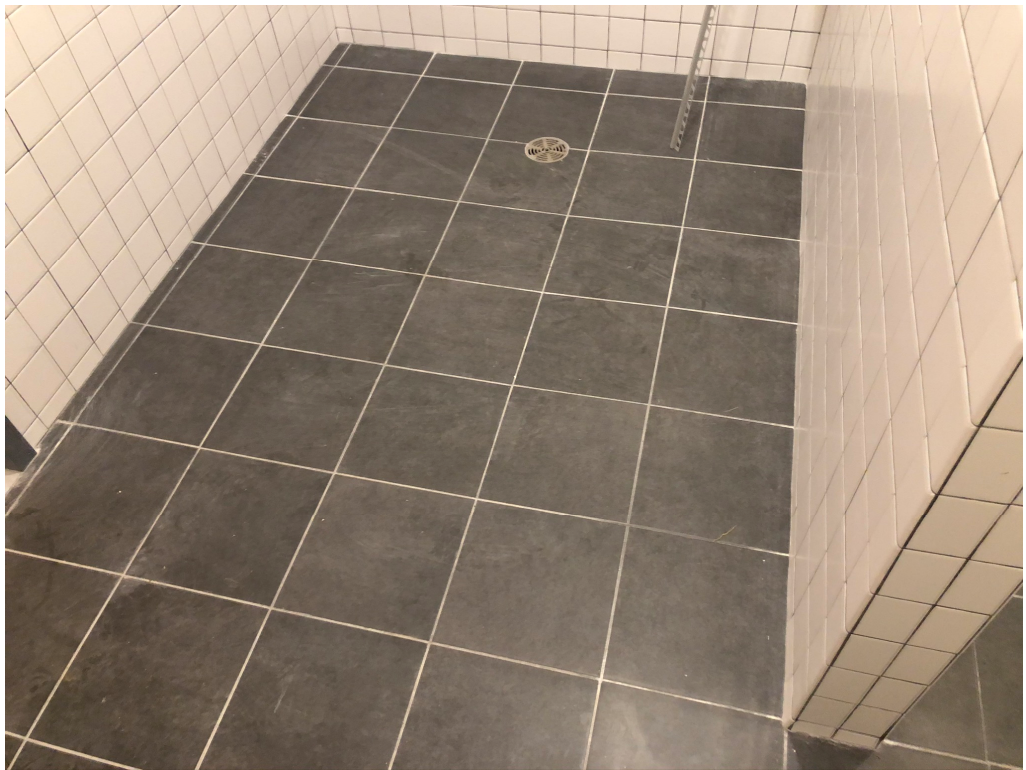
Figure 20 – Tile Grouted at ADA Bathroom
