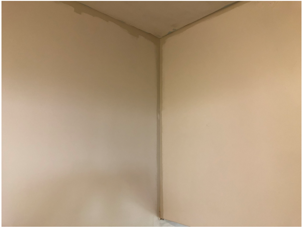
Figure 15 – Field Paint Applied; Awaiting Trim Out
