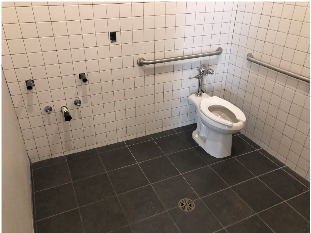
Figure 22 – ADA Bathroom Fixtures Partially Installed
