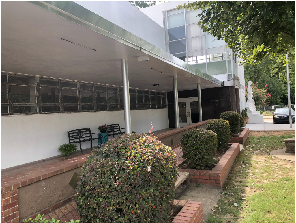
Figure 3 – Roof Edge Installed at Front Covering
