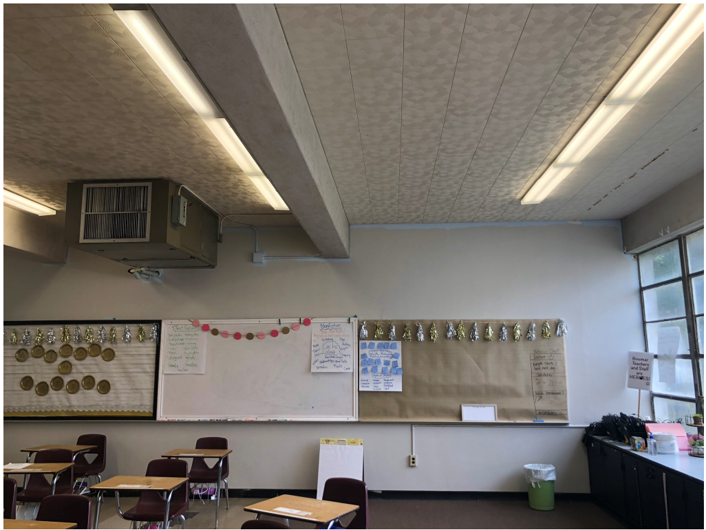
Figure 13 – Field Paint Applied; Awaiting Trim Out
