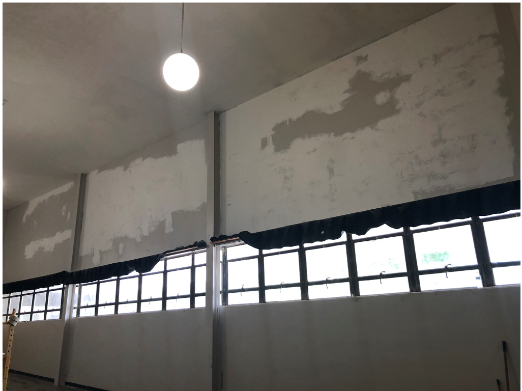
Figure 4 – Wall Prep at Auditorium
