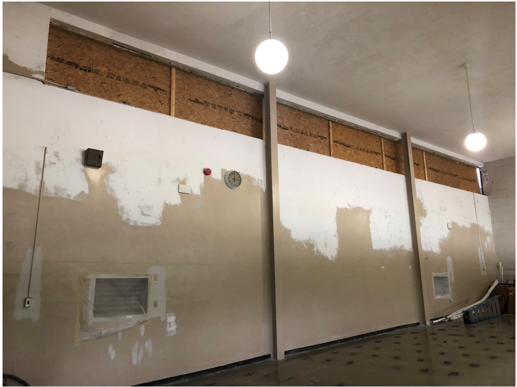
Figure 5 – Wall Prep at Auditorium
