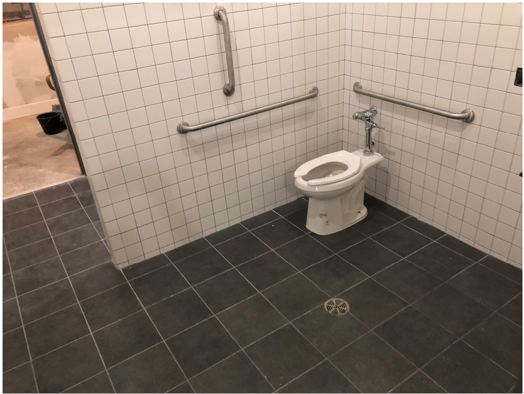
Figure 19 – Fixtures Partially Installed at ADA Bathroom
