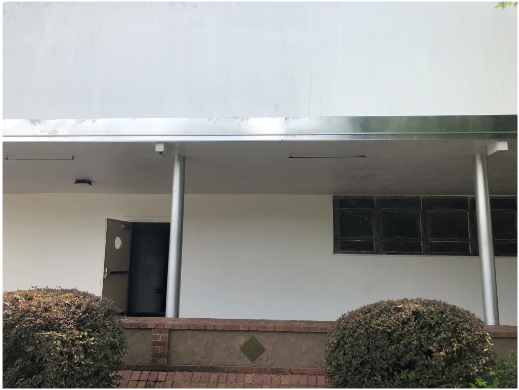
Figure 1 – Roof Edge Installed at Front Covering
