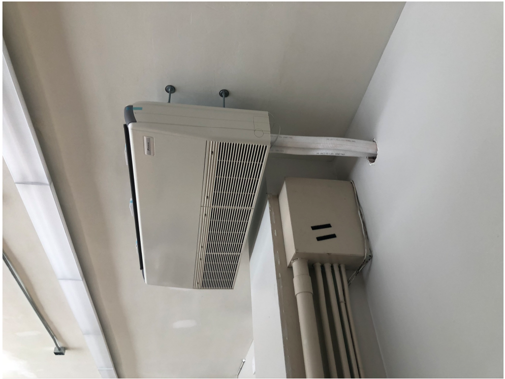
Figure 23 – HVAC Equipment Install Complete in Some Rooms
