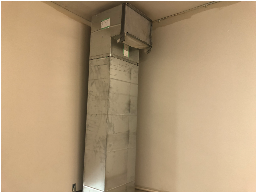
Figure 16 – HVAC Ducting Partially Installed
