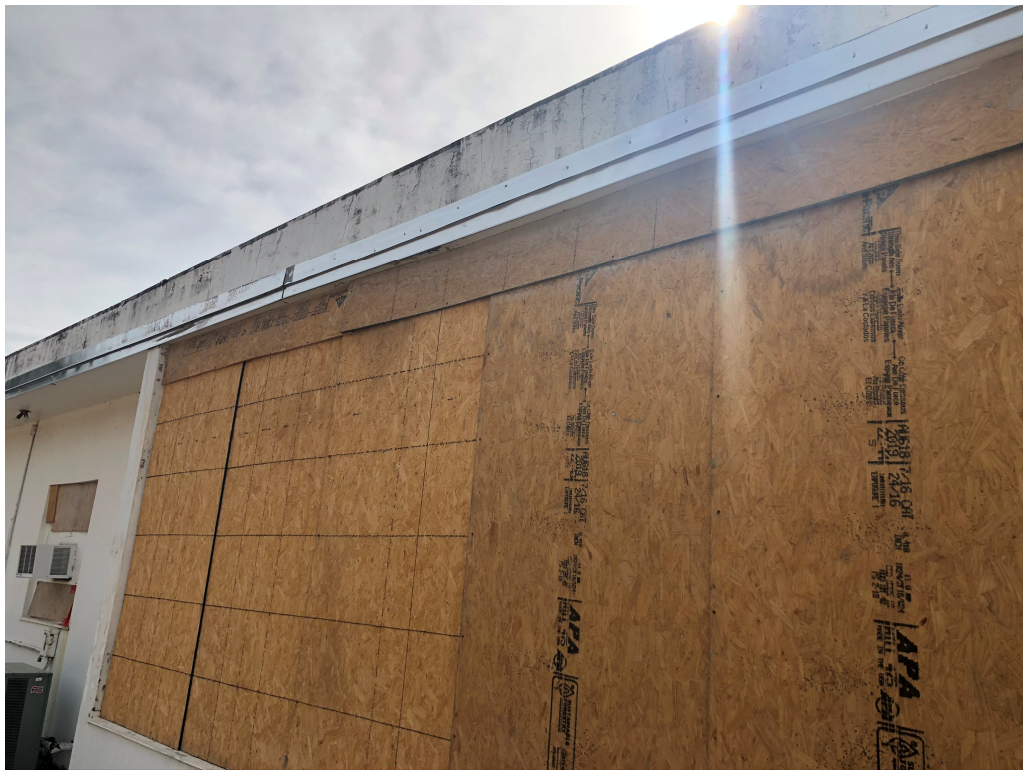
Figure 24 – Base Trim Installed Awaiting Cover Trim
