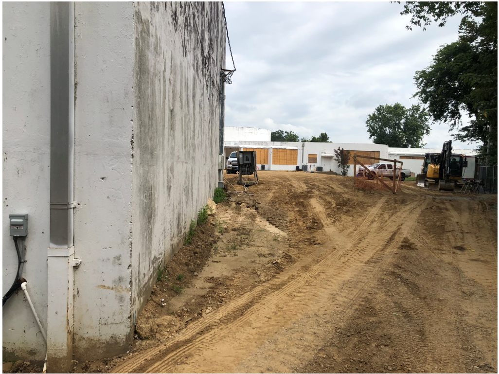
Figure 1 – Dirt Pad up to grade
