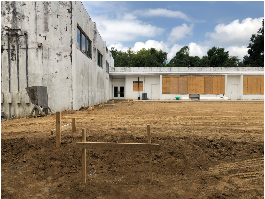
Figure 2 – Batter Boards set and Foundation layout in progress
