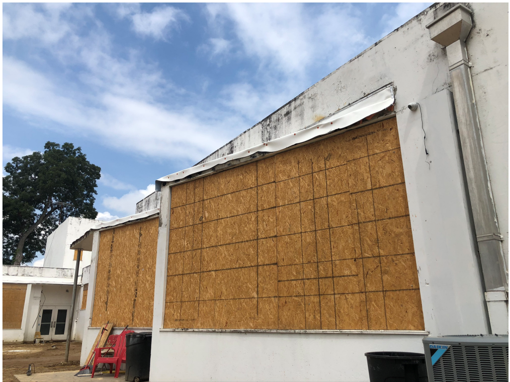
Figure 4 – Roof Material Brought Down Over Edge (typical)
