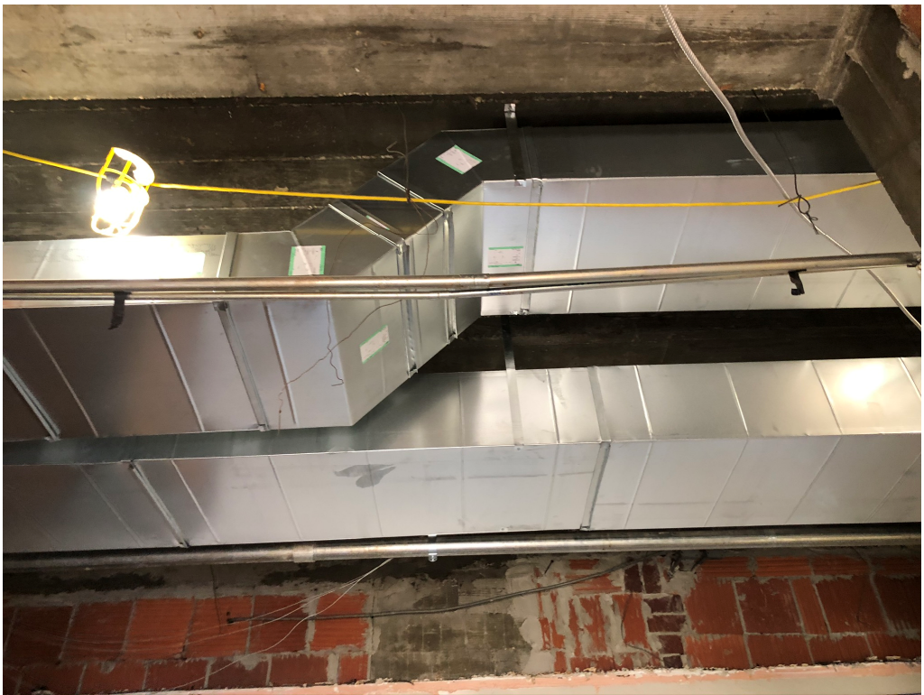
Figure 6 – New Ducting in Passage 116
