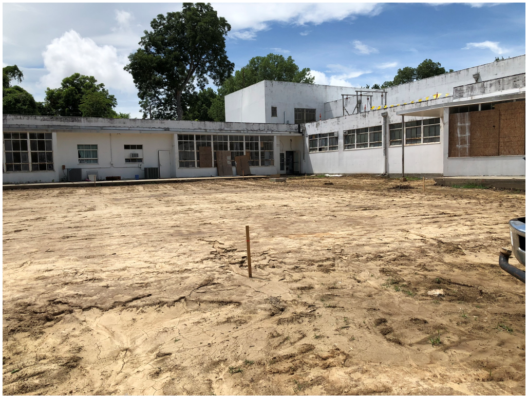
Figure 7 – Pad in Rear Yard
