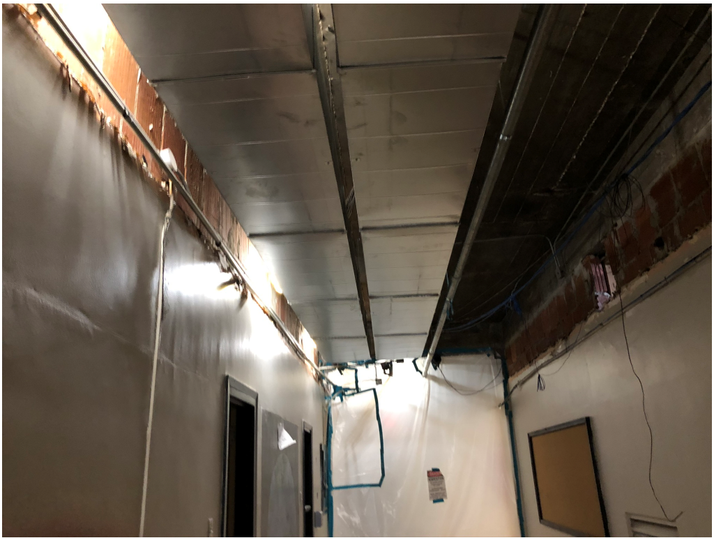
Figure 5 – New Ducting in Passage 116
