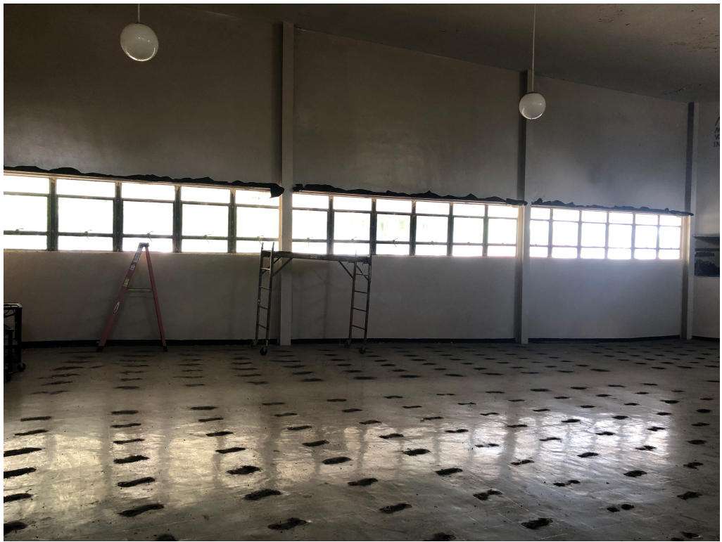
Figure 3 – Window Rehabilitation in Auditorium
