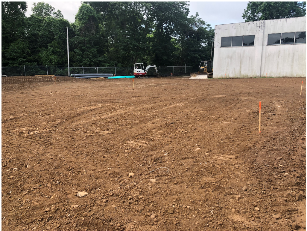
Figure 6 – Grading Stakes Set
