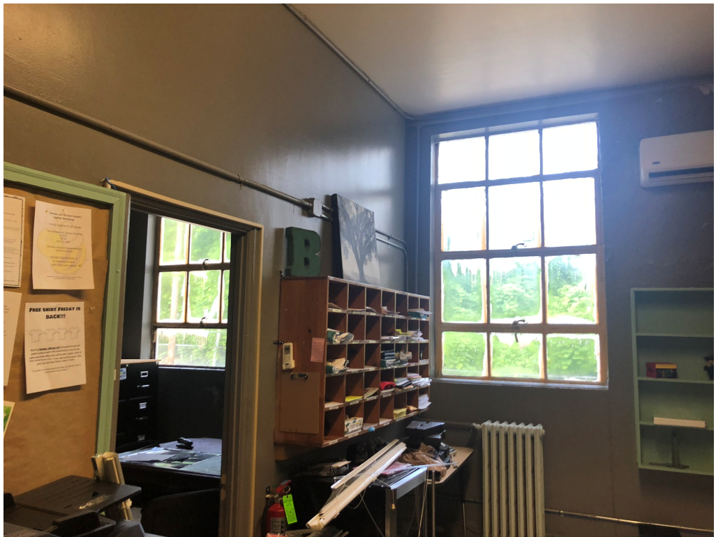
Figure 8 – Chemical Stripper Used to Remove Paint
