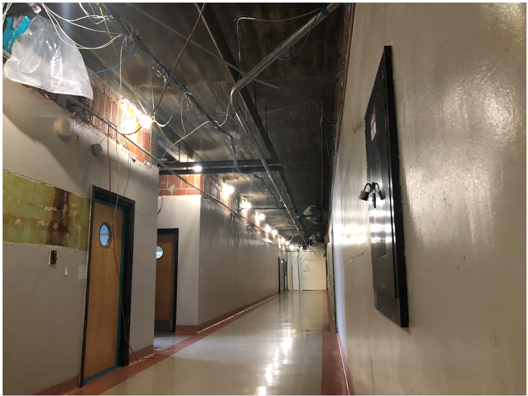
Figure 3 – Asbestos Insulation Removal @ Pipe
