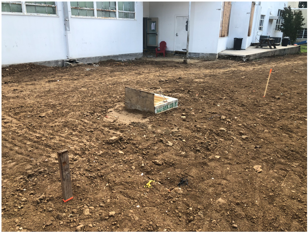
Figure 5 – Inlet Installed with Storm Drainage
