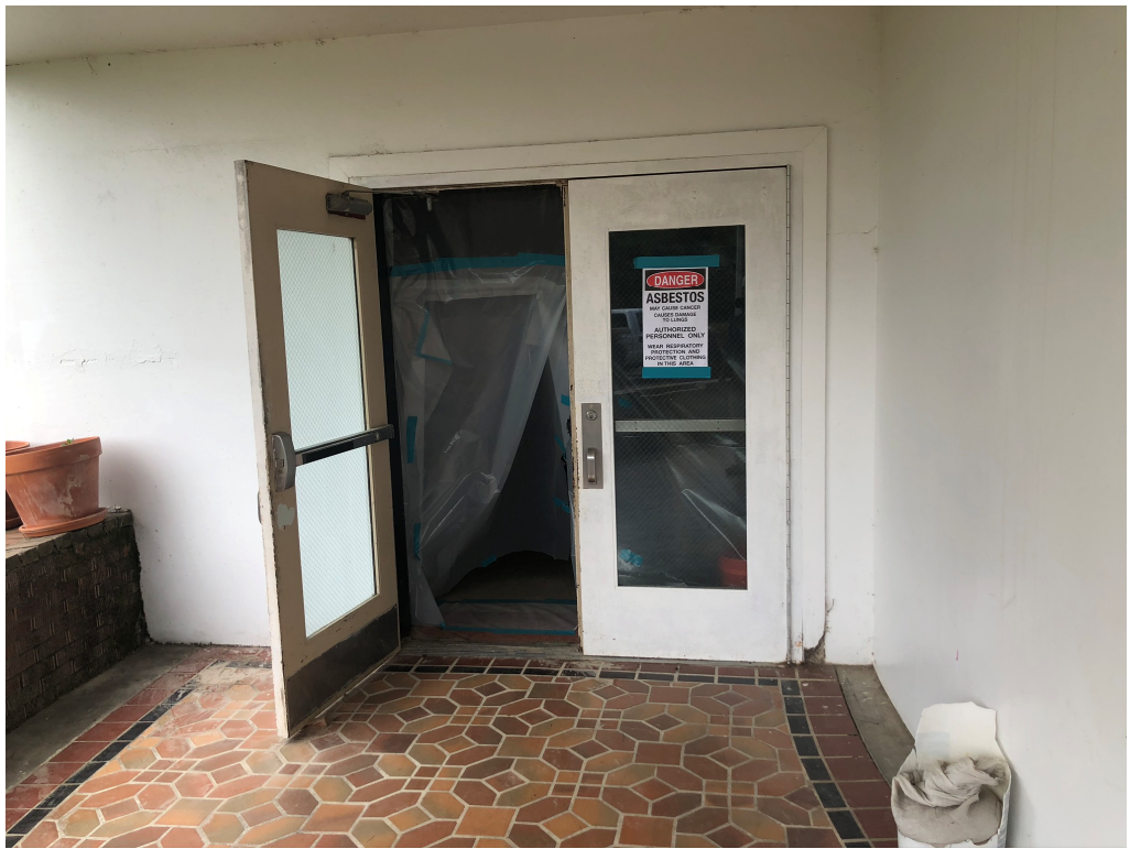
Figure 1 – Asbestos Protection Installed with Signage
