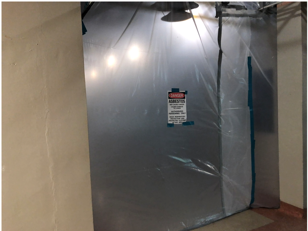
Figure 4 – Asbestos Protection between Halls
