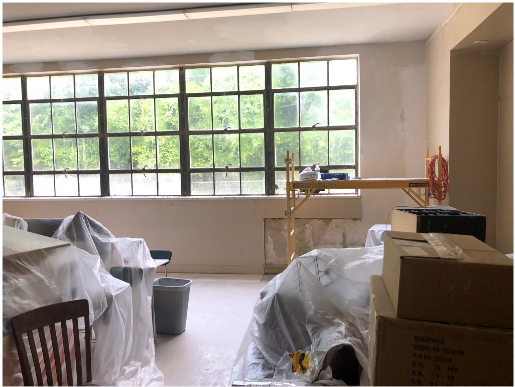
Figure 9 – Paint and Prep Ongoing
