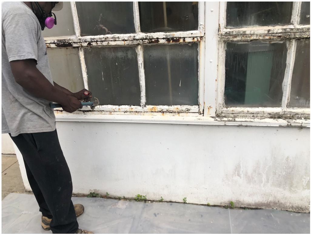
Figure 7 – Window Glazing Removal
