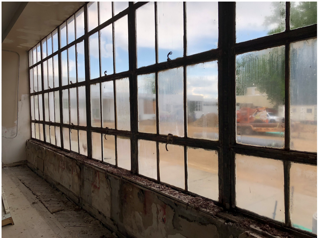
Figure 4 – Chemical Stripper Used to Remove Paint
