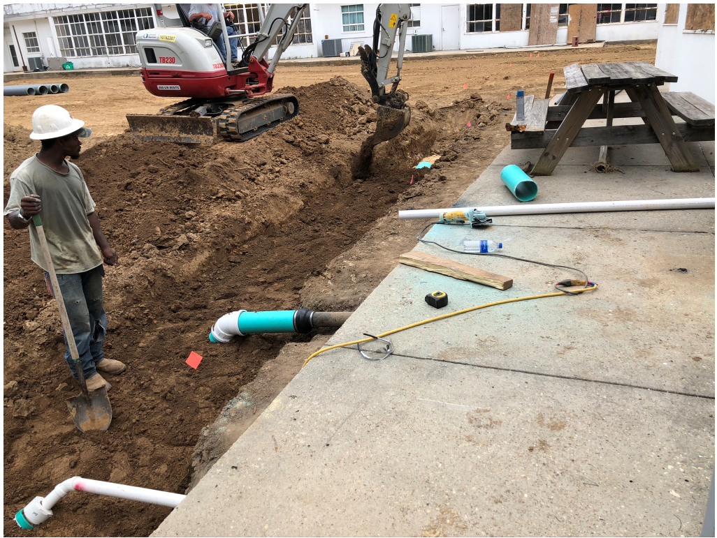
Figure 1 – Rough In Plumbing
