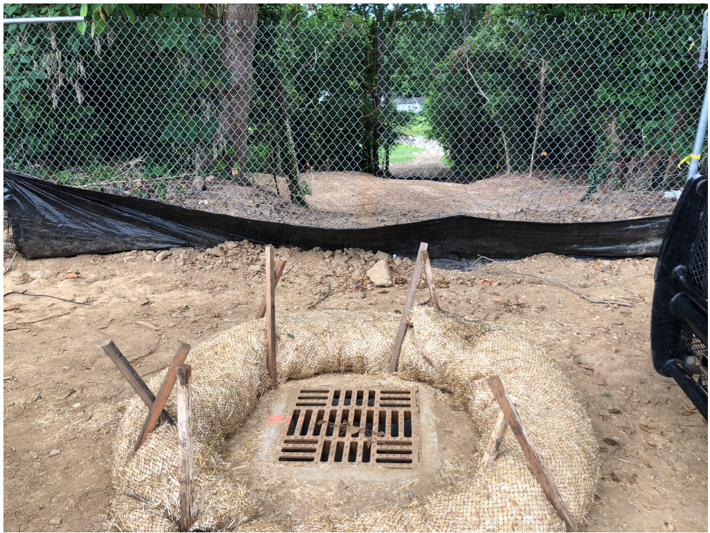
Figure 3 – Grate Surrounded by Sediment Protection
