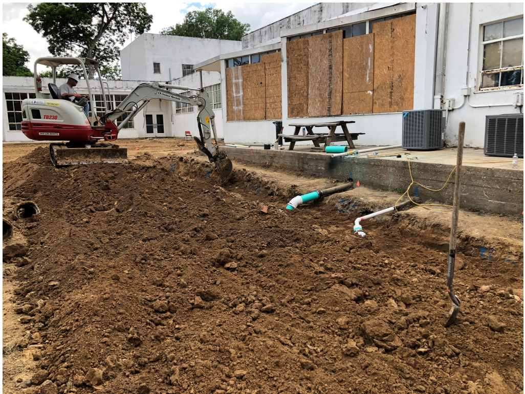
Figure 2 – Rough In Plumbing
