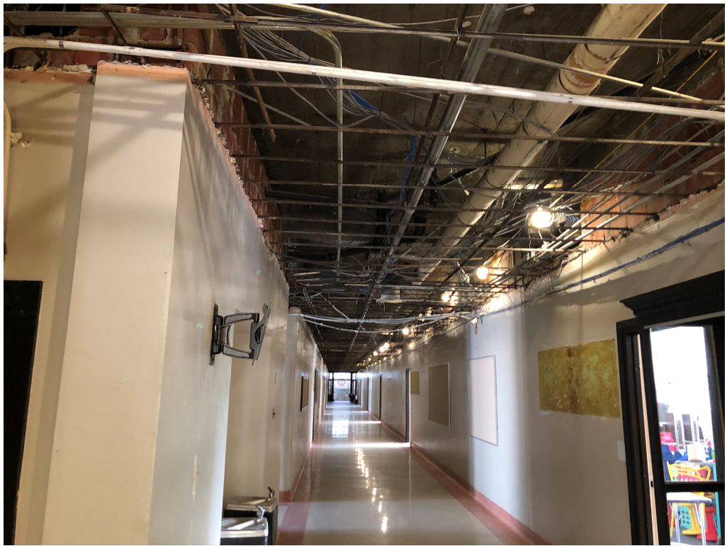
Figure 3 – West Hall Progress
