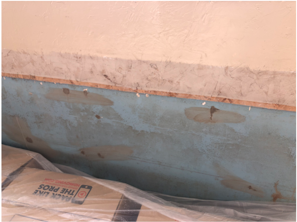
Figure 7 – OSB/Plywood Atop Plaster as Existing Repair to Plaster Sills (typical)
