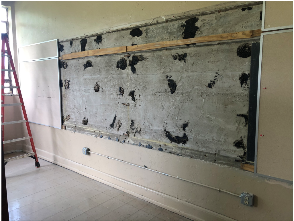
Figure 5 – Science Room 17 Blackboard Removal
