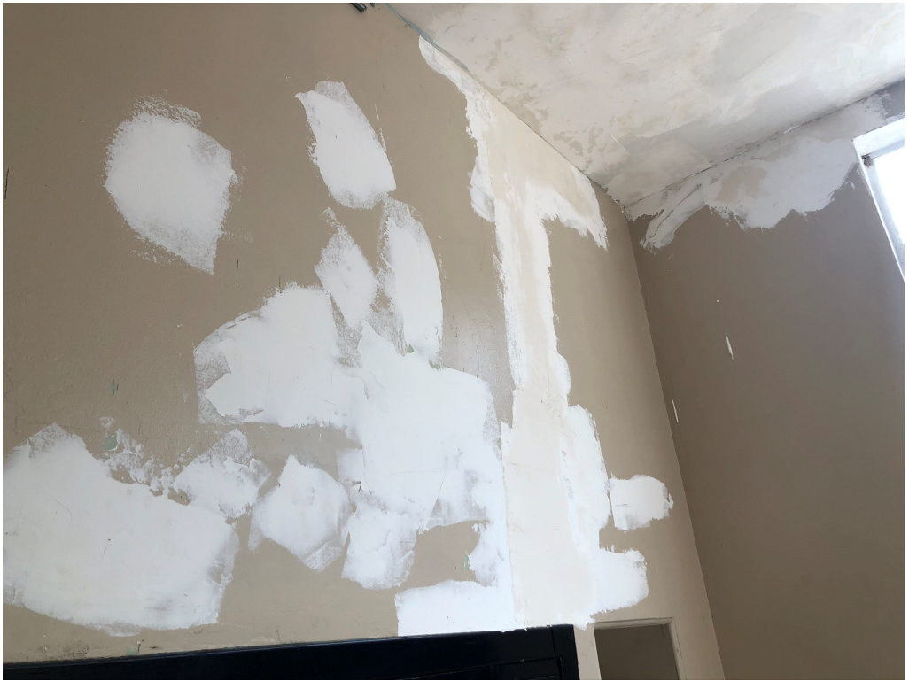
Figure 11 – Plaster Repair at Classroom 3
