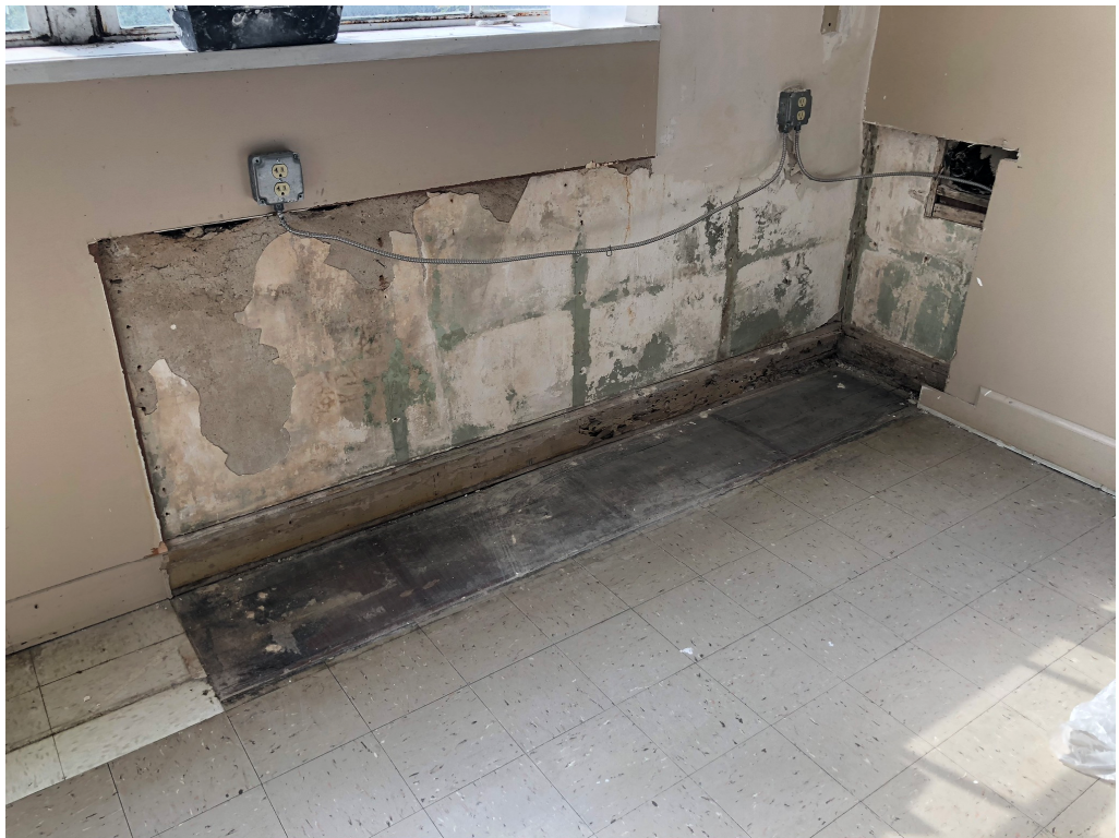
Figure 8 – Classroom 1 Cubby Removal
