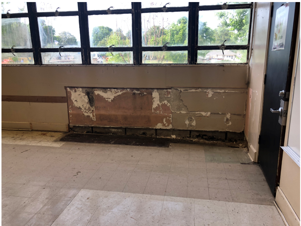
Figure 4 – Science Room 16 Cubby Removal
