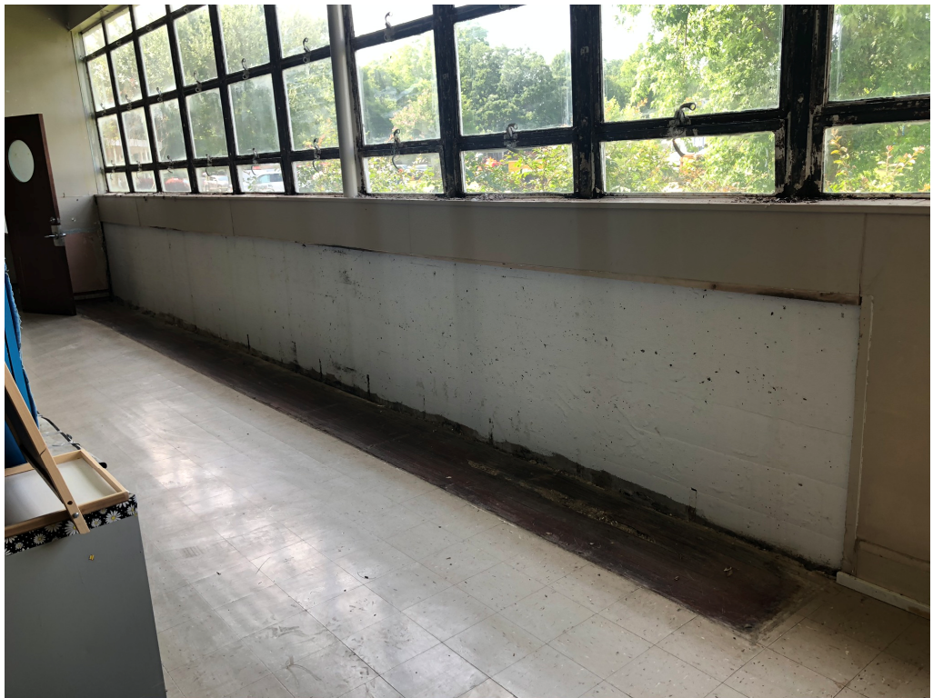
Figure 6 – Science Room 17 Cubby Removal
