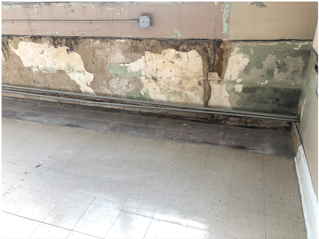
Figure 10 – Classroom 6 Cubby Removal
