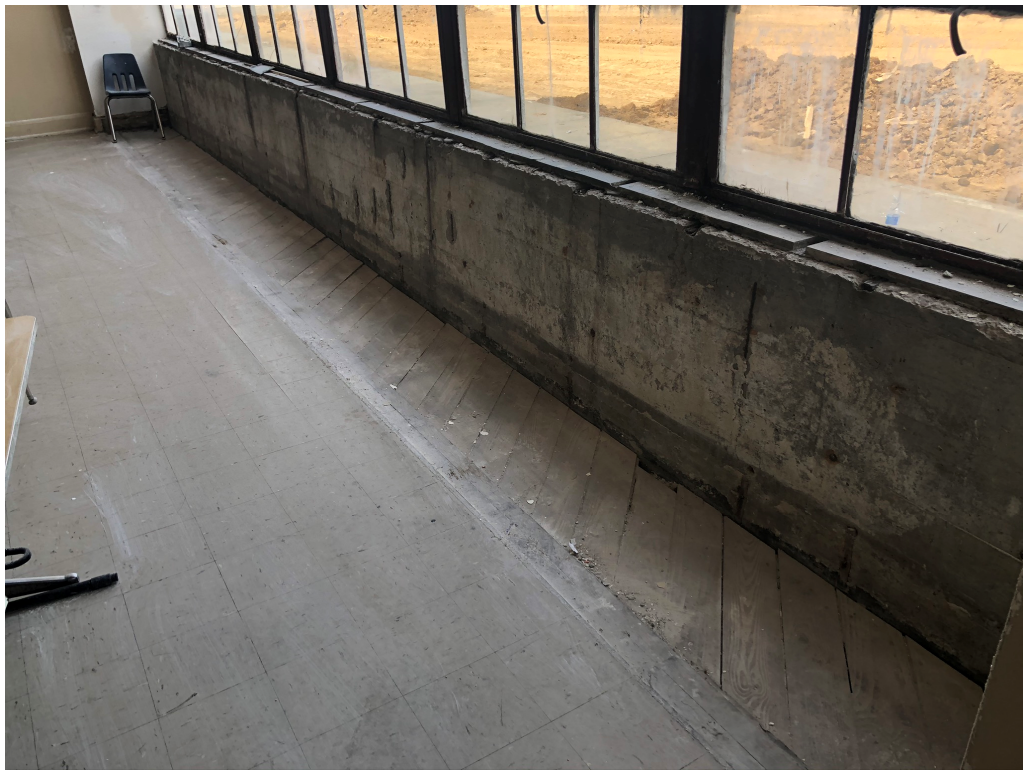
Figure 9 – Sped 2 Cubby Removal
