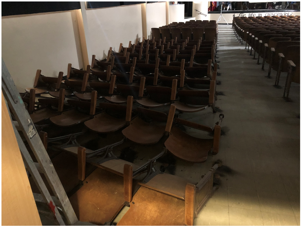
Figure 1 – Chairs in Auditorium have been unfastened at floor
