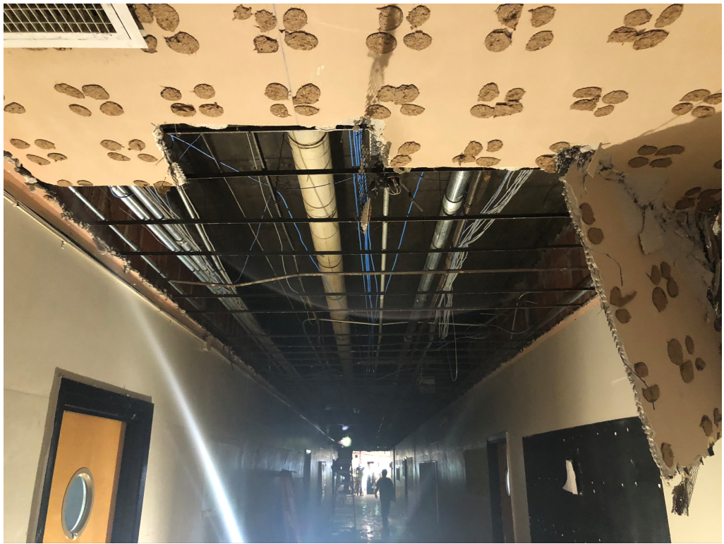
Figure 11 – Corridor 100 Demo Ongoing
