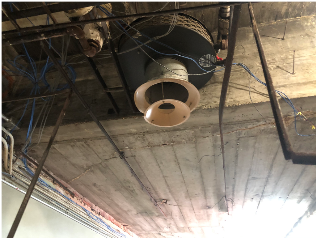
Figure 6 – Step down at Roof
