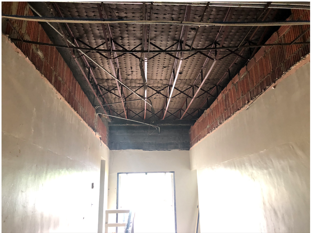
Figure 4 – Demo work at Hallway
