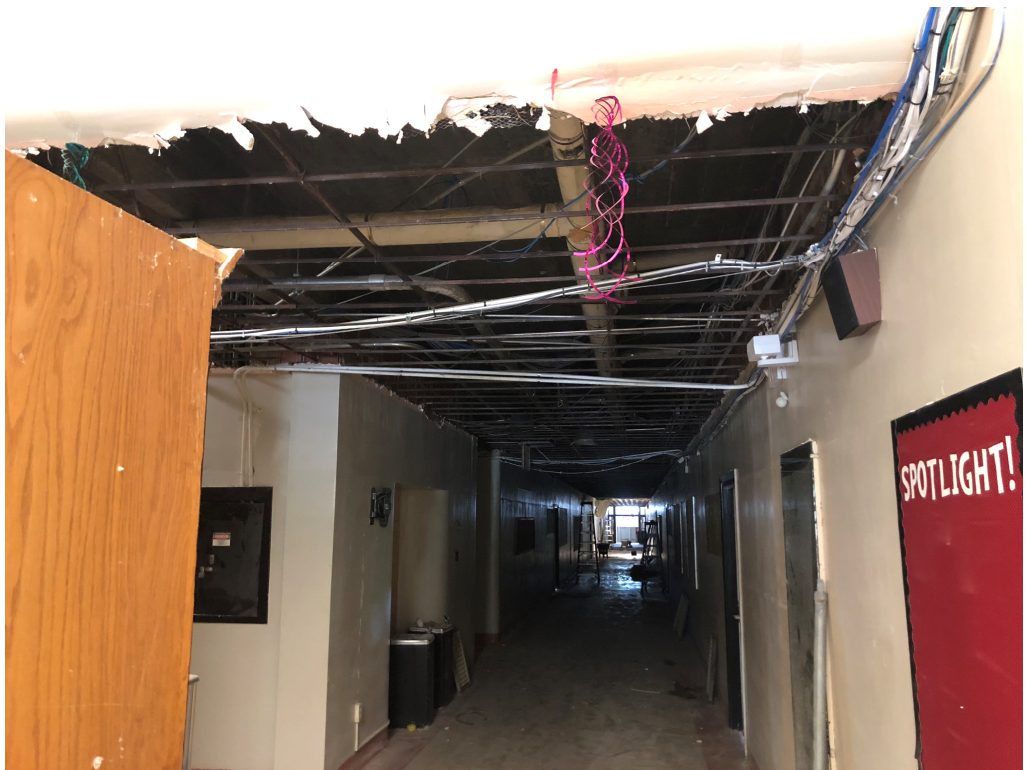
Figure 2 – Demo work at Hallway
