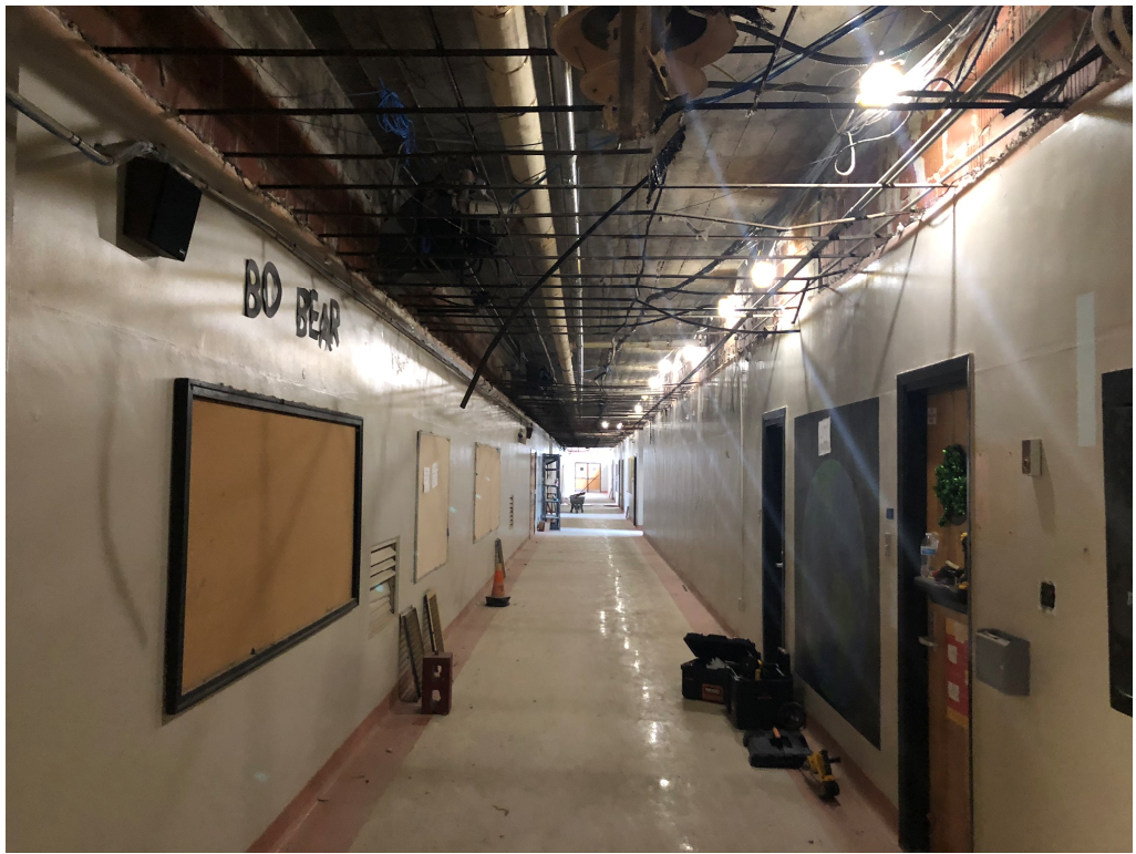
Figure 3 – Demo work at Hallway
