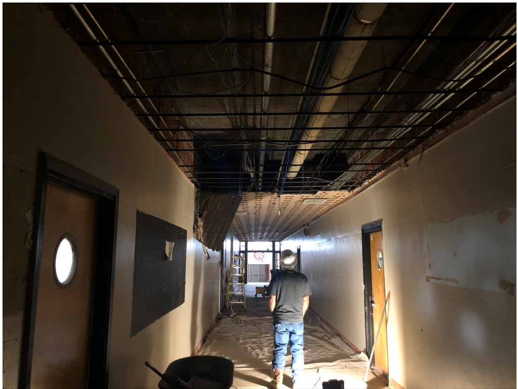
Figure 12 – Corridor 100 Demo Ongoing
