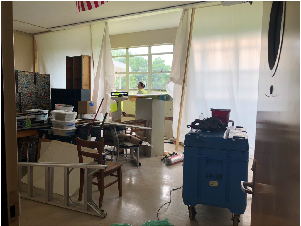
Figure 5 – Classroom 15 plastic protection & window refinishing
