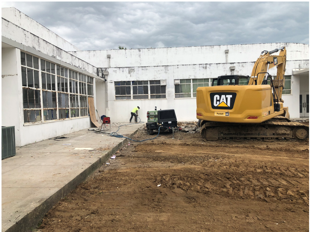
Figure 10 – Concrete Demo Ongoing
