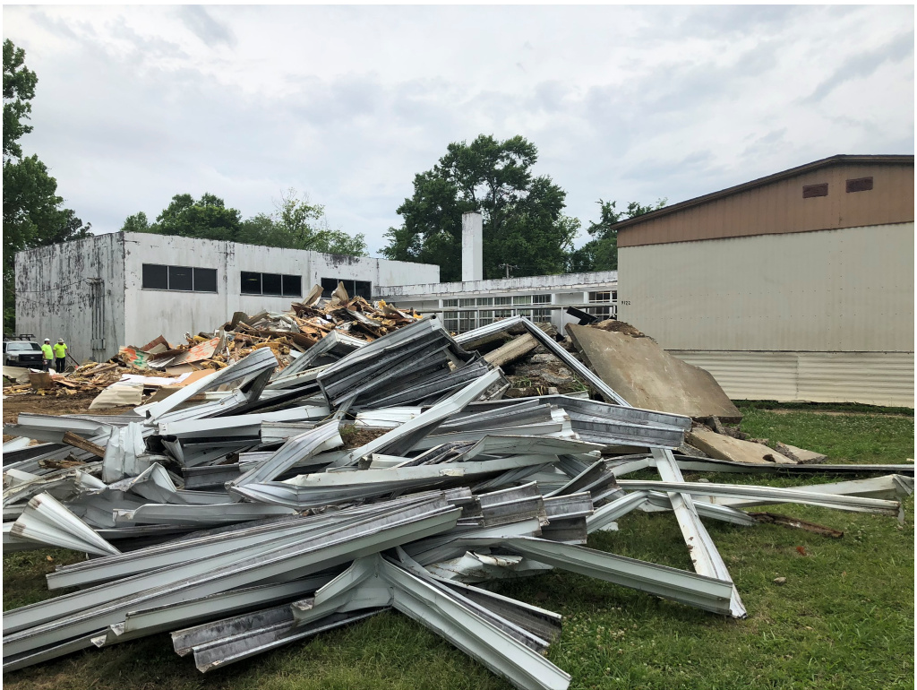
Figure 2 – Demo Work at Trailers
