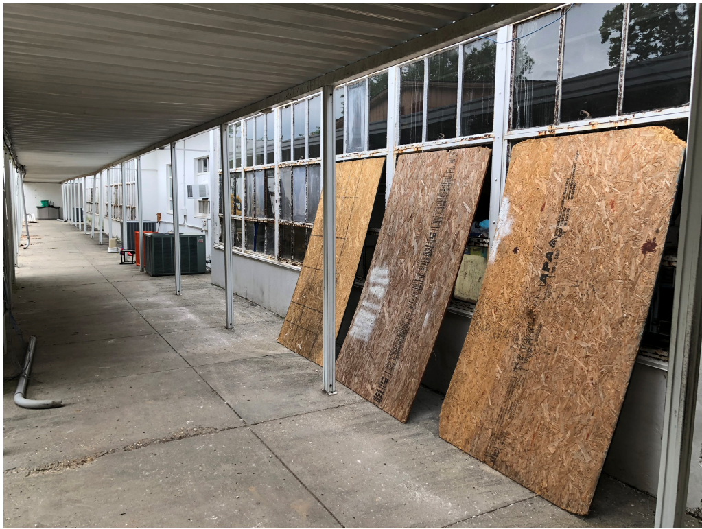
Figure 5 – Some Protection in place for windows
