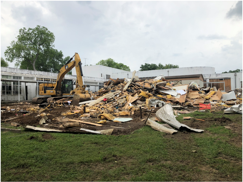
Figure 1 – Demo Work at Trailers
