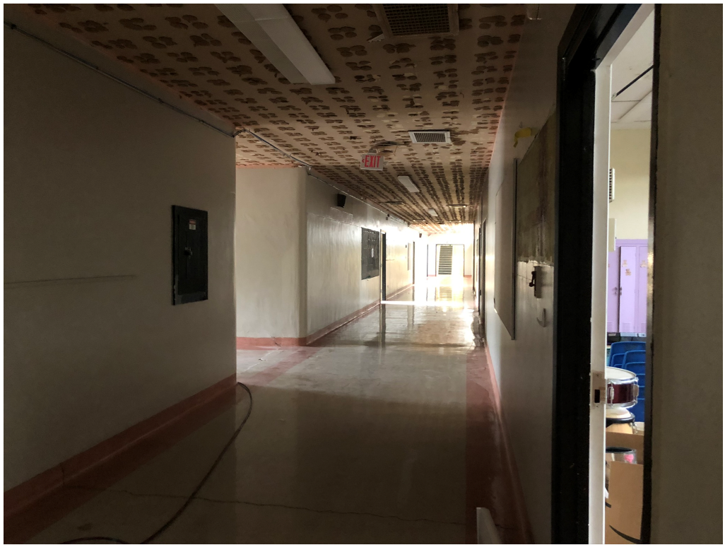
Figure 3 – Ceiling Tile Removed
