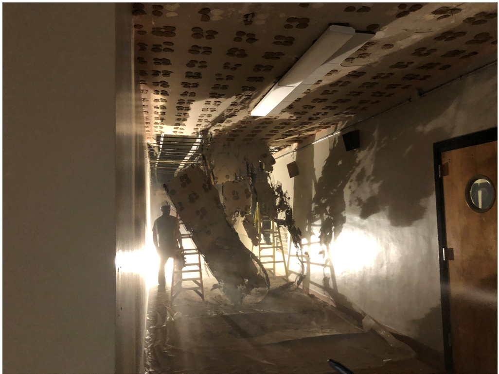
Figure 4 – Ceiling Demo has commenced
