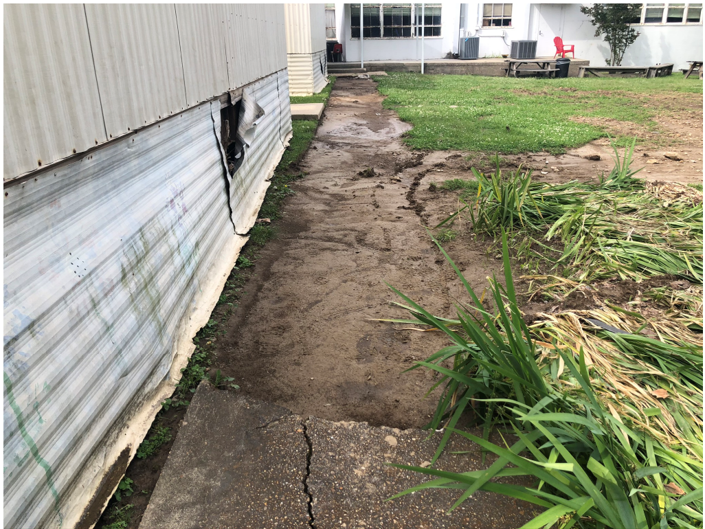
Figure 2 – Demo at Concrete Walk
