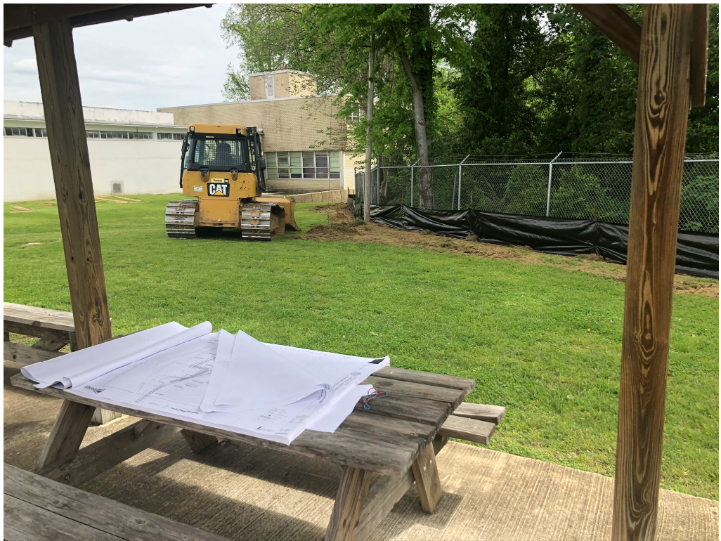
Figure 2 – Silt Fence Install In progress
