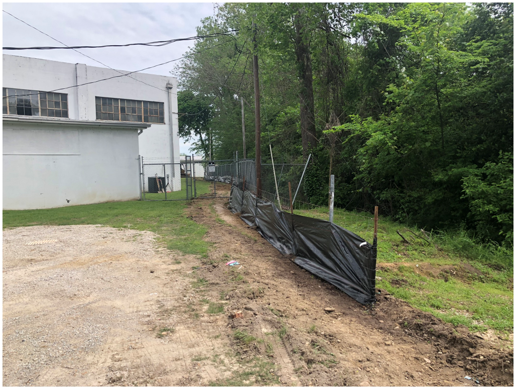
Figure 1 – Silt Fence Install in Progress
