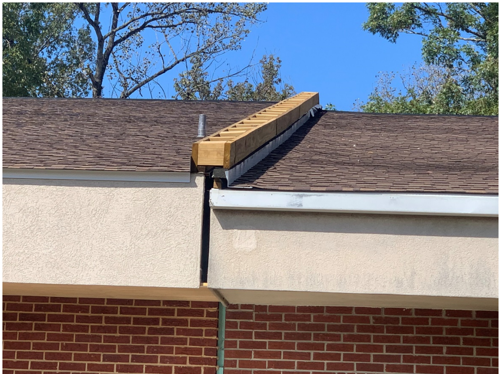
Figure 2 – Framing @ Roofing Connection
