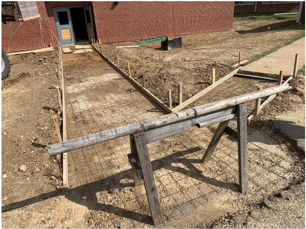
Figure 1 – Sidewalk Formed
