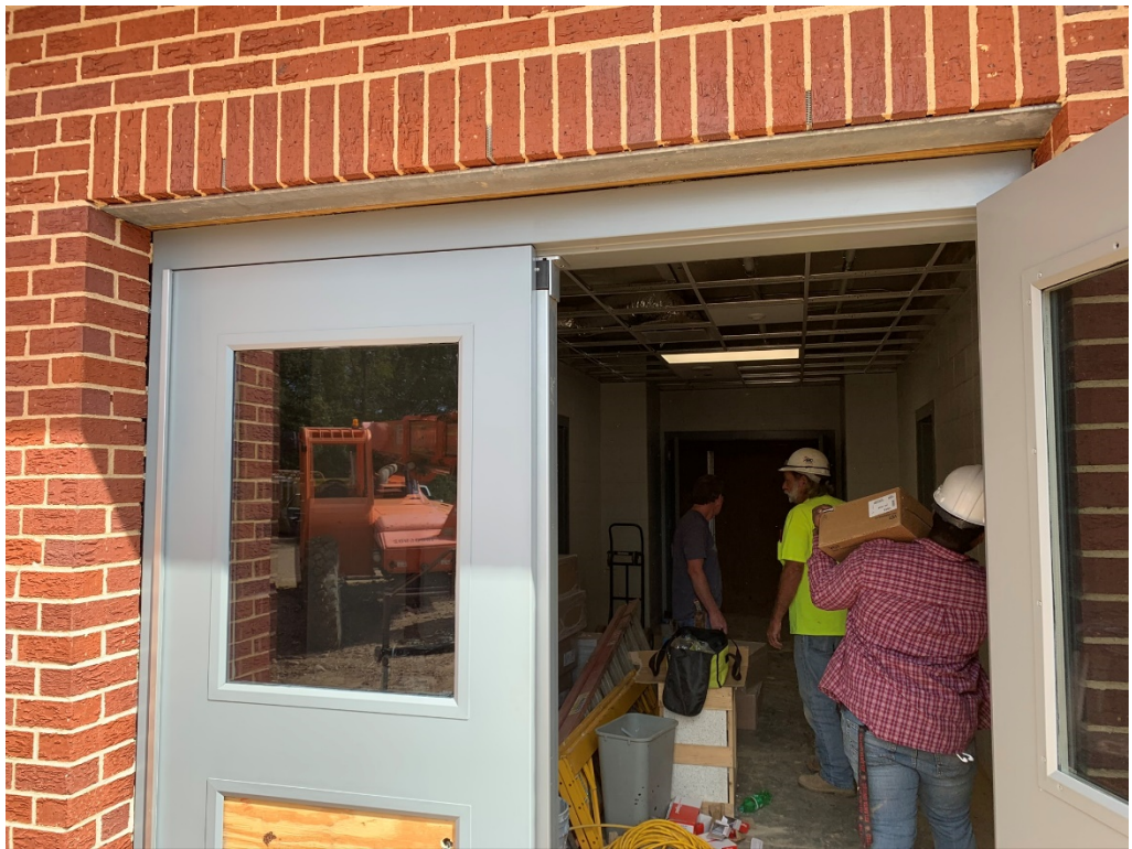
Figure 10 – Glass Installed at Door Panels
