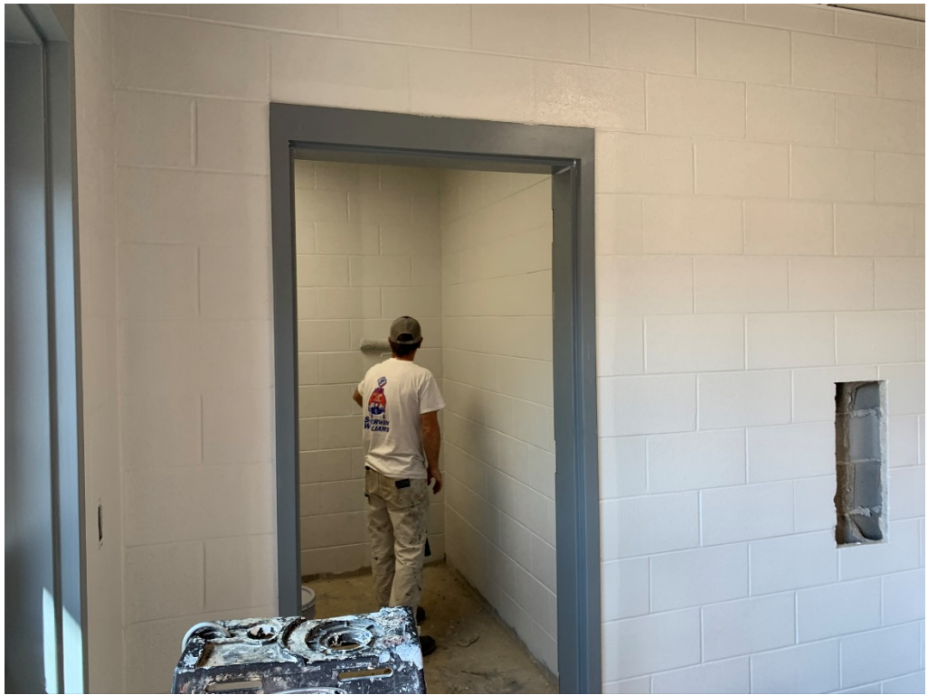
Figure 3 – Paint is ongoing at interior
