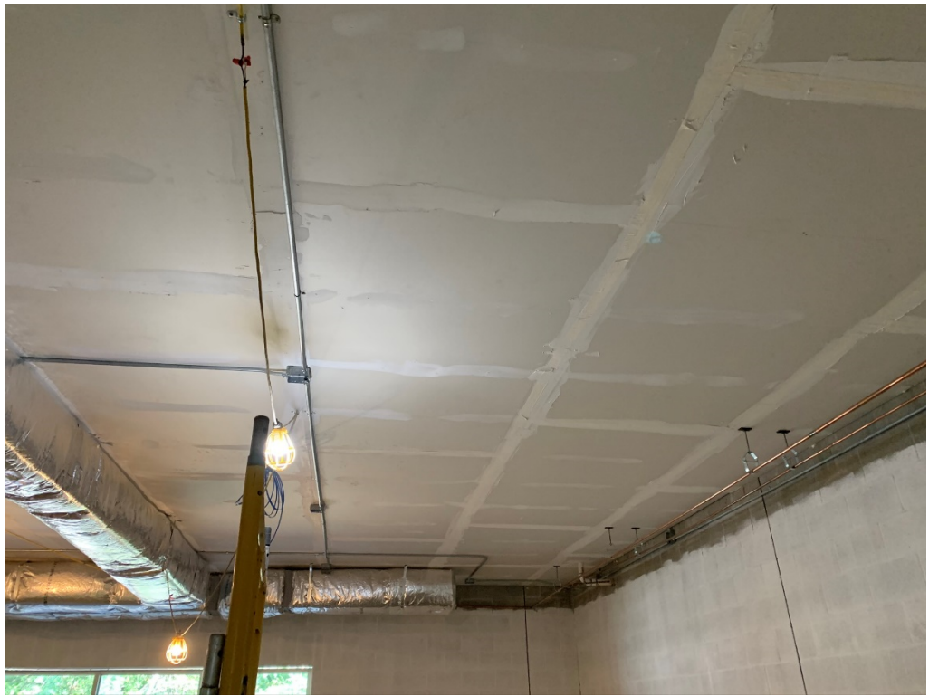
Figure 13 – Services Work at Hard Ceiling is Ongoing
