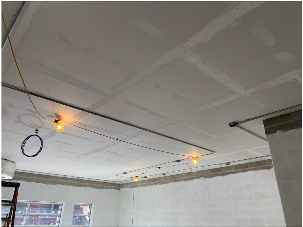
Figure 11 – Services Work at Hard Ceiling is Ongoing
