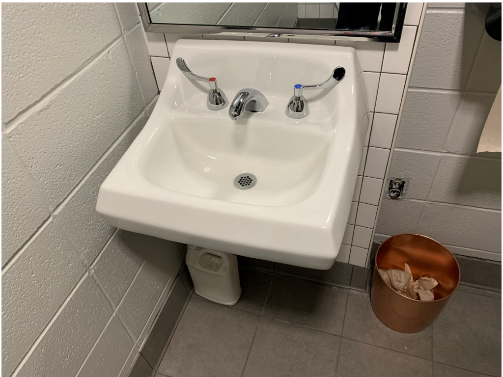
Figure 8 – Several Electrical Code Violations need to be Remedied ASAP
