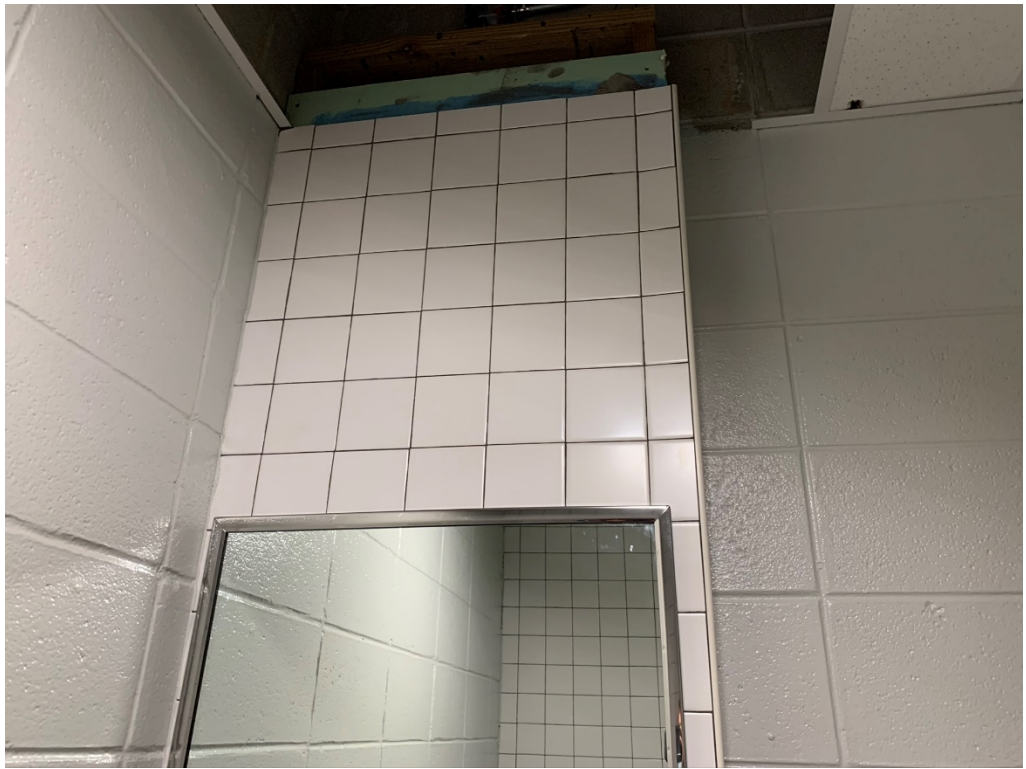
Figure 9 – Staff Toilet Ceiling Work Appears Ongoing
