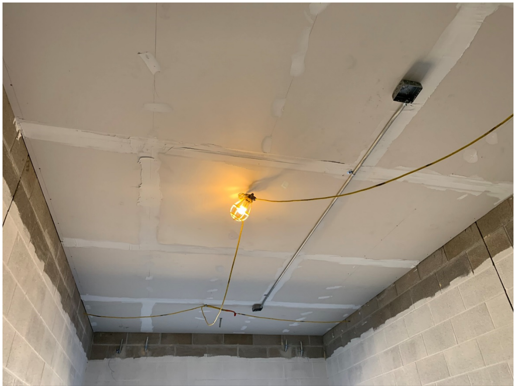
Figure 12 – Services Work at Hard Ceiling is Ongoing
