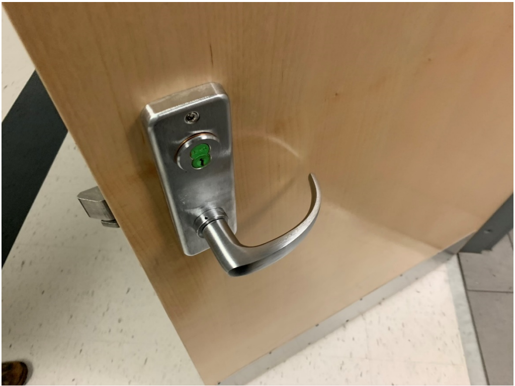
Figure 3 – Hardware at Teacher Bathroom in South Hall
