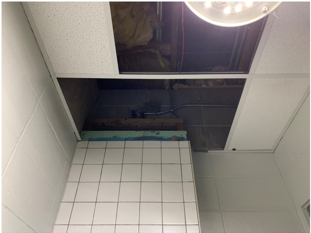
Figure 10 – Staff Toilet Ceiling Work Appears Ongoing
