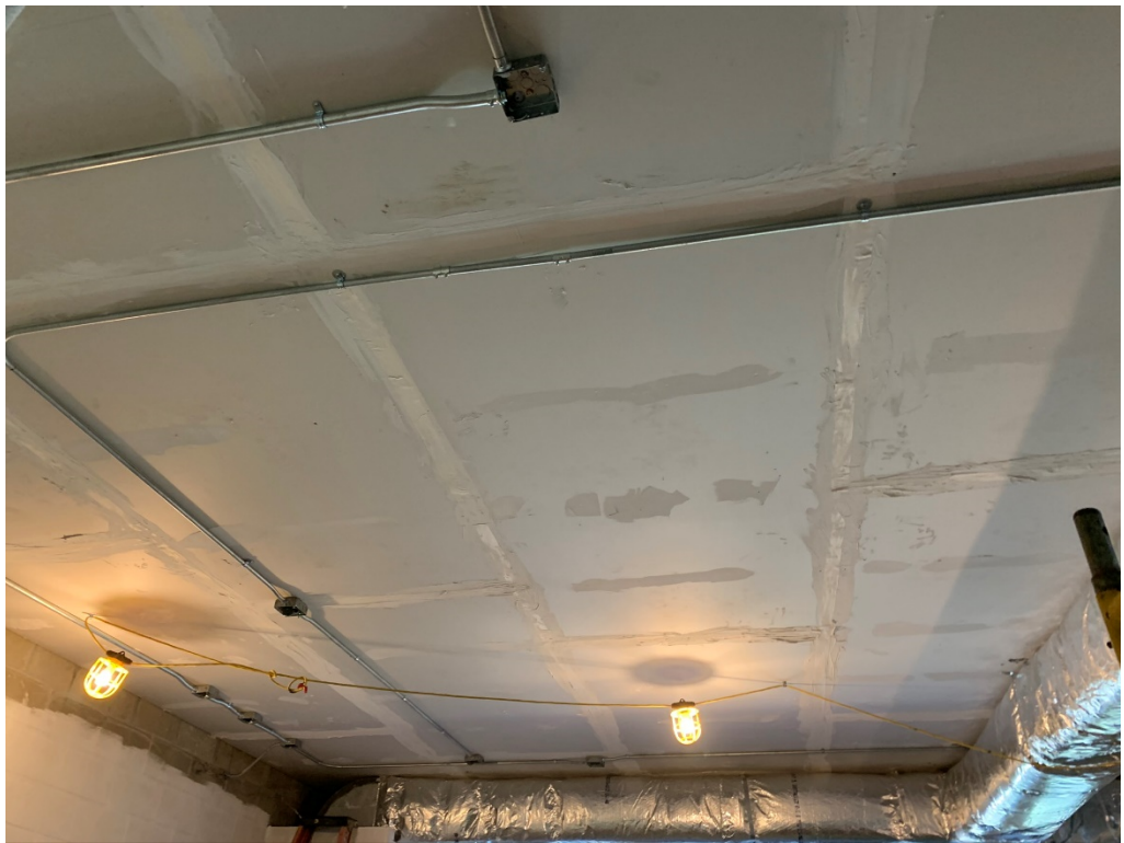
Figure 14 – Services Work at Hard Ceiling is Ongoing
