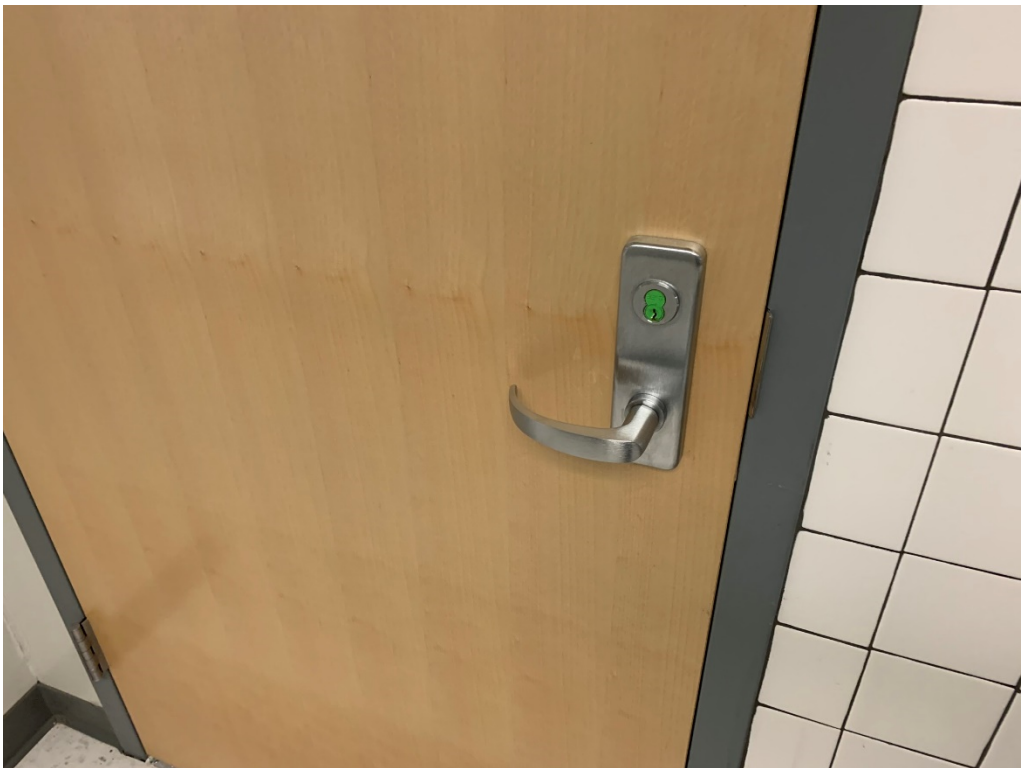
Figure 4 – Hardware at Teacher Bathroom in South Hall
