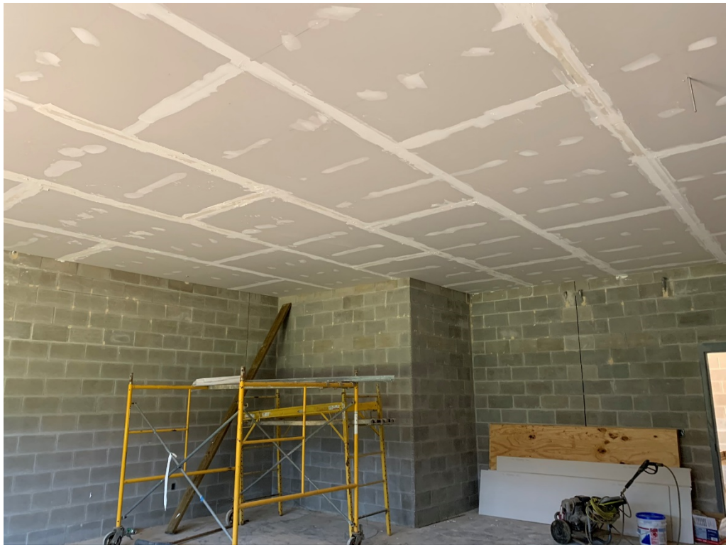
Figure 11 – Hard Ceiling Installed and Level 1 Finish Applied
