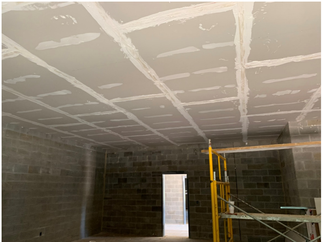
Figure 8 – Hard Ceiling Installed and Level 1 Finish Applied
