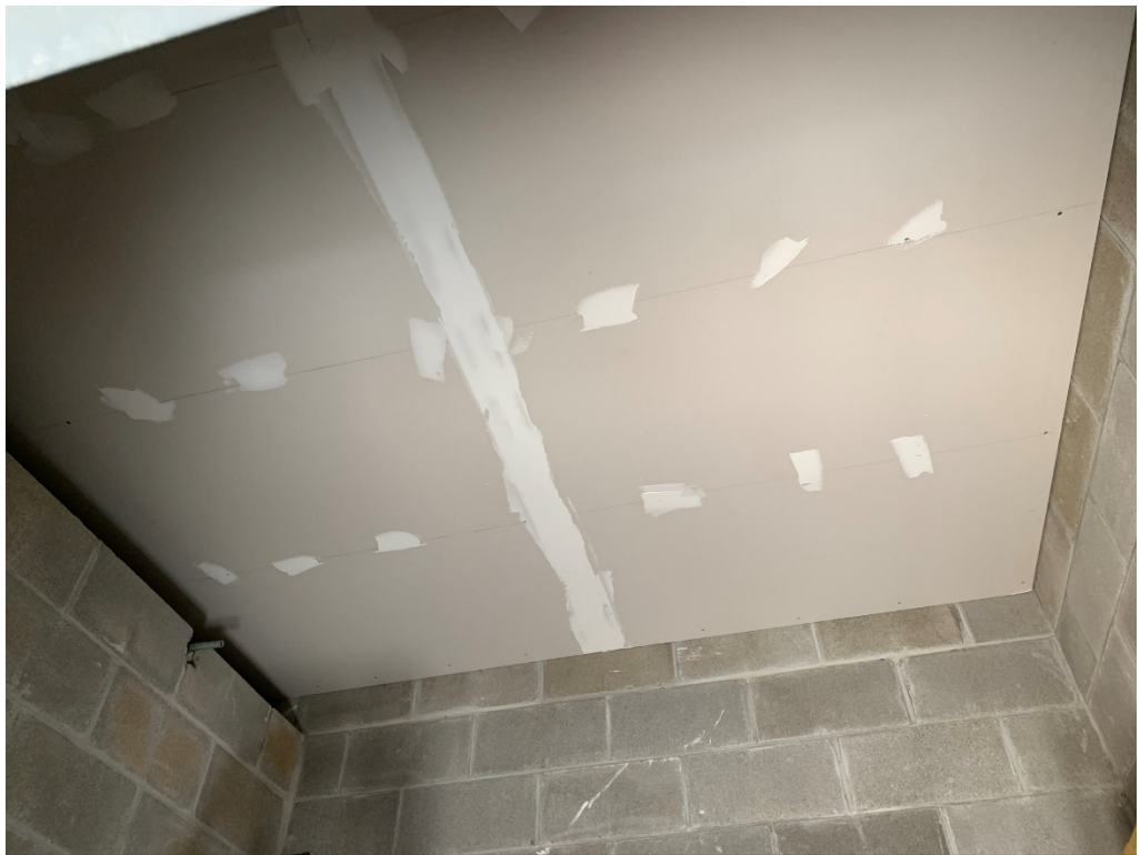
Figure 6 – Hard Ceiling Installed and Level 1 Finish Applied
