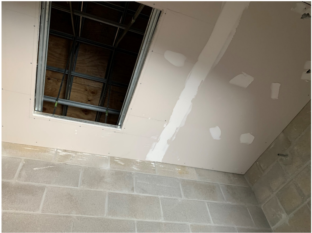
Figure 7 – Hard Ceiling Installed and Level 1 Finish Applied
