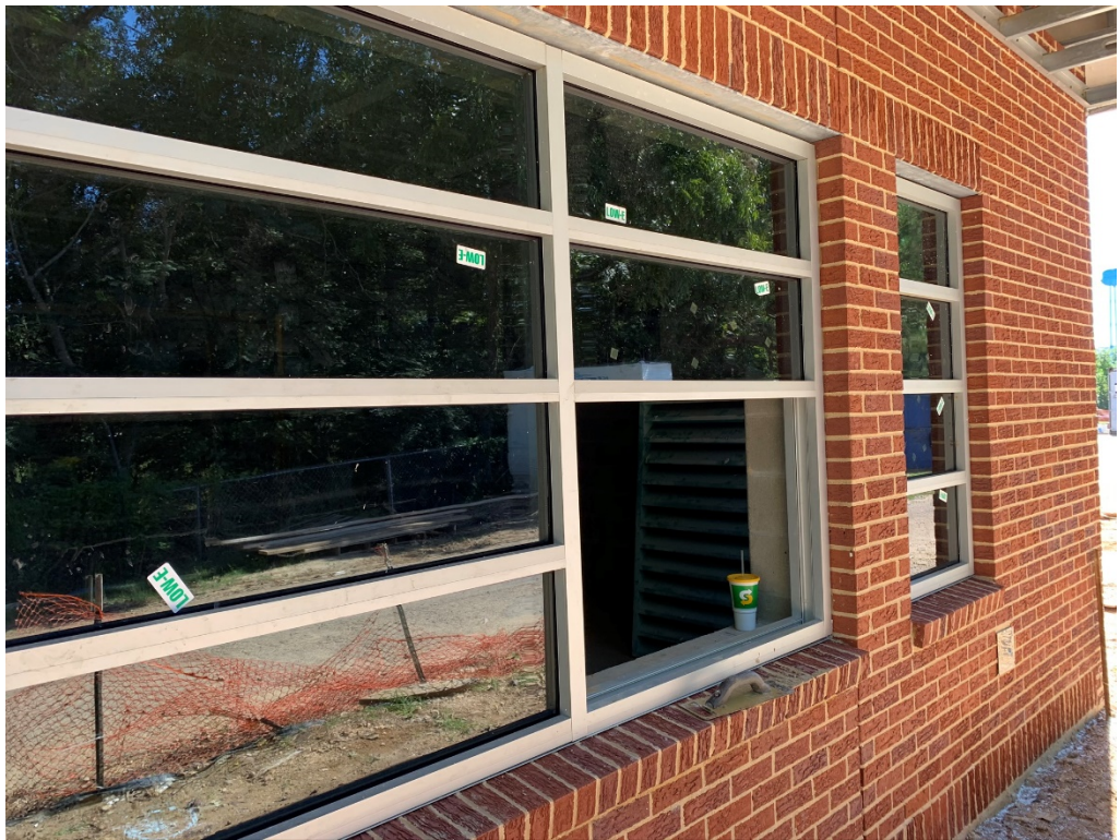
Figure 2 – Glazing in Place; awaiting egress panel
