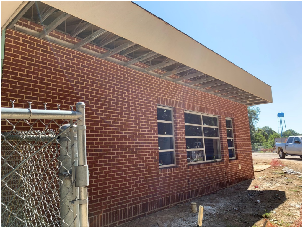
Figure 1 – Exterior Work Ongoing
