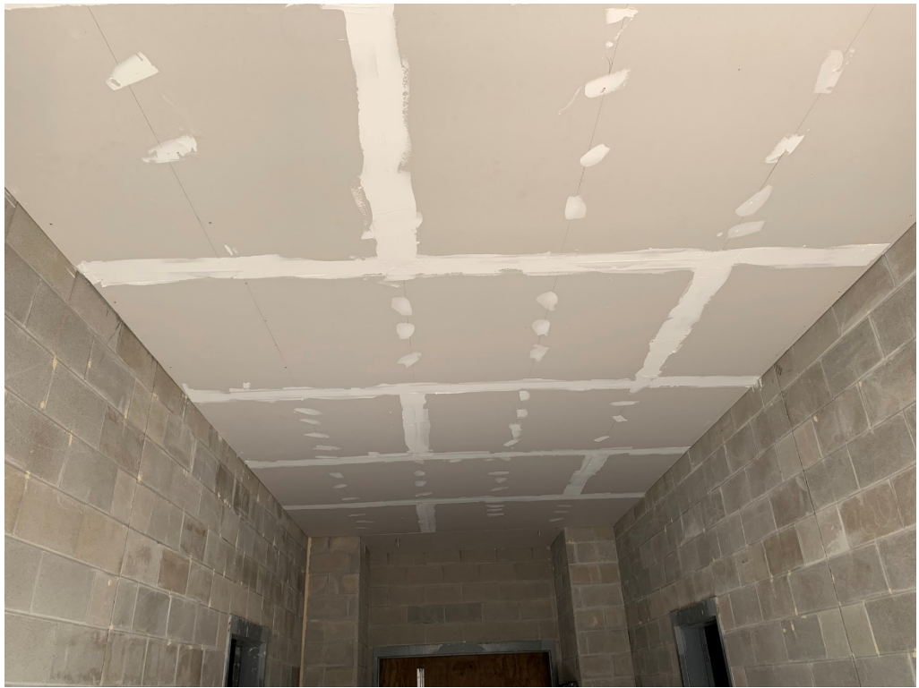
Figure 5 – Hard Ceiling Installed and Level 1 Finish Applied
