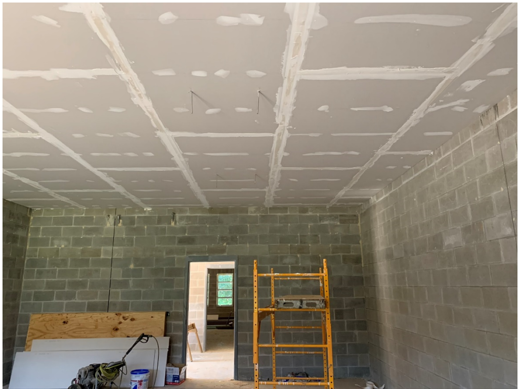
Figure 12 – Hard Ceiling Installed and Level 1 Finish Applied
