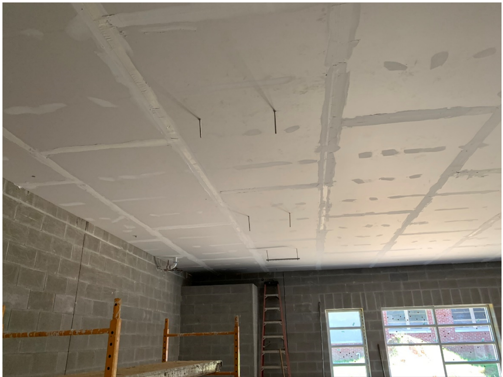
Figure 10 – Hard Ceiling Installed and Level 1 Finish Applied
