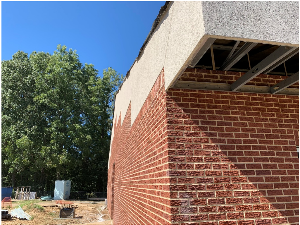
Figure 3 – Stucco Finished at Soffit
