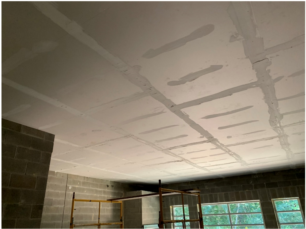
Figure 9 – Hard Ceiling Installed and Level 1 Finish Applied
