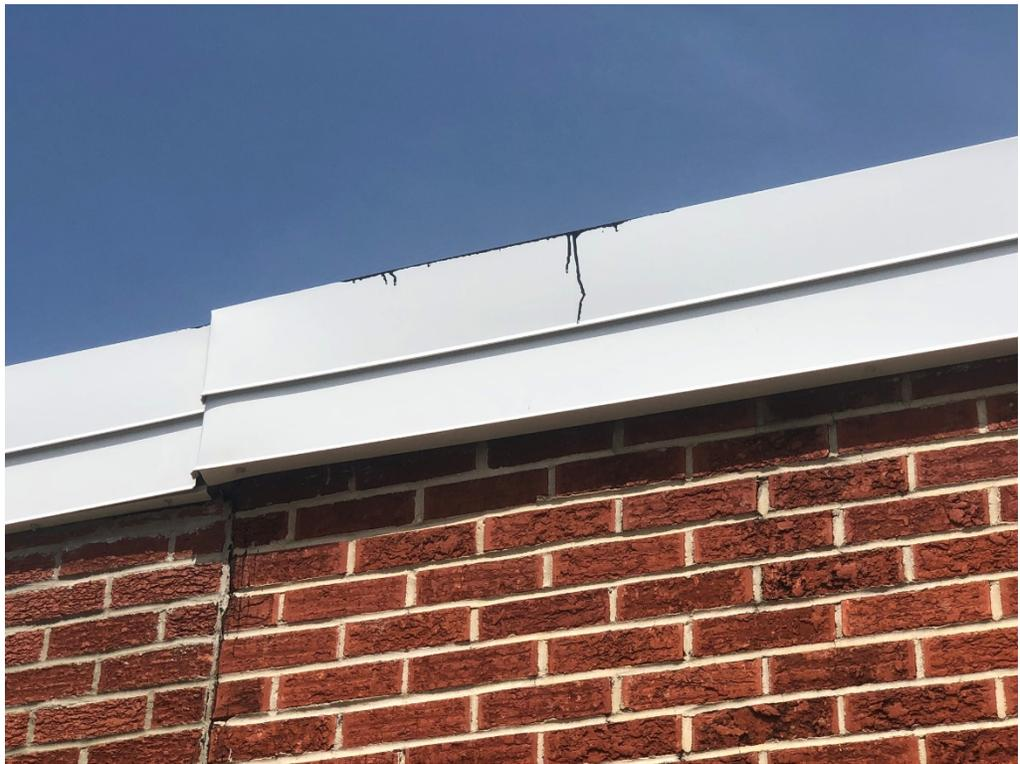
Figure 4 – Asphalt Drips at New Eave Trim (remove drip from face)
