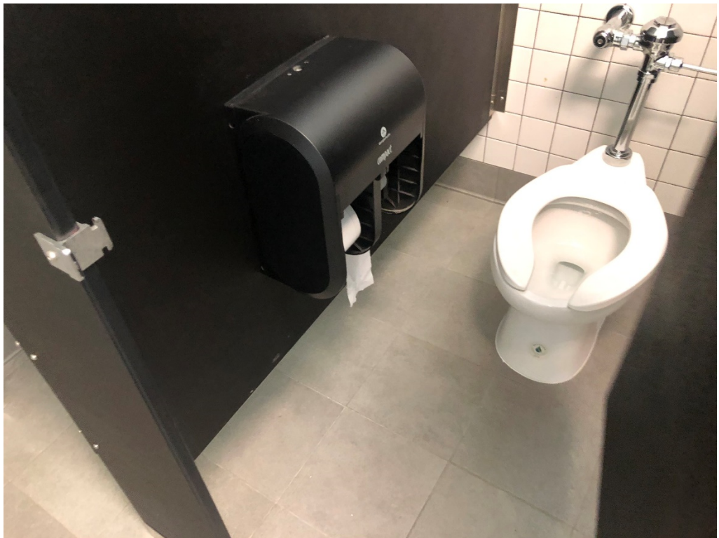
Figure 10 – Toilet Paper Towel Holders Installed
