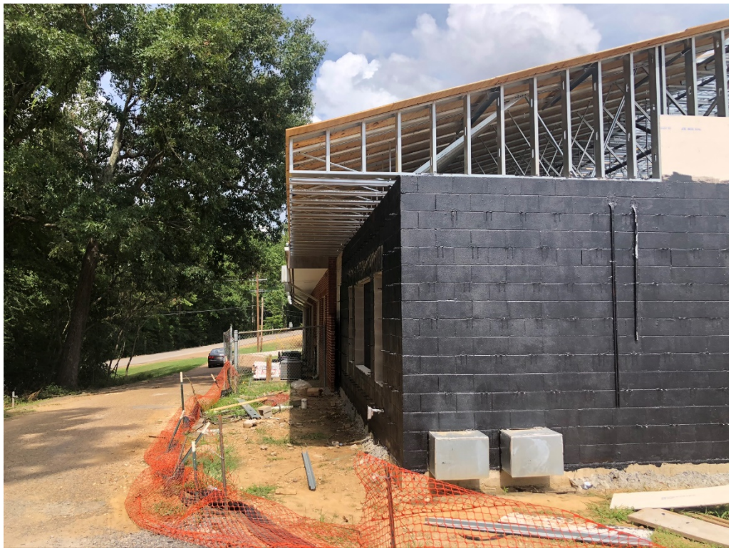
Figure 2 – Decking Partially Installed
