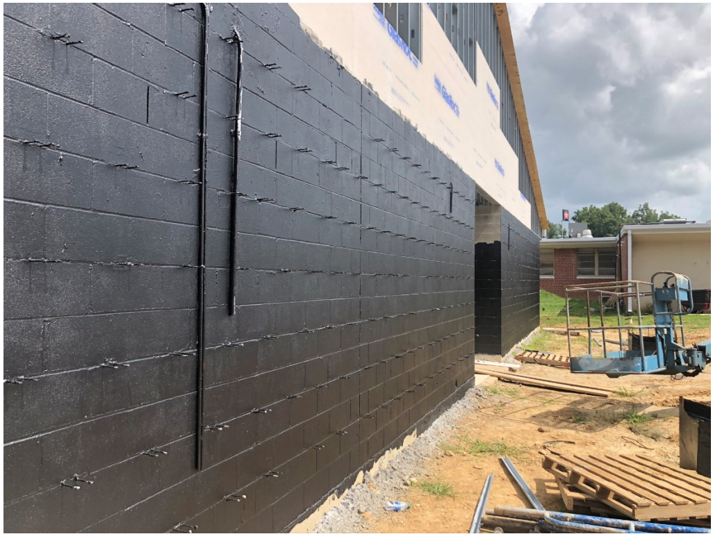
Figure 5 – Exterior Rock Partially Installed
