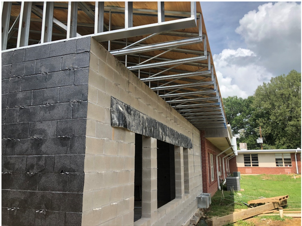
Figure 6 – Water-Proofing Partially Installed
