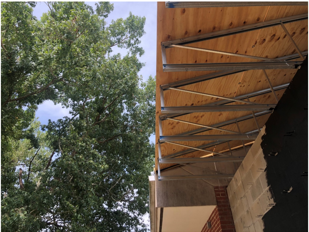
Figure 4 – Roof Edge at North Side of Building
