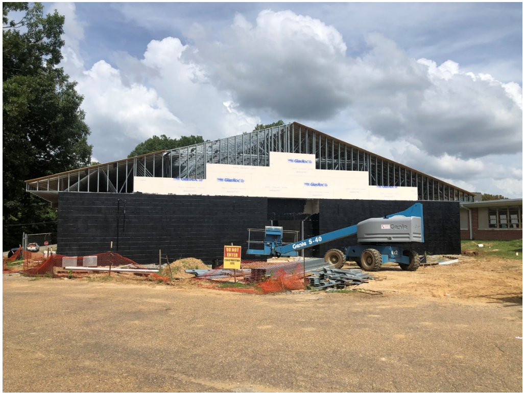
Figure 1 – On-going build at Addition
