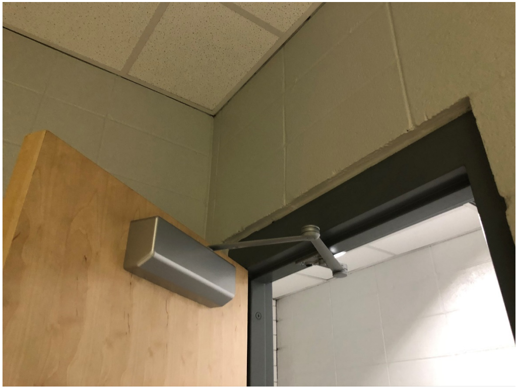
Figure 15 – Closer Opens Approx. 70 degrees
