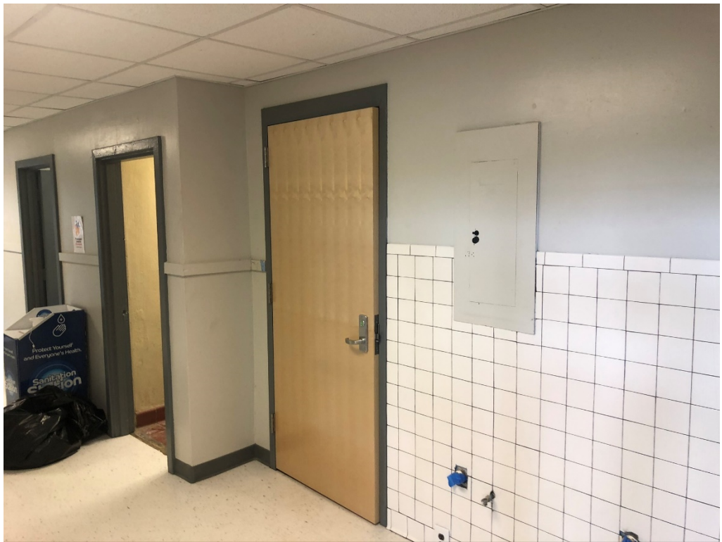
Figure 16 – Door Panels Installed
