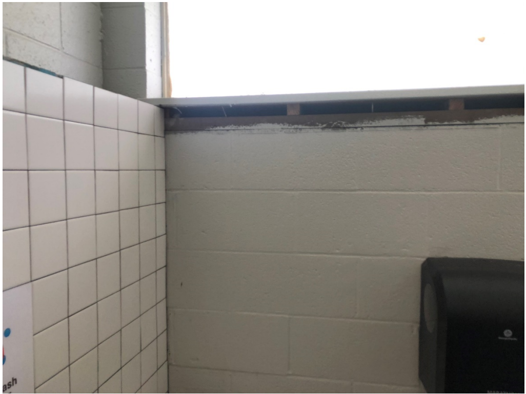
Figure 11 – Finishing Still Needed at top of Walls
