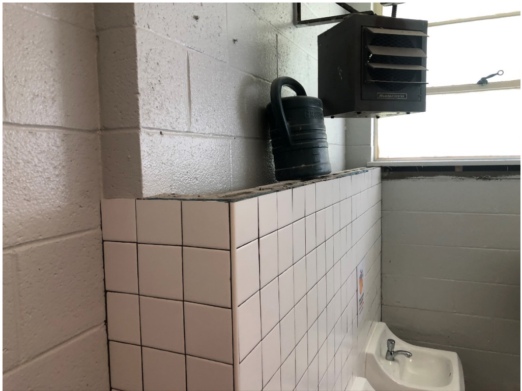
Figure 12 – Caps Required at Wall Tops
