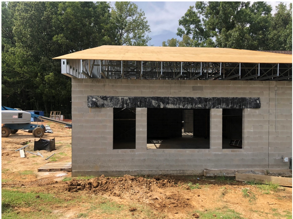
Figure 8 – Decking Partially Installed
