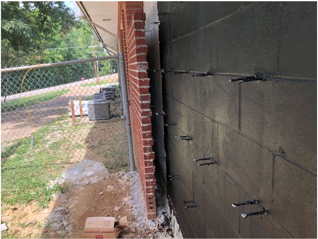
Figure 3 – Brick Mockup and example of Air Gap
