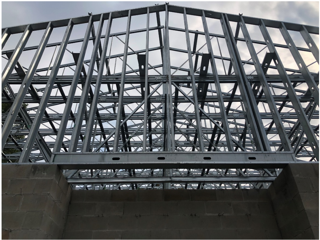
Figure 3 – Trusses Complete
