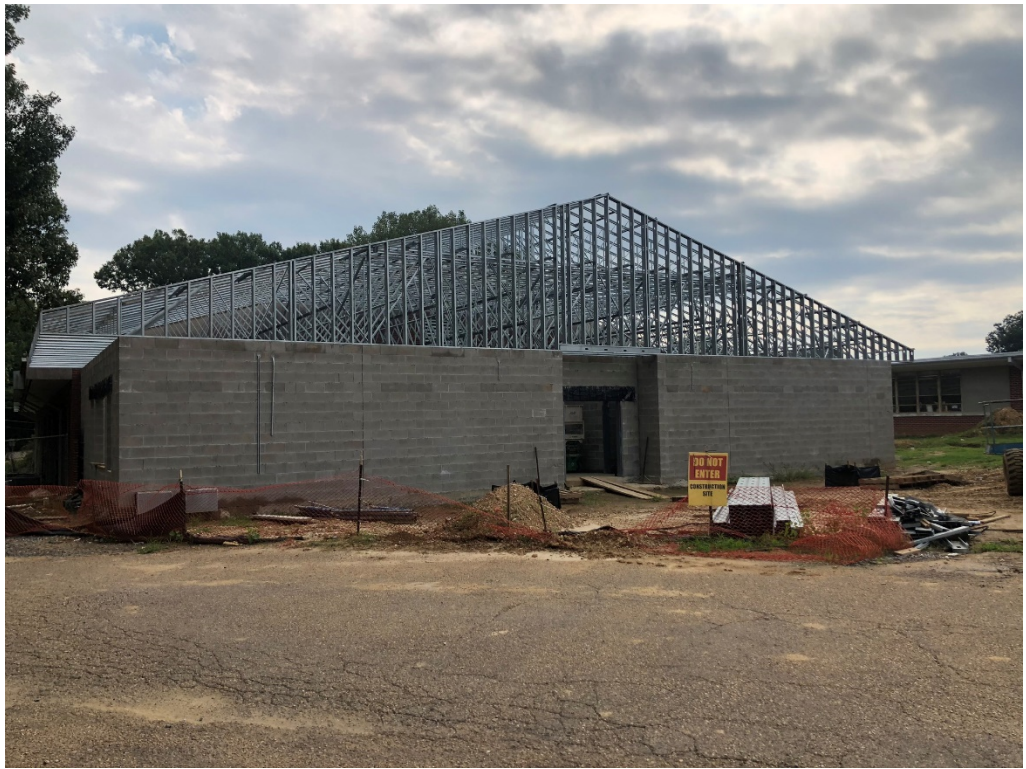
Figure 1 – Metal Trusses Complete and Ready for Decking
