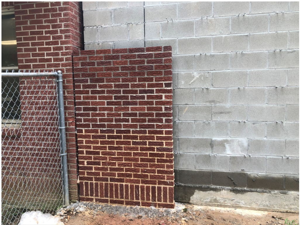
Figure 2 – Masonry Sample Wall
