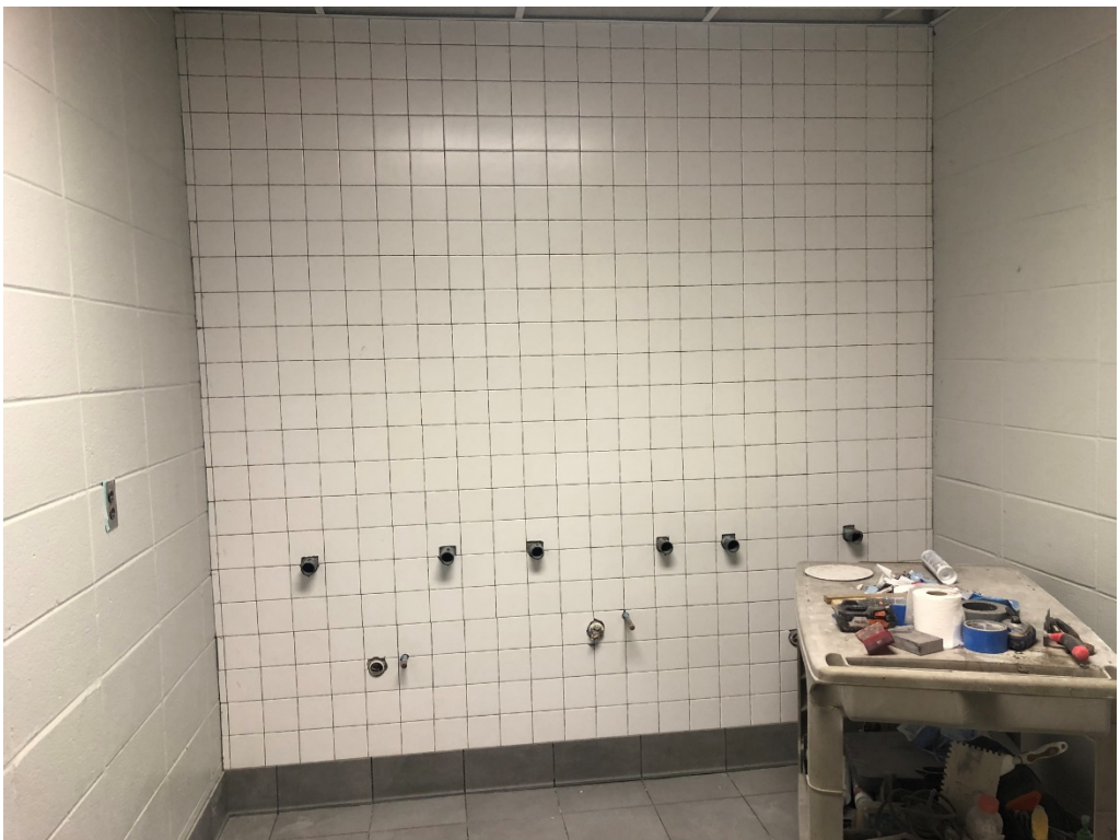
Figure 6 – Tile at Wet Wall
