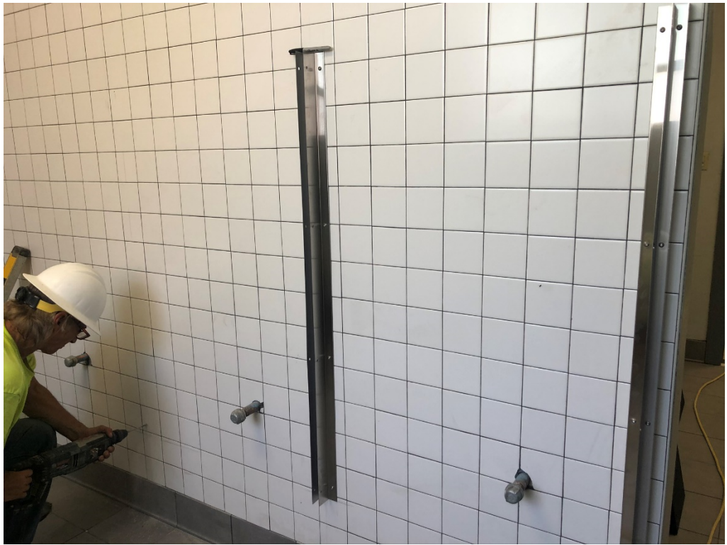
Figure 11 – Toiler Partition Installation
