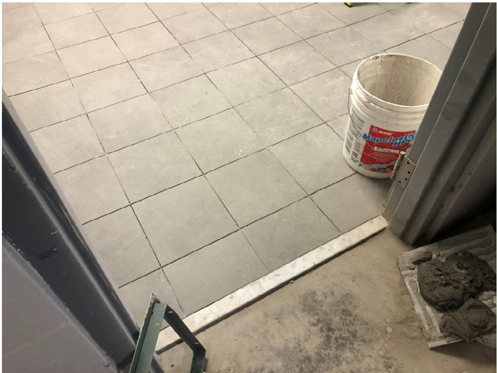
Figure 5 – Marble Threshold Installed
