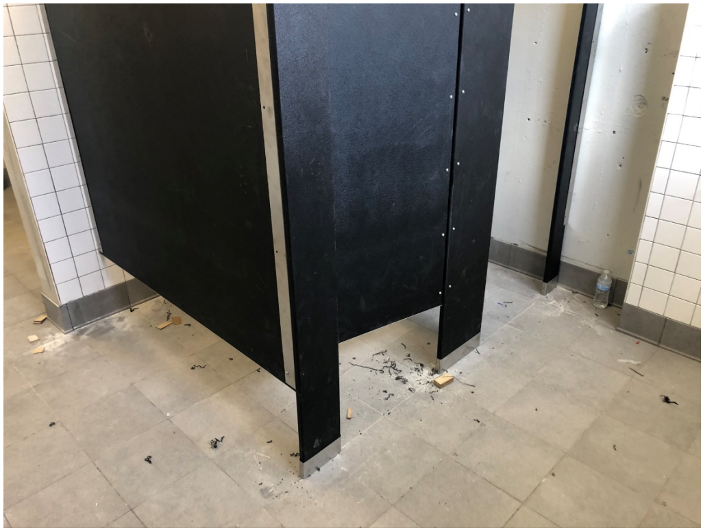
Figure 12 – Toiler Partition Installation
