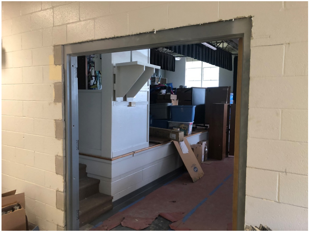
Figure 1 – Steel Frame Installed at Auditorium
