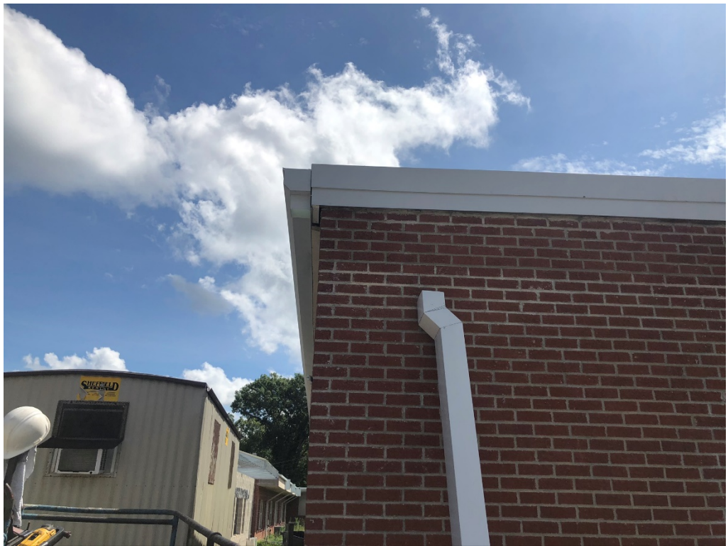
Figure 10 – New Metal Edge Trim & Downspout ready to install
