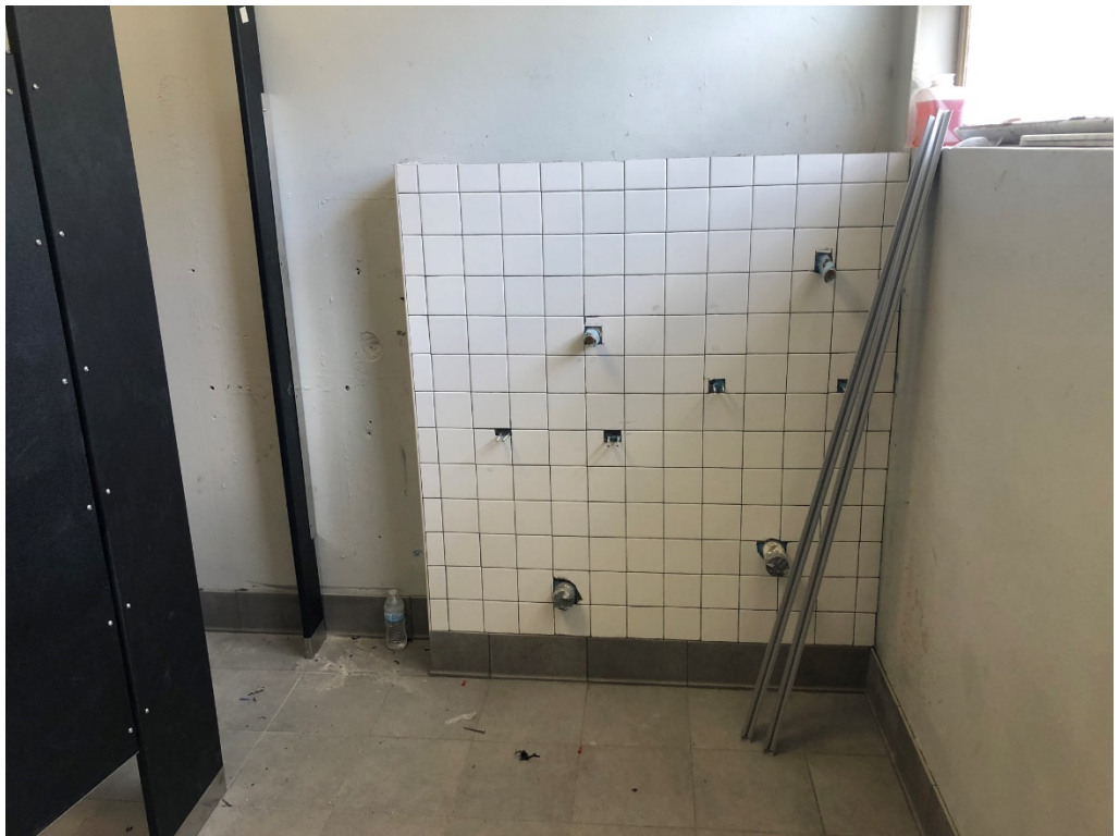
Figure 14 – Tile at Urinal Wall
