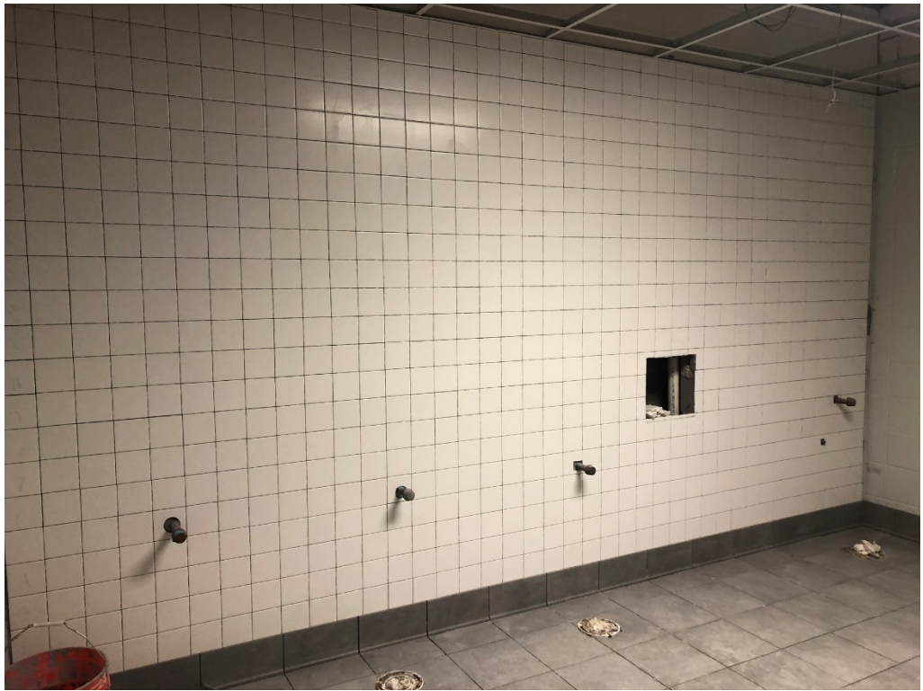
Figure 7 – Tile at Wet Wall
