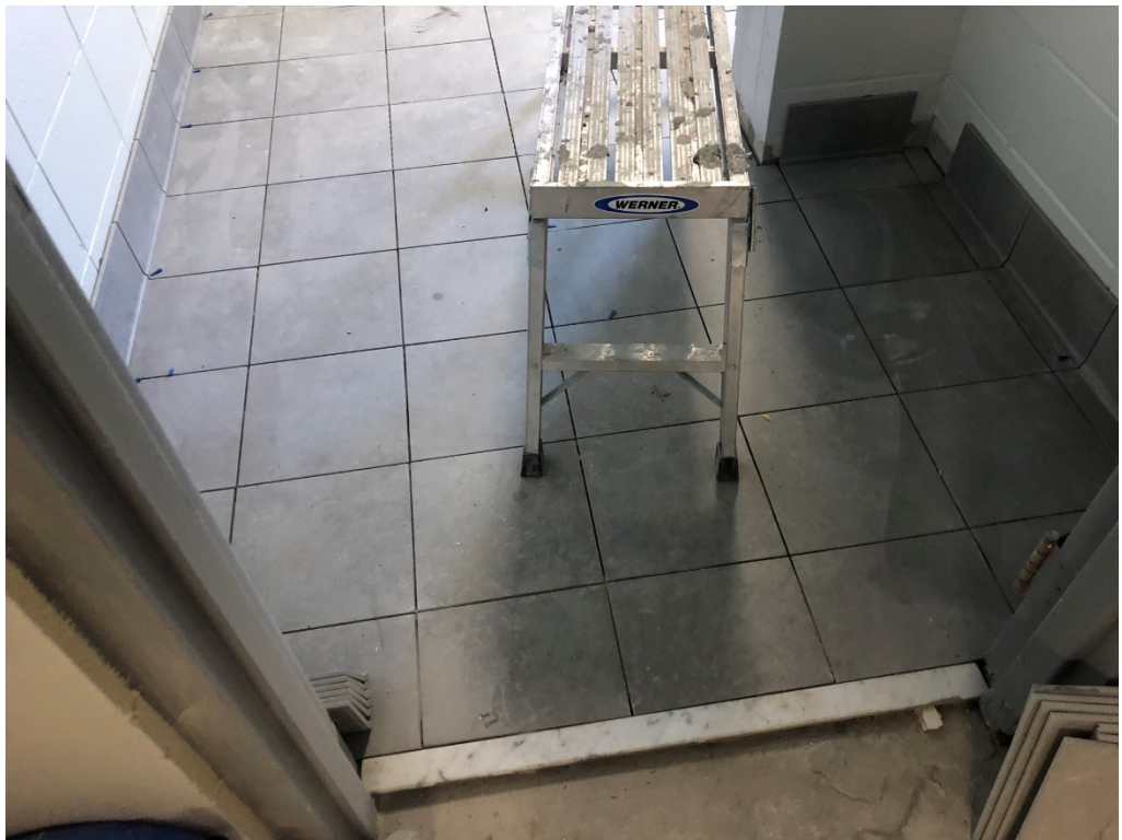
Figure 8 – Tile at Wet Wall
