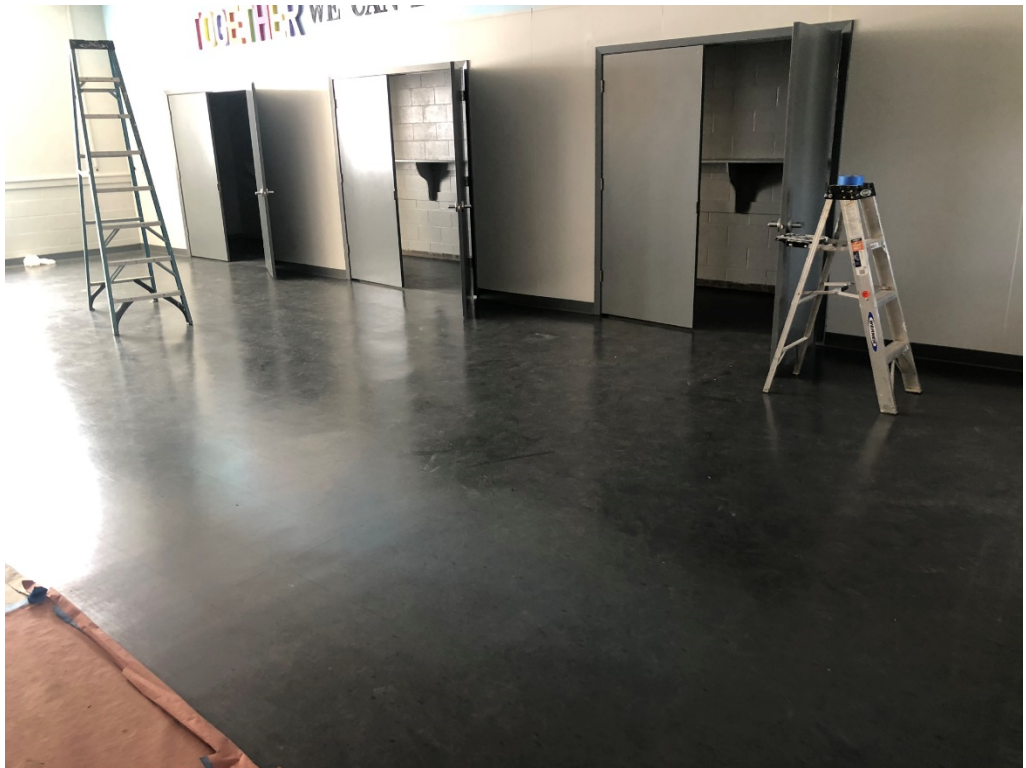
Figure 2 – VCT installed and Waxed at Auditorium
