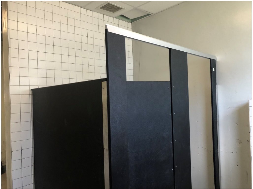
Figure 13 – Toiler Partition Installation
