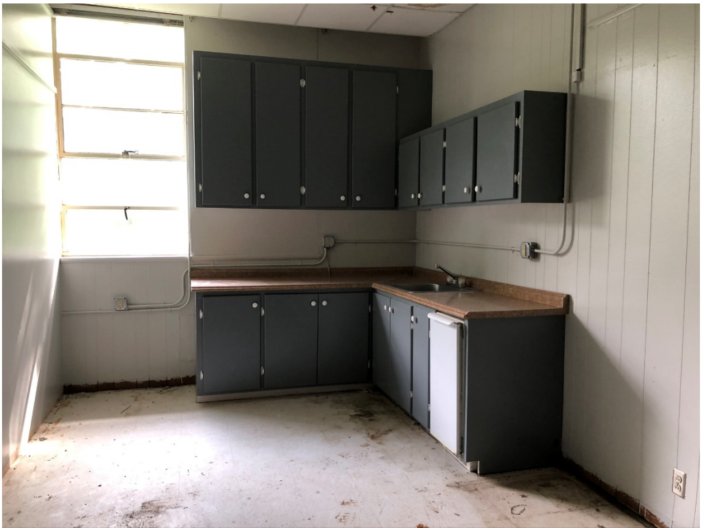
Figure 6 – Cabs Painted; paint, overall, is ongoing
