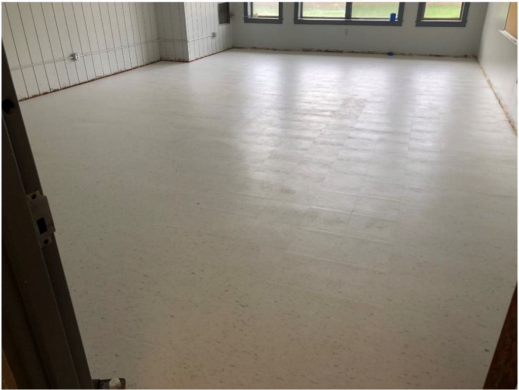
Figure 7 – VCT Install at North hall Classrooms is ongoing
