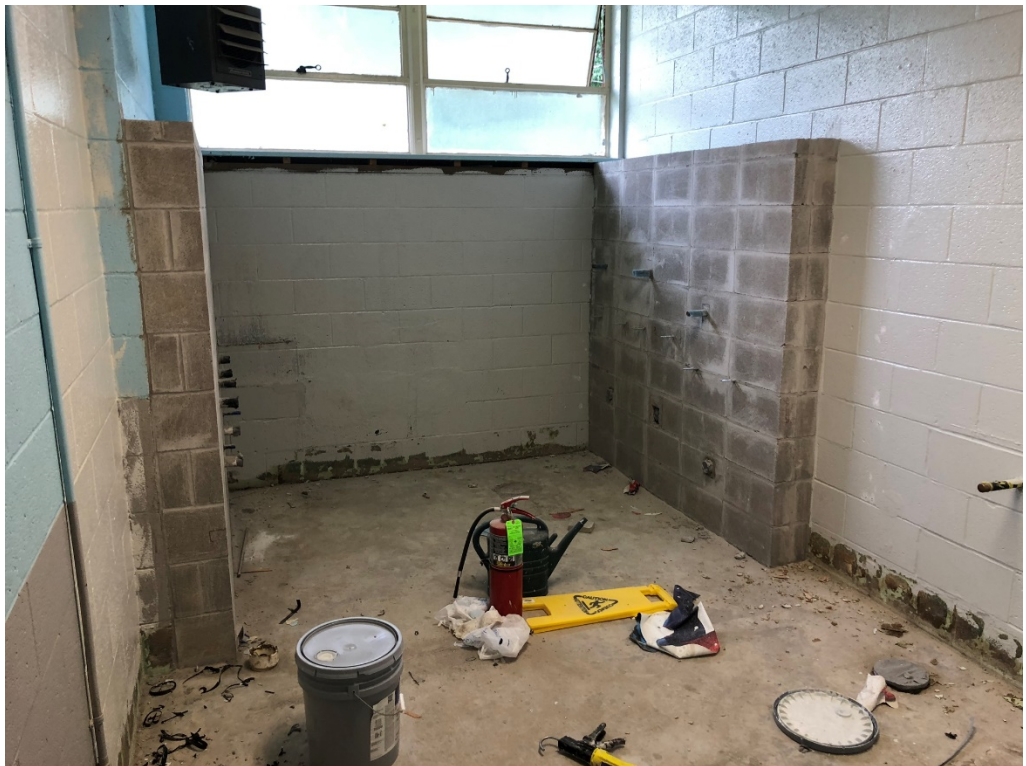
Figure 4 – CMU Complete in Bathroom Areas
