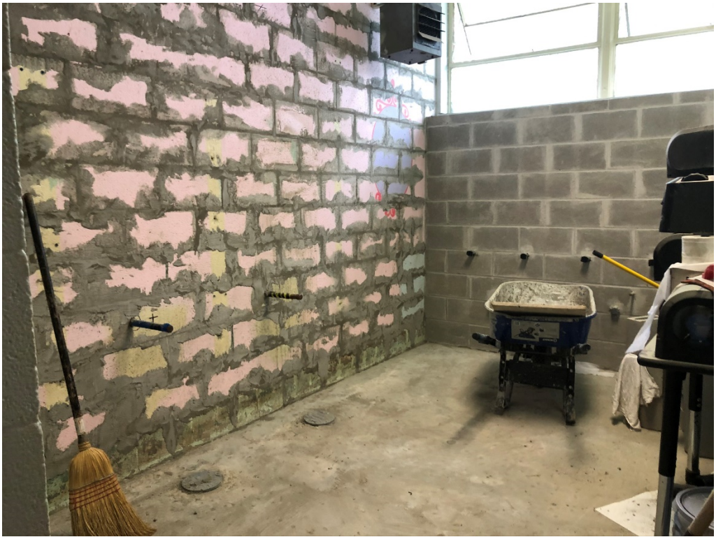
Figure 5 – Wall Patch In Progress at Existing CMU
