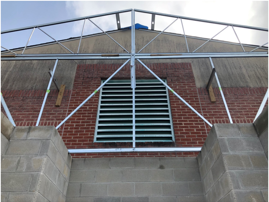
Figure 8 – Truss set at Addition
