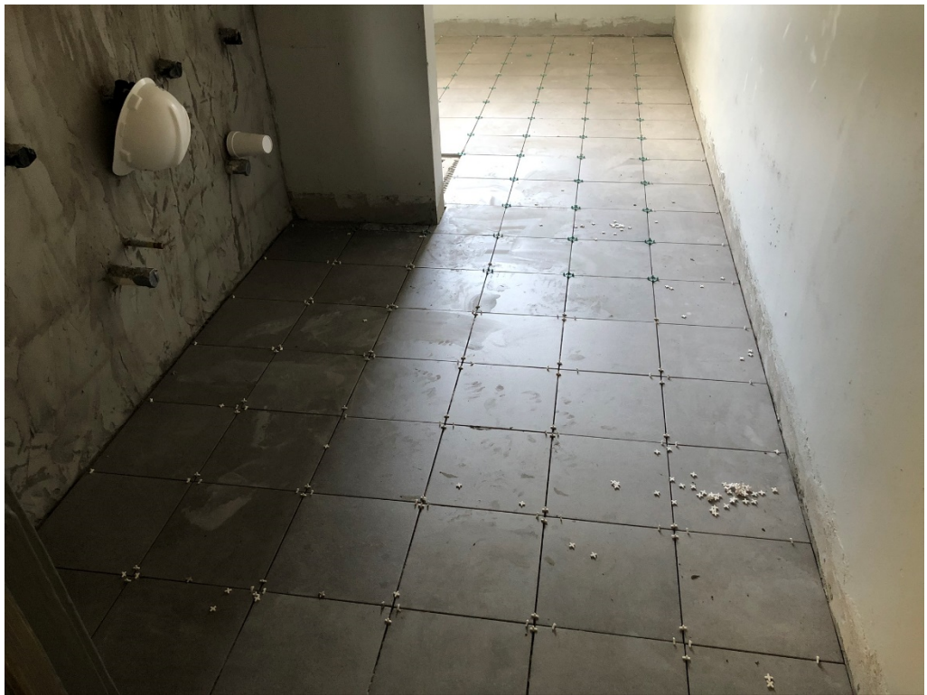
Figure 2 – Tile Work in progress at Bathrooms
