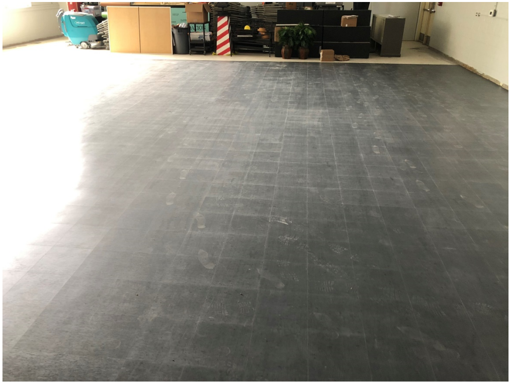
Figure 1 – VCT Tile Installation at Auditorium
