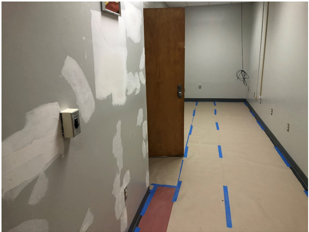
Figure 4 – Paint Prep is Ongoing
