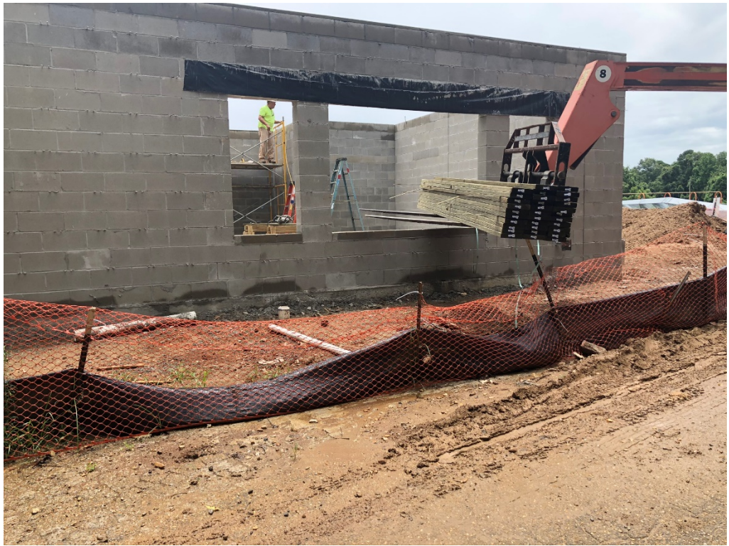
Figure 1 – Treated Boards Set As Plate for Trusses
