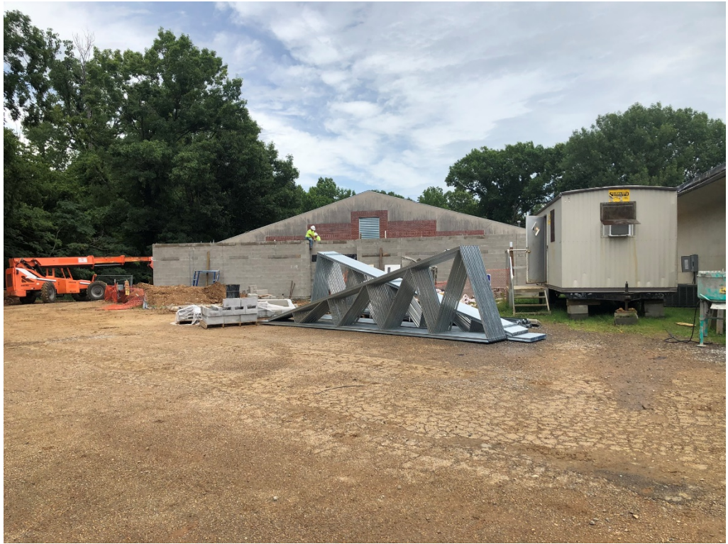
Figure 7 – Trusses On Site
