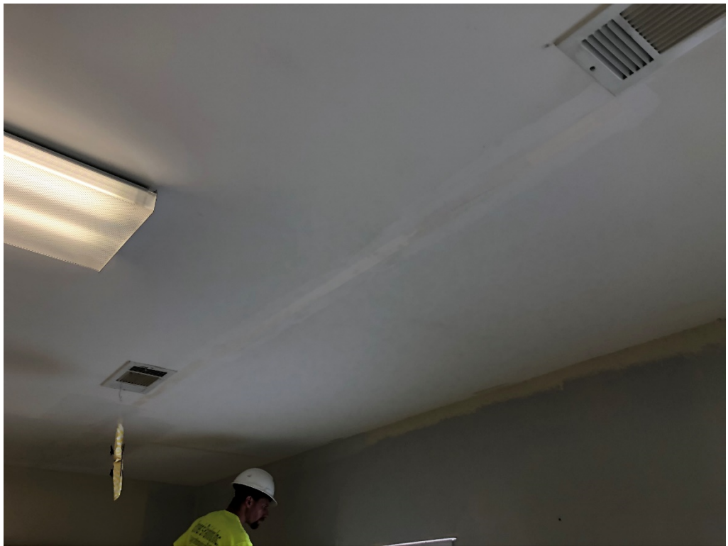
Figure 6 – Ceiling Prep at Cafeteria
