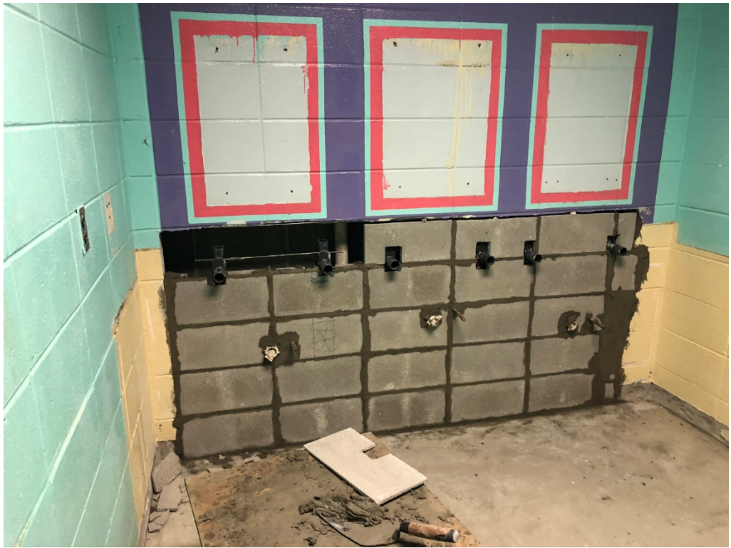
Figure 3 – Continued Masonry Repair
