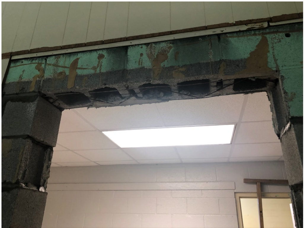
Figure 2 – Interior Header at New Entry @ Workroom 25
