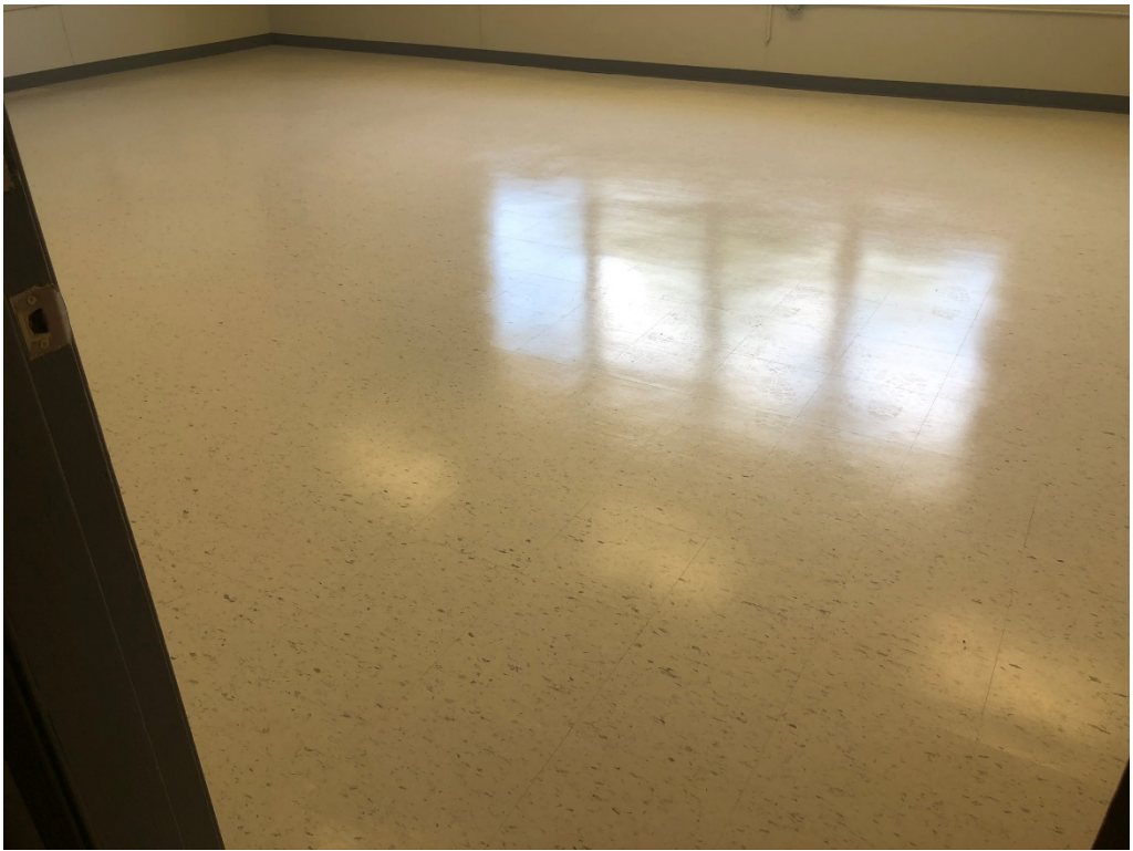
Figure 5 – NEW VCT at North side Classrooms of South Hall
