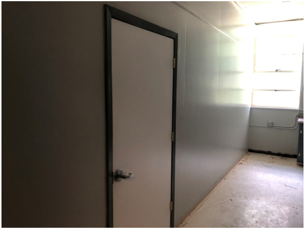
Figure 3 – Paint Work is Ongoing
