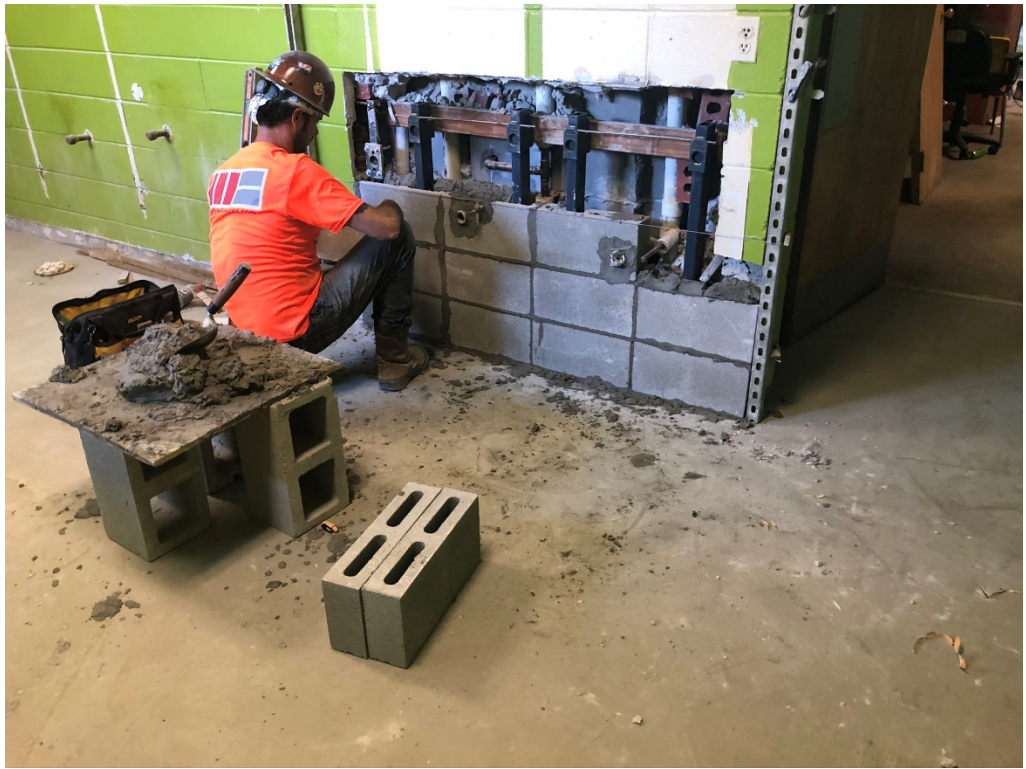
Figure 7 – Block Work at Boys T1
