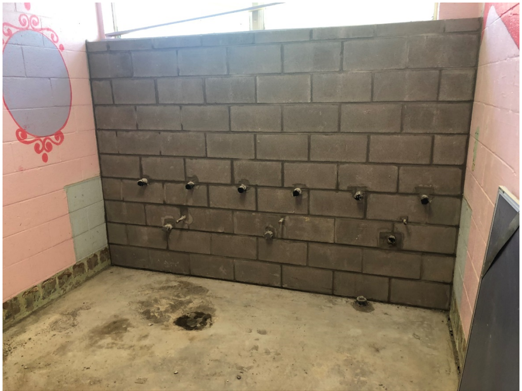
Figure 4 – Block Work at Boys T5
