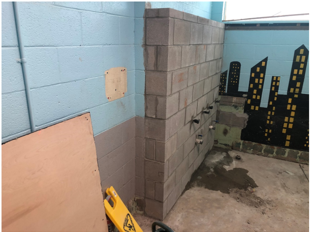
Figure 10 – Block Work at Boys T10
