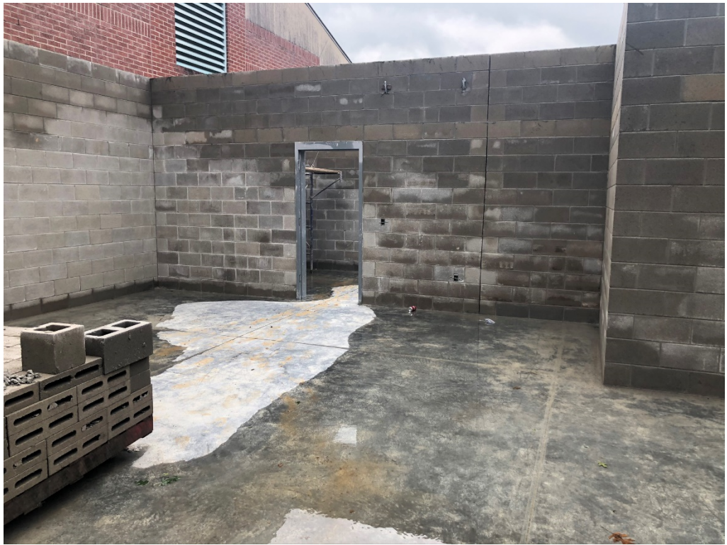
Figure 7 – Addition Interior: STEM 101
