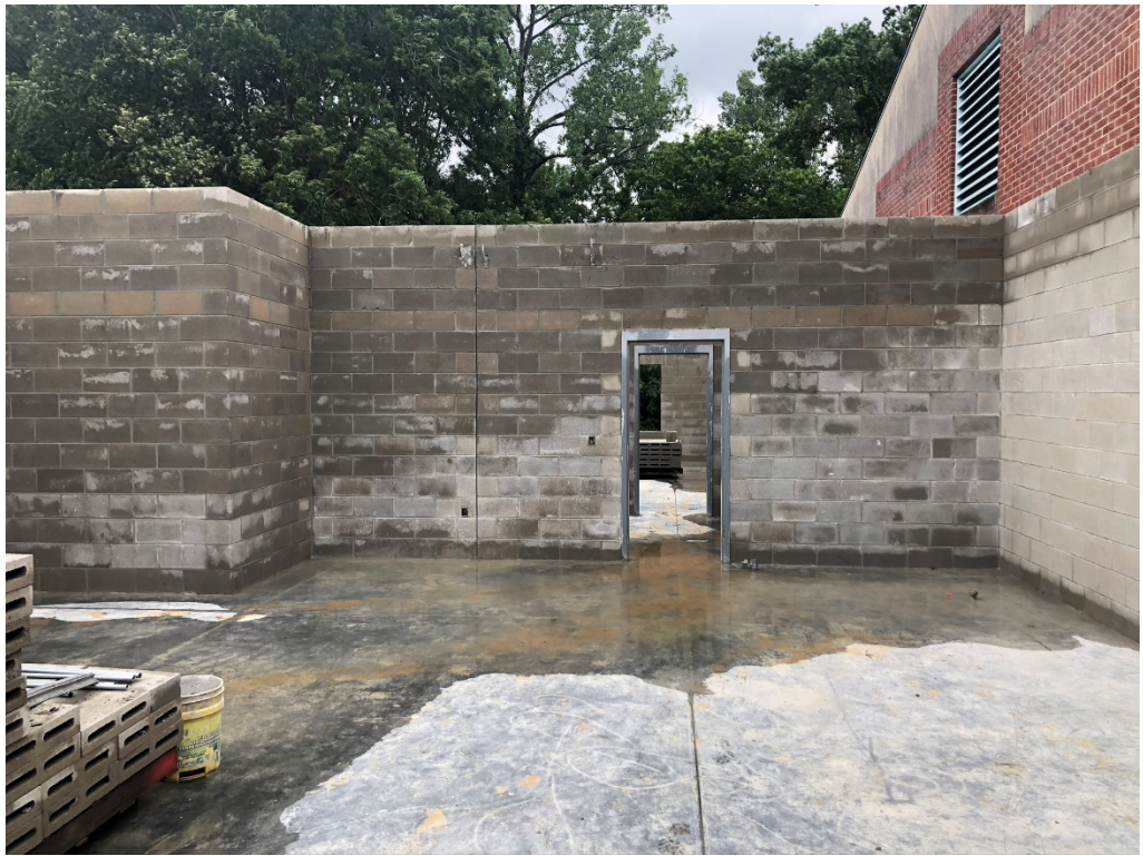
Figure 11 – Addition Interior: Music 102
