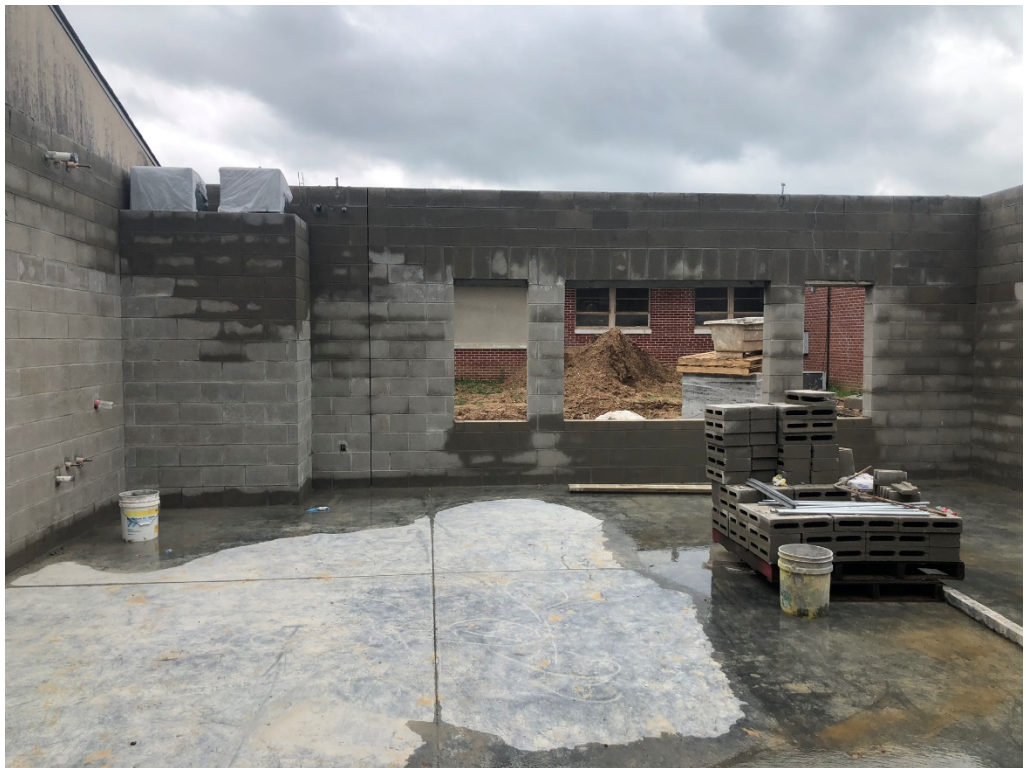
Figure 12 – Addition Interior: Music 102
