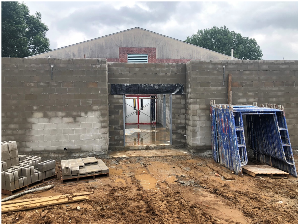
Figure 6 – Addition Ready for Trusses
