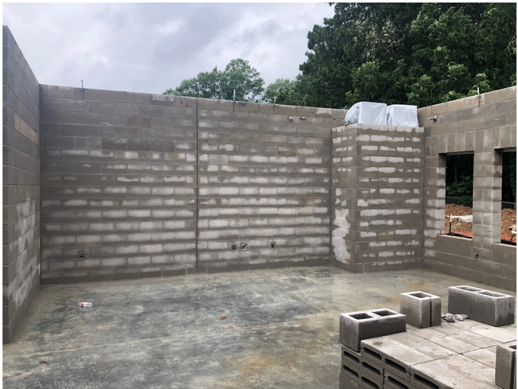
Figure 8 – Addition Interior: STEM 101
