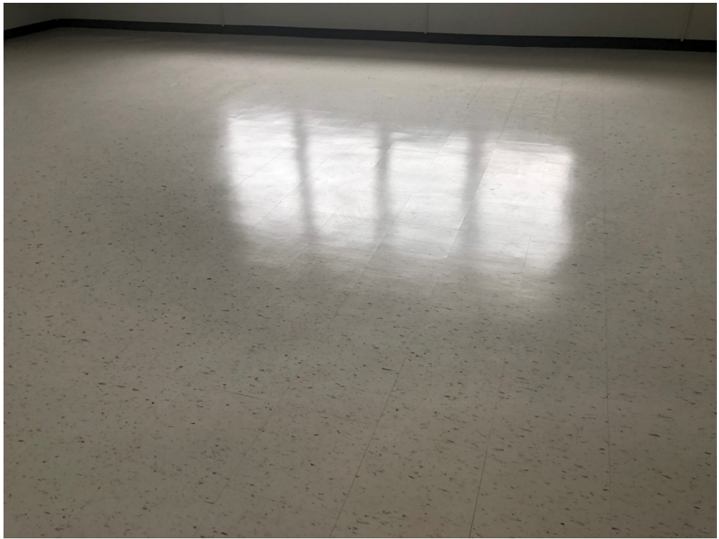
Figure 5 – NEW VCT has Been Waxed in South Side of South Hall Rooms
