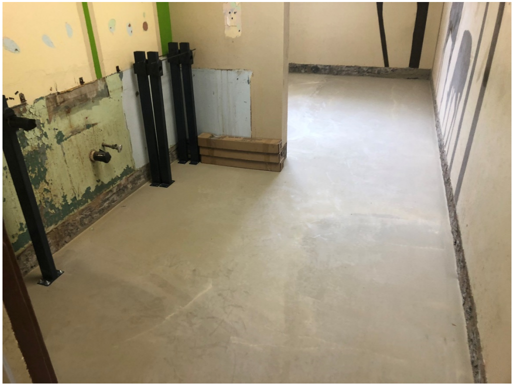
Figure 3 – Counter Steel Carriers Installed
