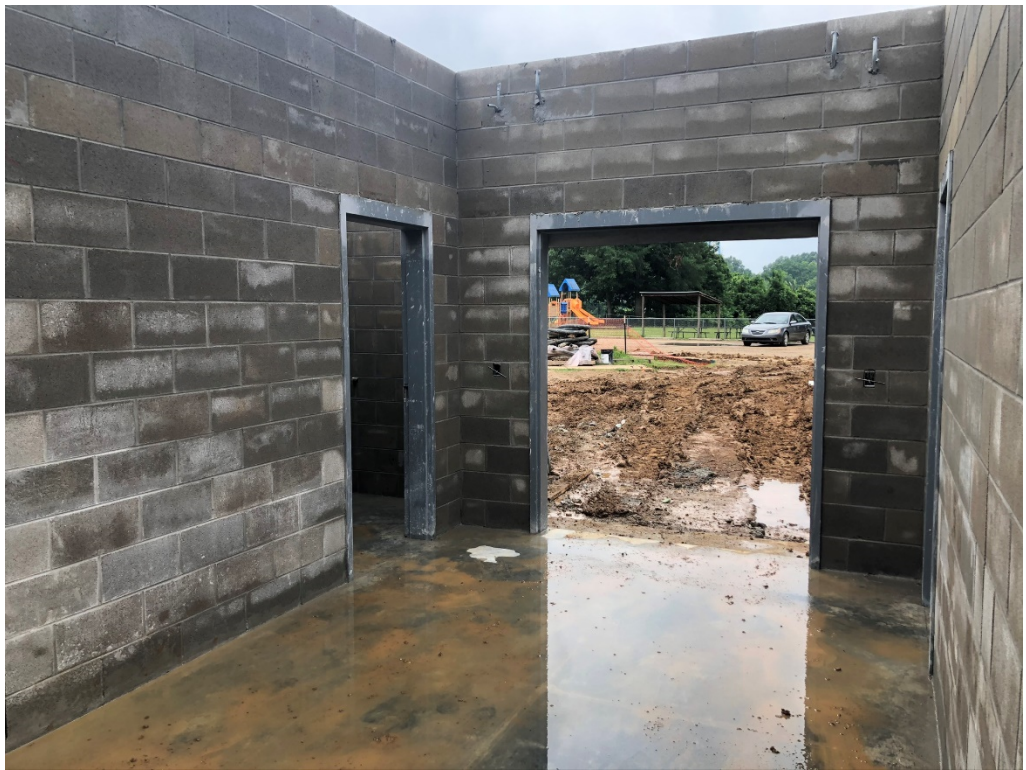
Figure 10 – Addition Interior: Corridor 104
