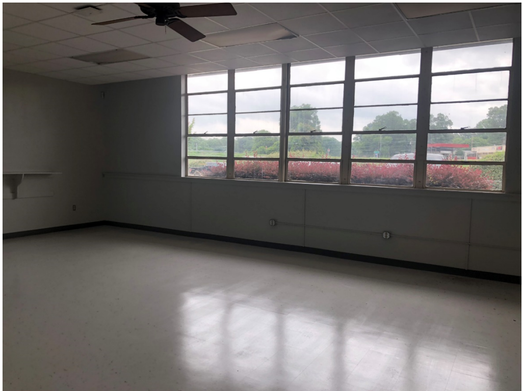
Figure 4 – South Side of South Hall Rooms Ready for Punch List
