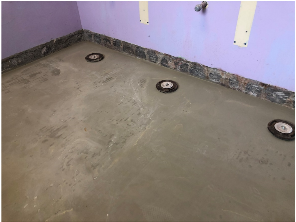
Figure 1 – South Hall Bathroom Floor Prep
