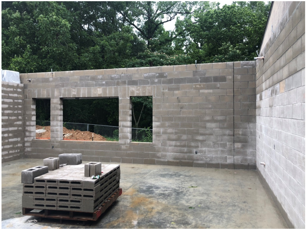
Figure 9 – Addition Interior: STEM 101
