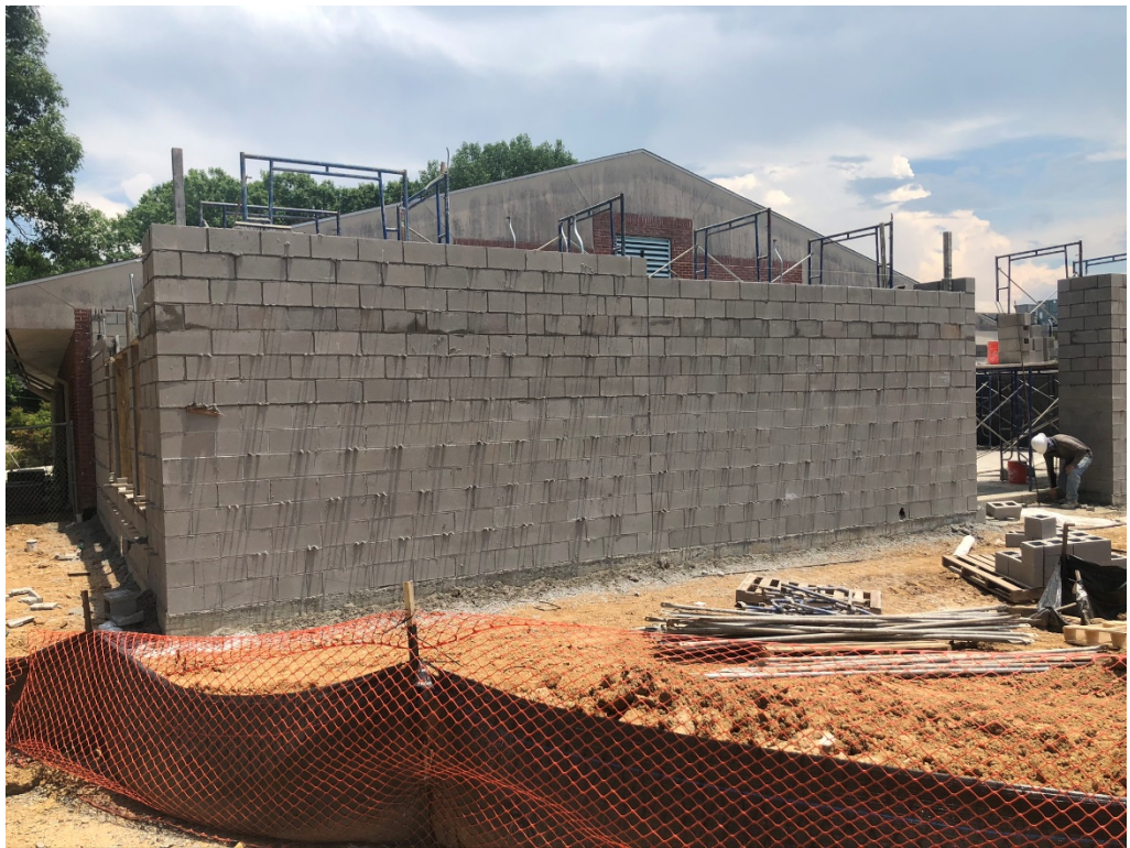
Figure 2 – NW Corner of Addition
