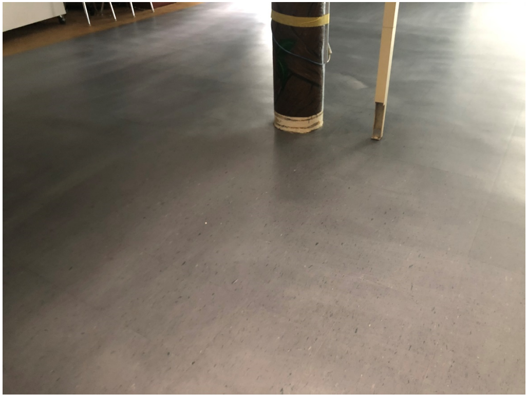
Figure 11 – VCT Install @ Library (Ongoing)
