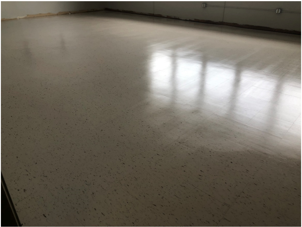
Figure 7 – New VCT Floor in South Hall Classrooms (typical)
