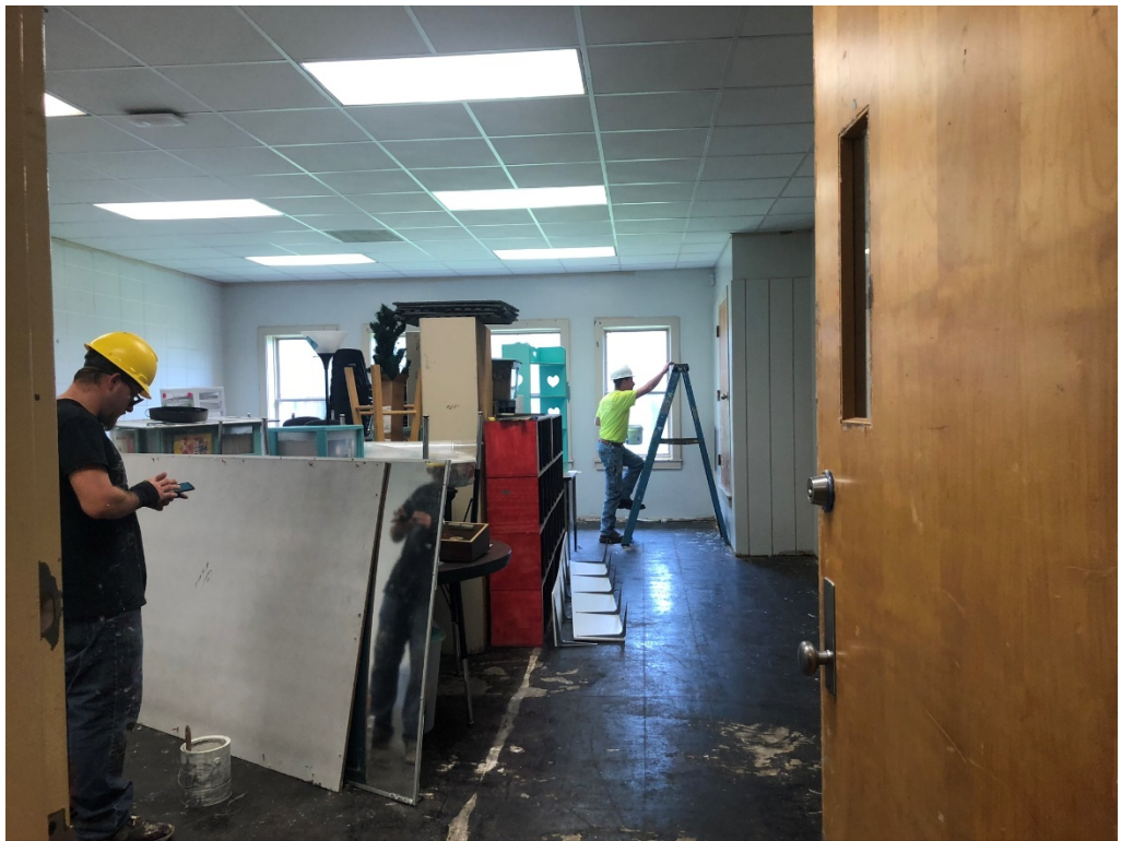
Figure 12 – Paint at North Corridor Classrooms is Ongoing
