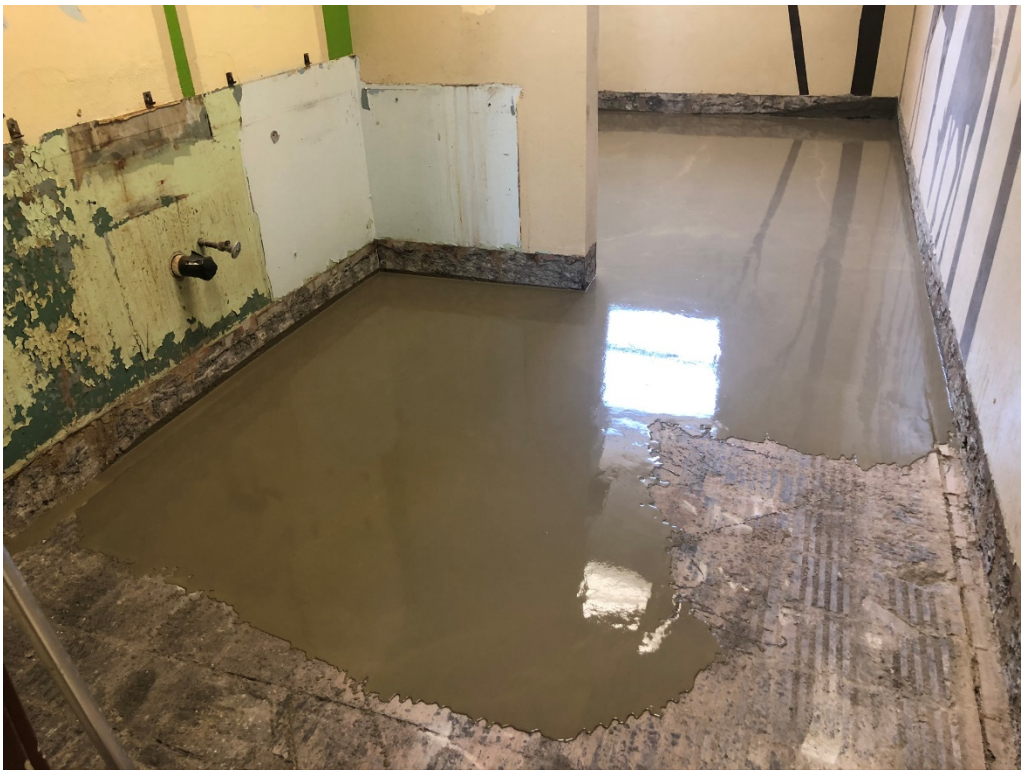
Figure 6 – Floor Leveler as Prep as Substrate for Tile
