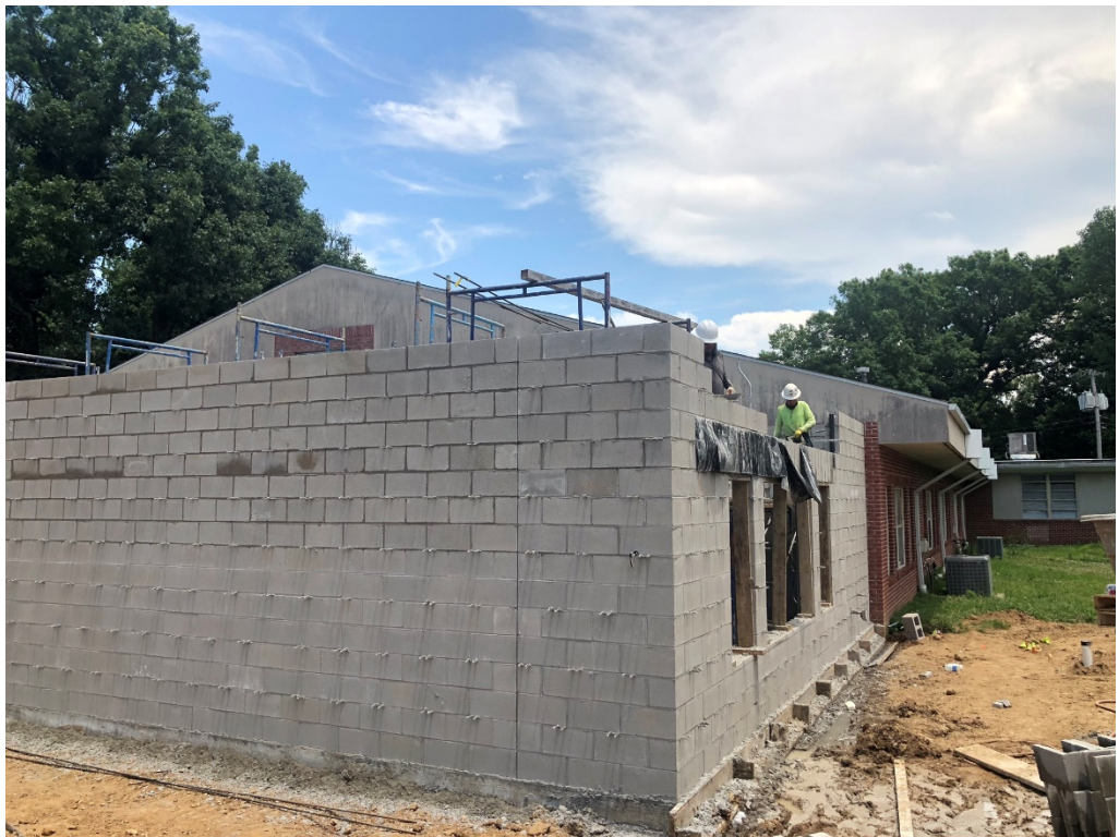
Figure 4 – SW Corner of Addition
