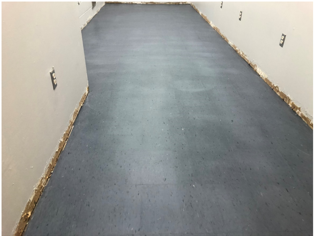
Figure 10 – VCT Install @ Counselor's Office
