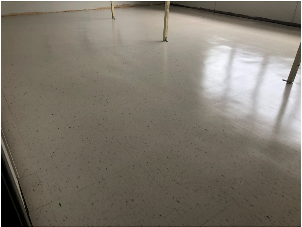
Figure 5 – New VCT Floor in South Hall Classrooms (typical)
