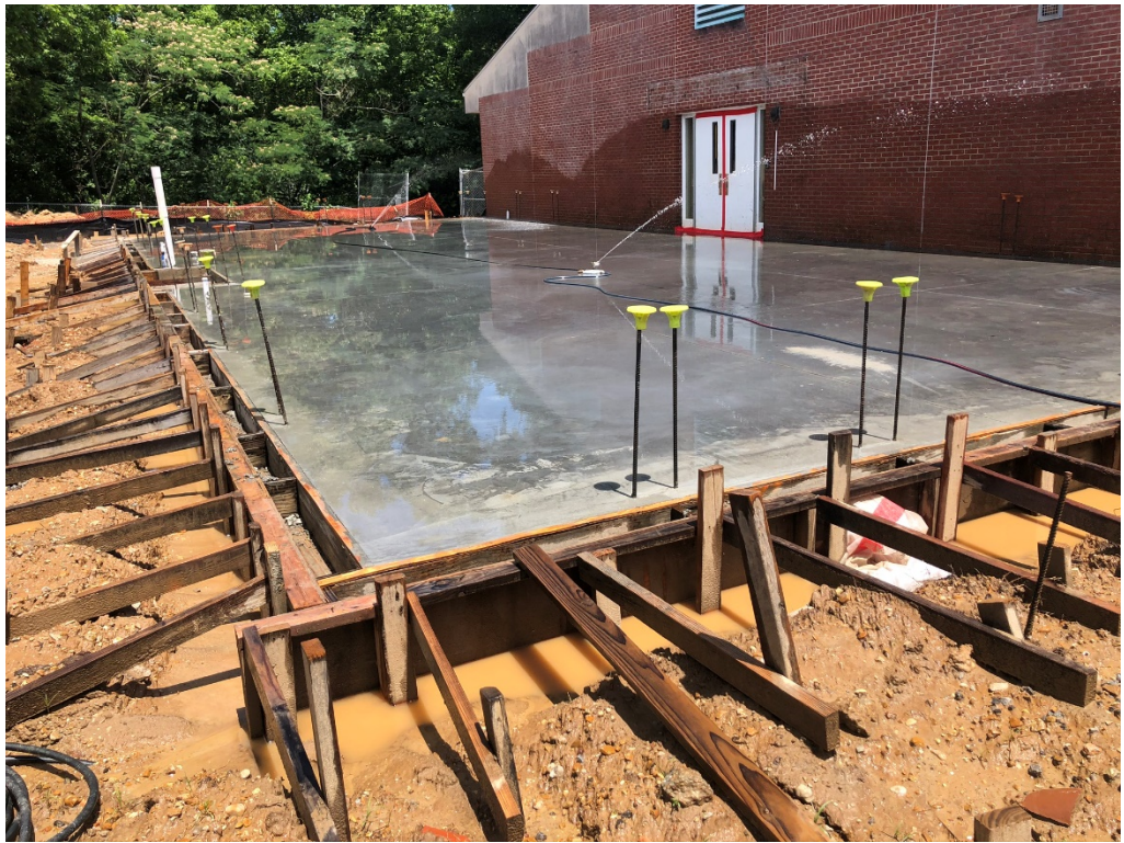
Figure 1 – Concrete Slab on its 5 th day
