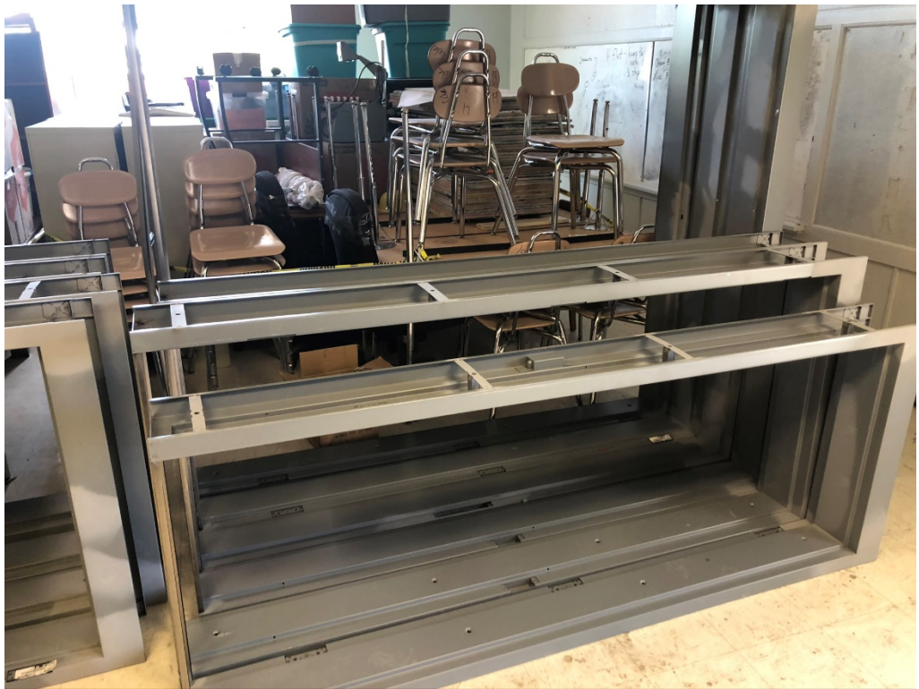
Figure 2 – HM Frames on Site
