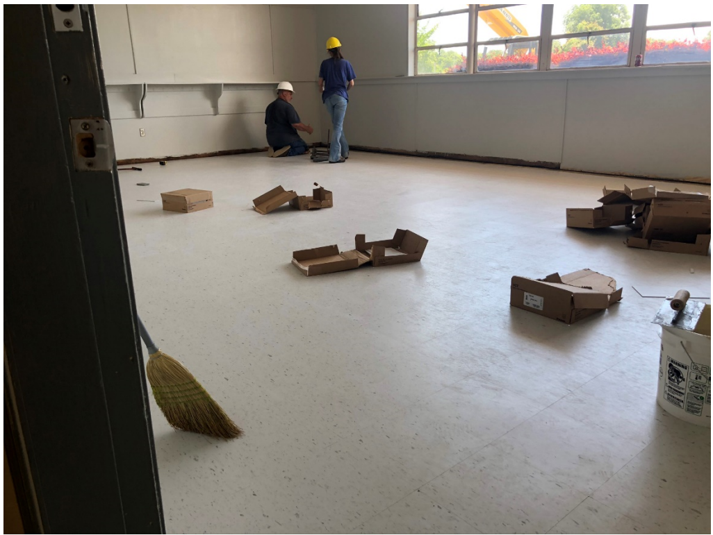
Figure 7 – Carpentry Repair at Termite Damaged Areas
