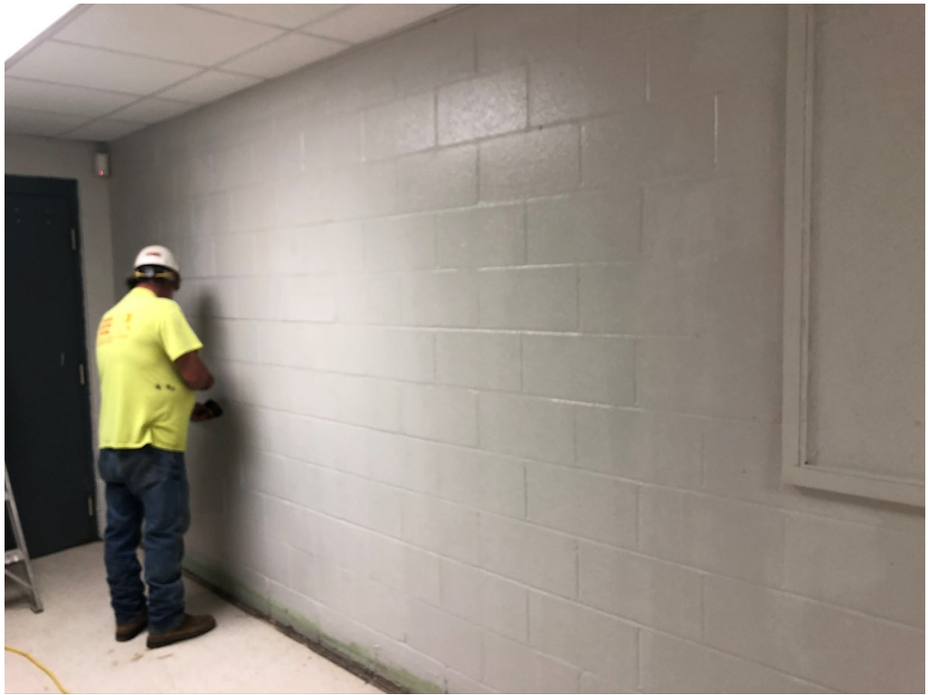
Figure 3 – Hall Side of Teacher Workroom (now used as classroom)
