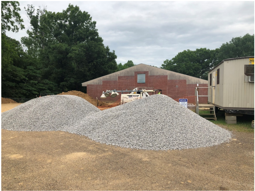
Figure 3 – Base Substrate for Foundation
