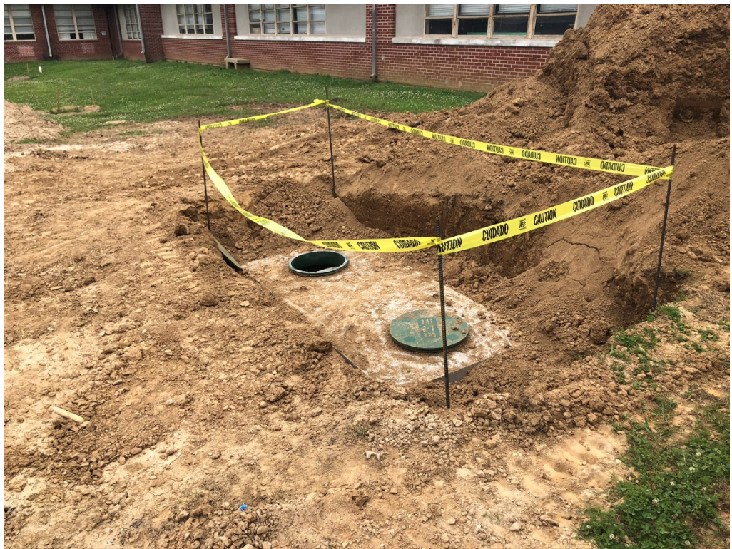
Figure 6 – New Grease Trap Installed
