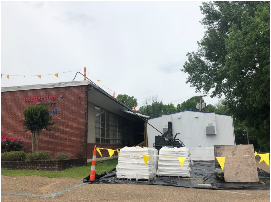
Figure 2 – Roofing Work has begun
