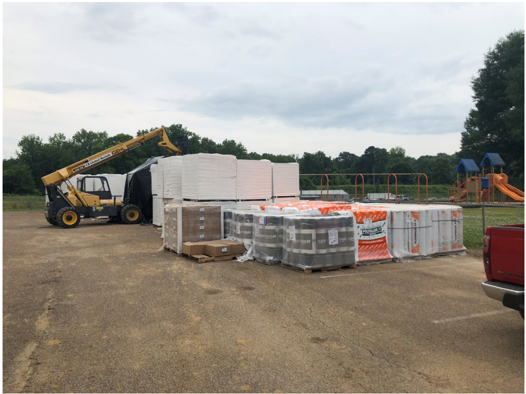
Figure 1 – Roofing Material Stored on Site
