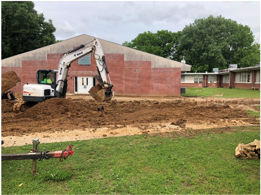
Figure 1 – North Addition Dirt Work
