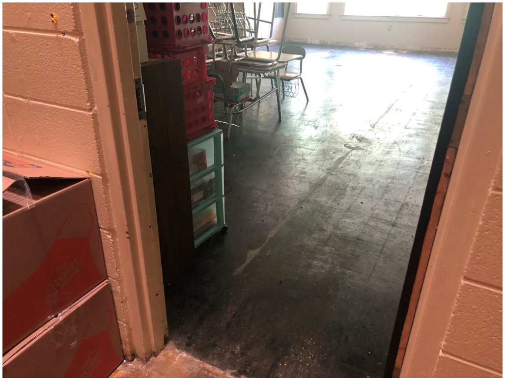
Figure 8 – North Hall Demo Complete (typical class)
