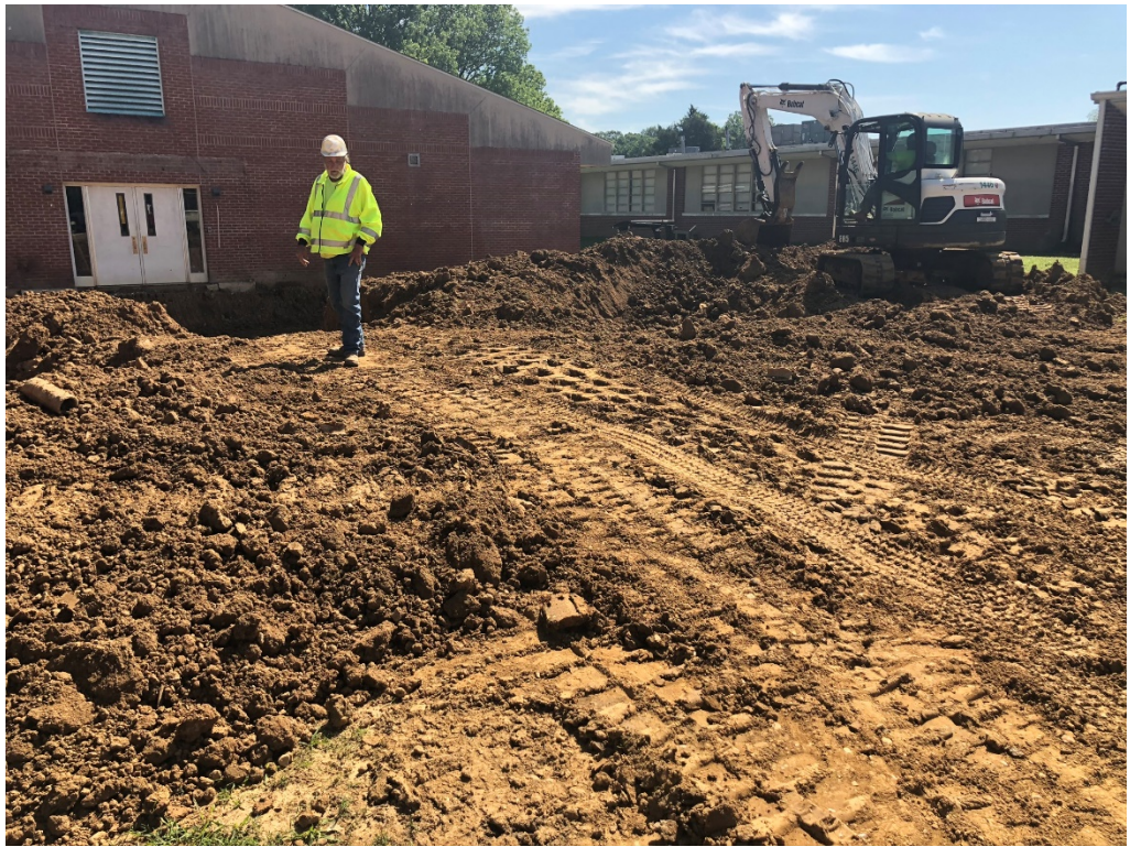
Figure 1 – North Addition Dirt Work
