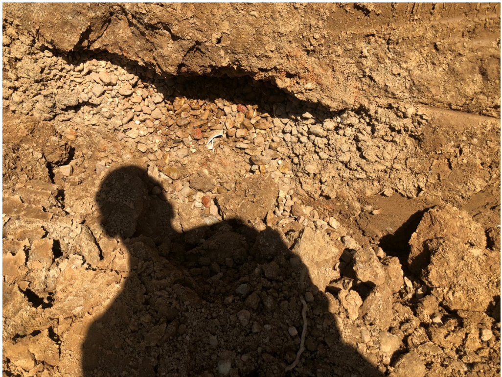
Figure 2 – Drain at Extent of Project Bounds
