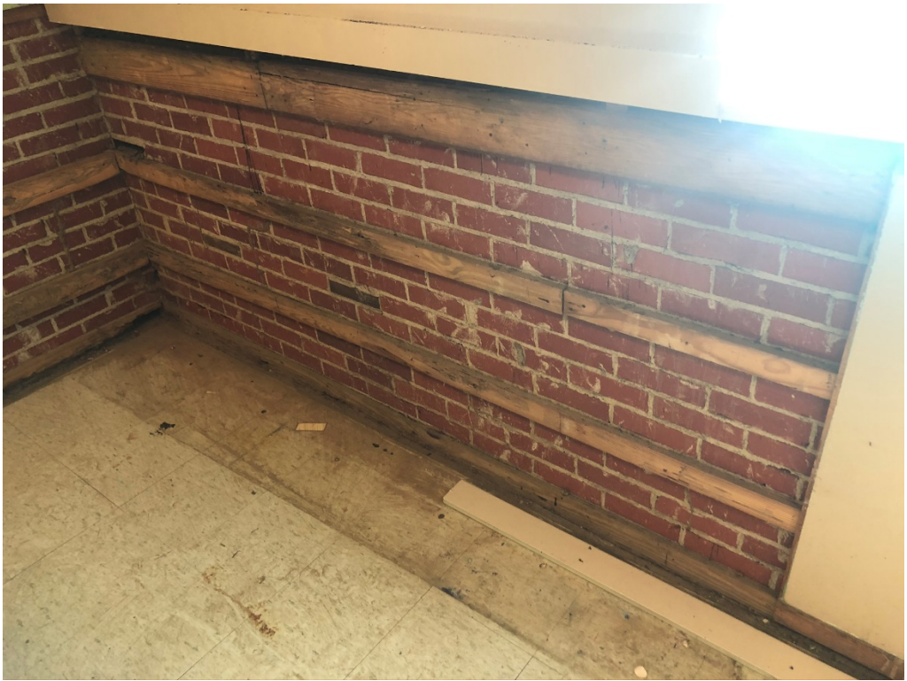
Figure 5 – Southern Wall Paneling Removed @ Classroom 4
