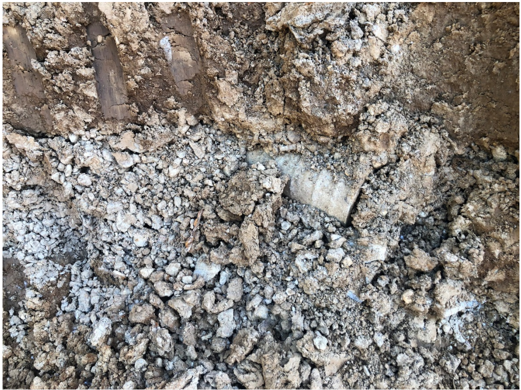
Figure 3 – Drain that Moves Below Building Footing
