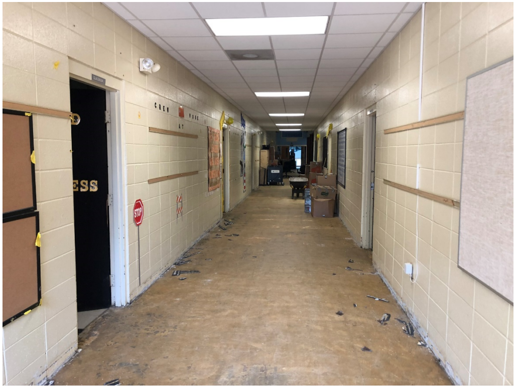
Figure 1 – North Hallway Floor Demo
