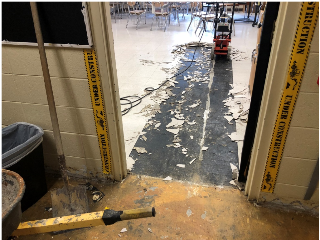
Figure 2 – North Hall Classrooms Demo Begun
