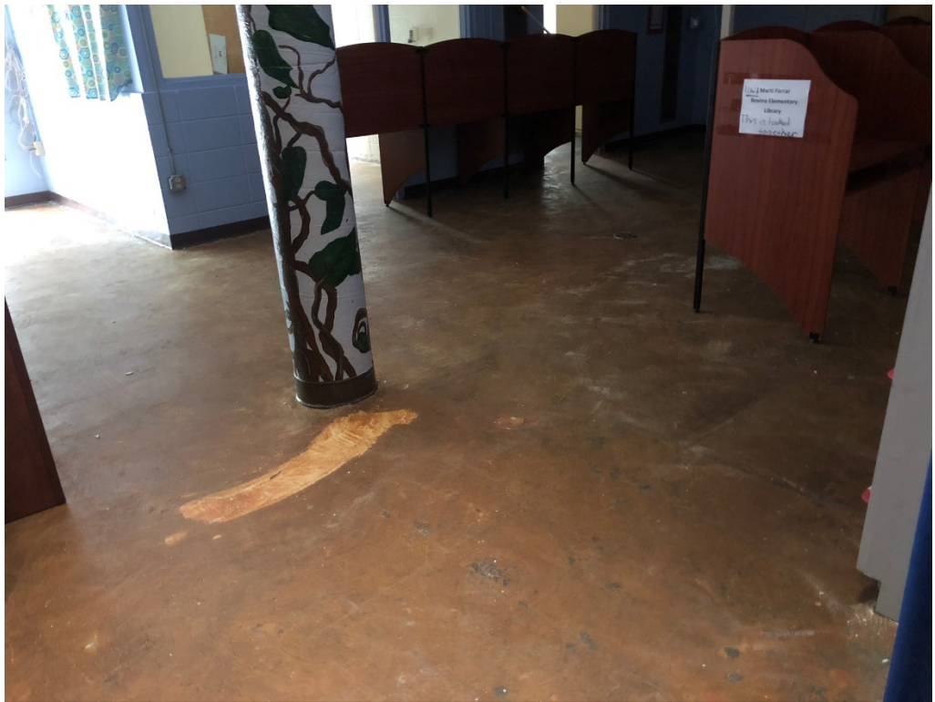
Figure 4 – Library Floor Demo Complete
