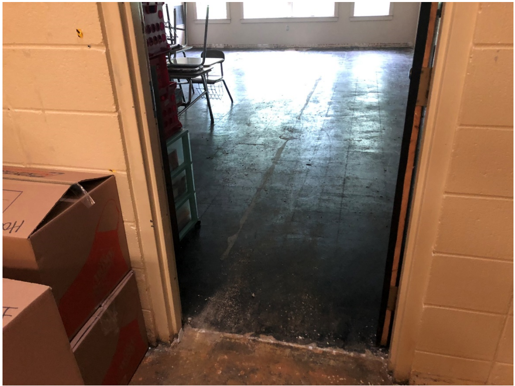
Figure 3 – Some Classrooms Complete
