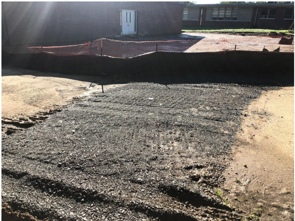
Figure 2 – Drainage Compacted and base installed
