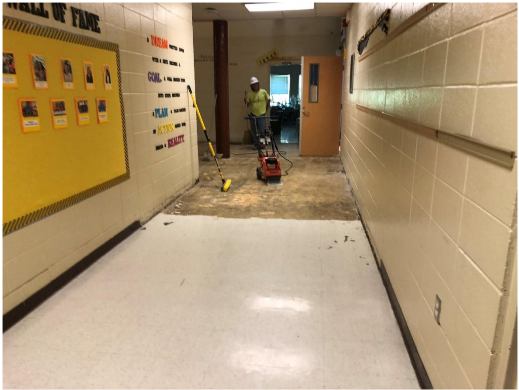
Figure 5 – East Hall floor Progress
