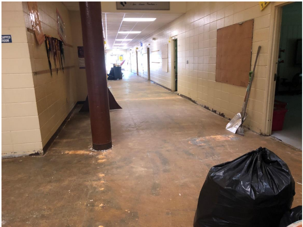
Figure 6 – North Hall demo
