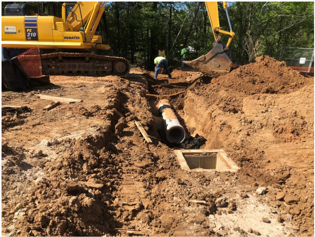
Figure 1 – Storm Drainage Covered (from March 26)
