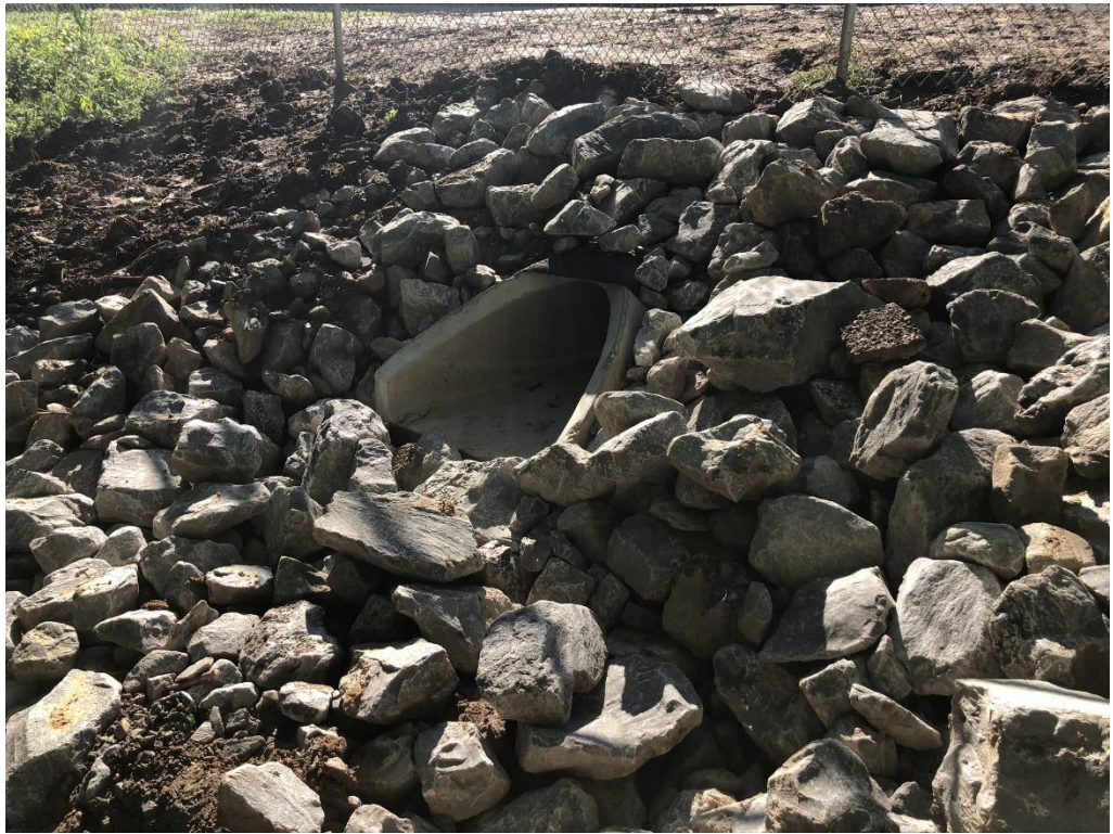
Figure 3 – Rip Rap and discharge complete
