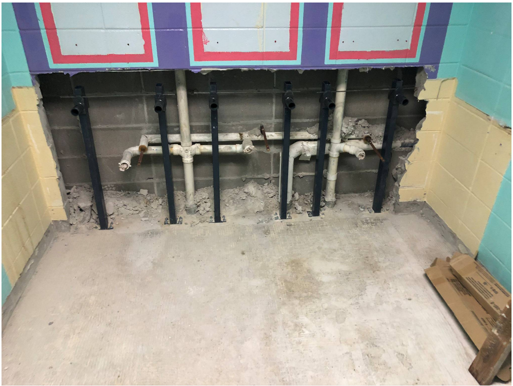
Figure 5 – Plumbing Rough In
