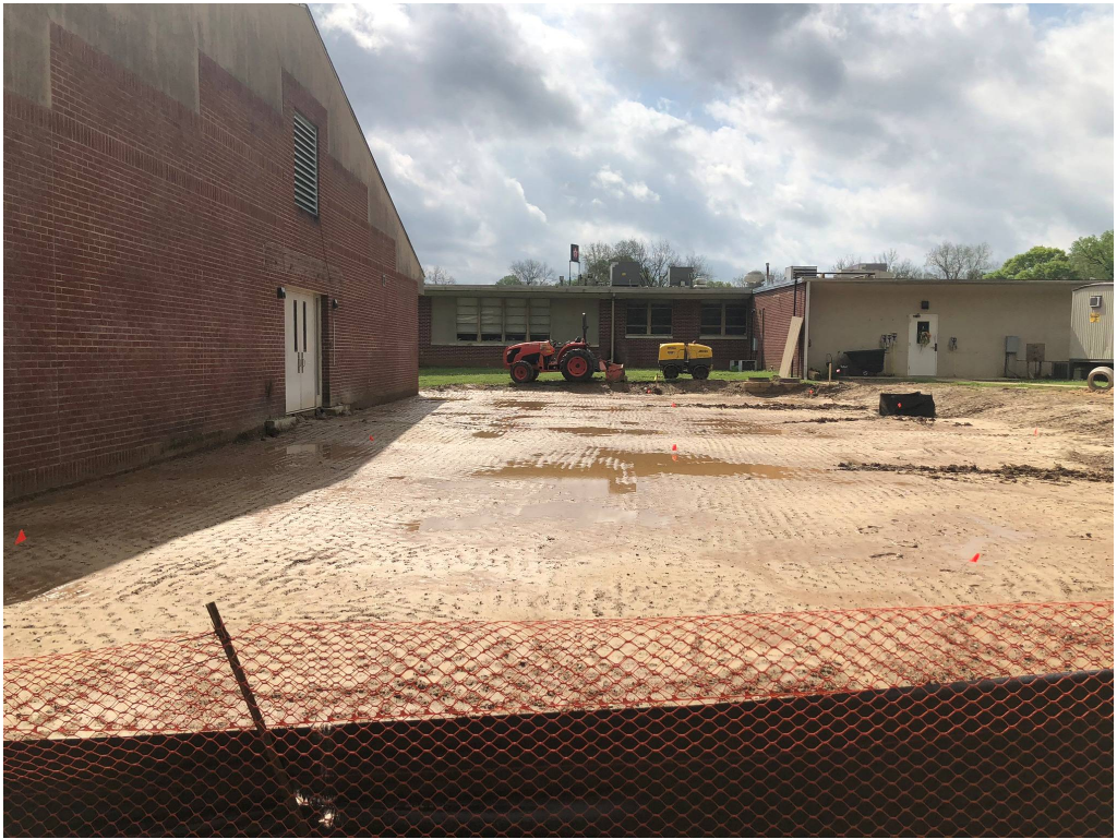
Figure 1 – Pad Development at Addition
