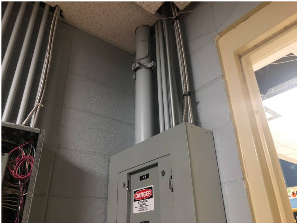
Figure 24 – Electrical Panel Work
