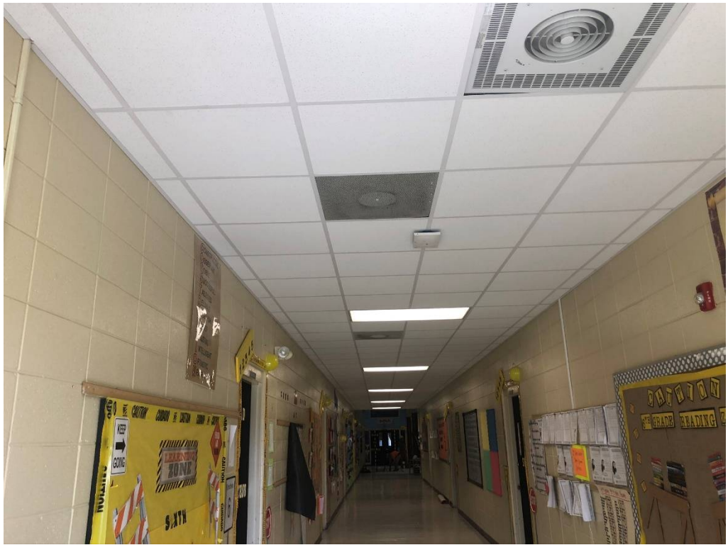
Figure 3 – North Hall Ceiling Grid Complete
