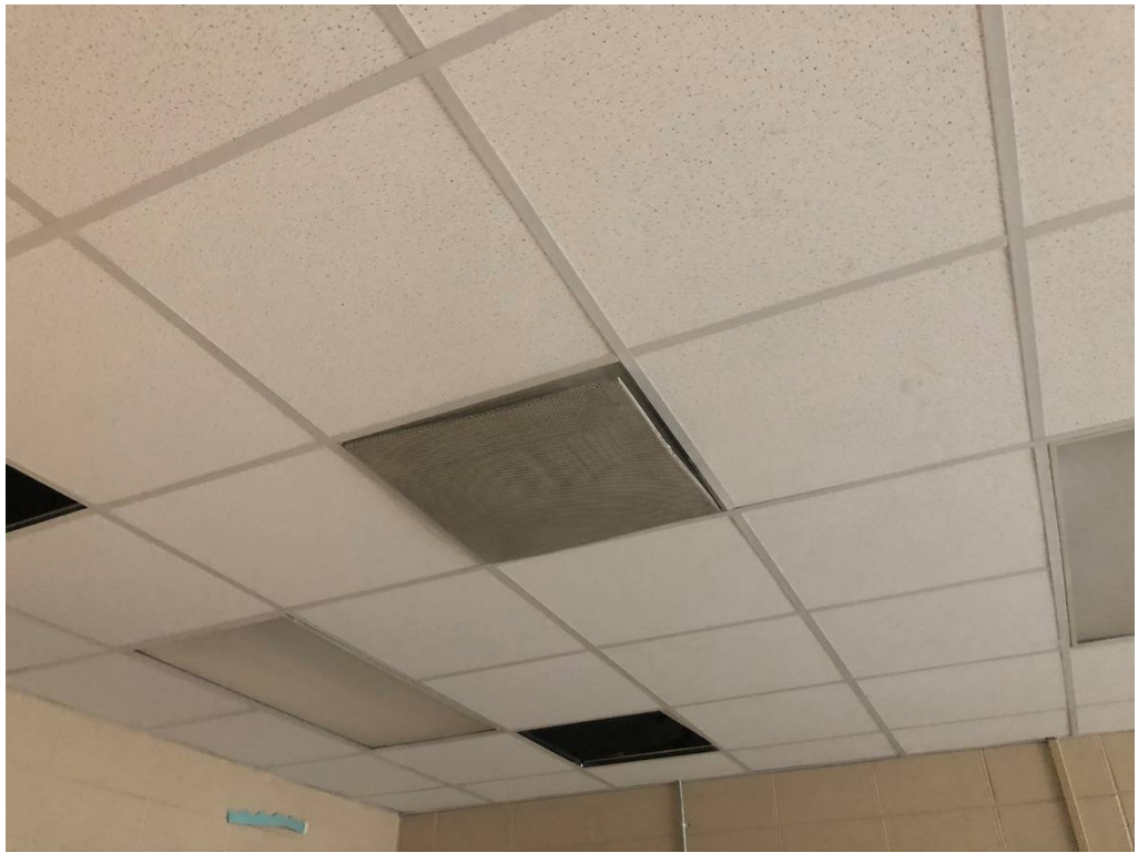
Figure 5 – Hanging Vent Cover (Classroom 7 in North Hall as noted by Sign Above Door)
