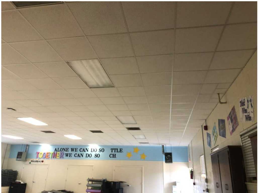
Figure 18 – Auditorium New Ceiling
