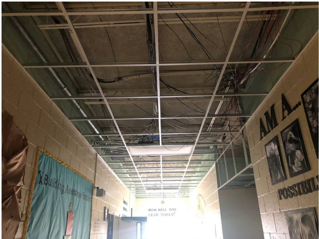
Figure 16 – South Entry Hall
