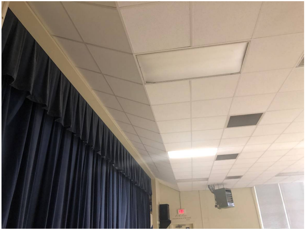
Figure 17 – Auditorium New Ceiling
