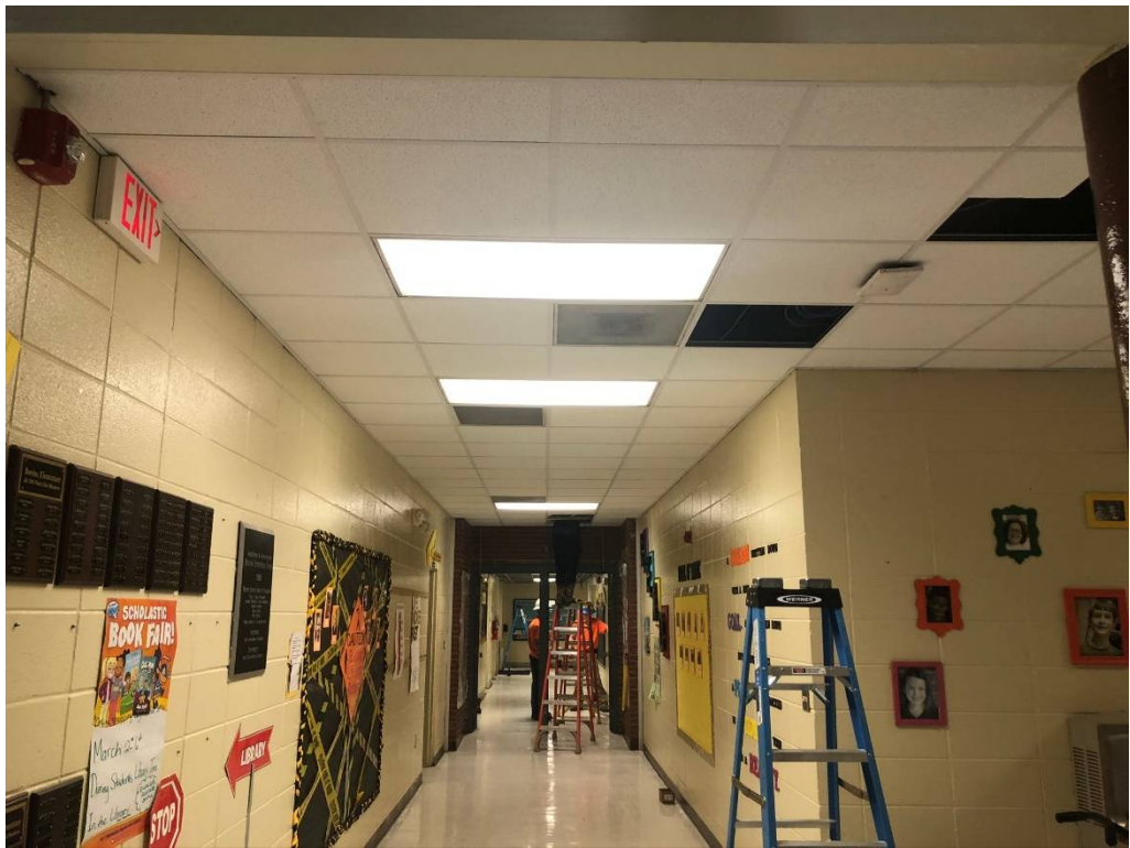
Figure 8 – North Hall Looking South from Classroom 15 Entry
