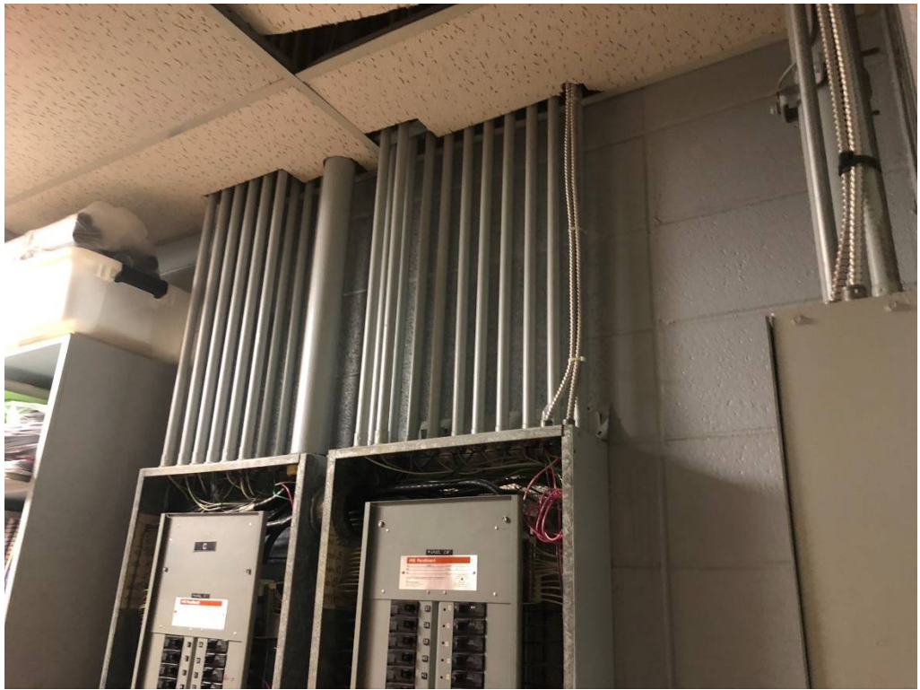
Figure 23 – Electrical Panel Work
