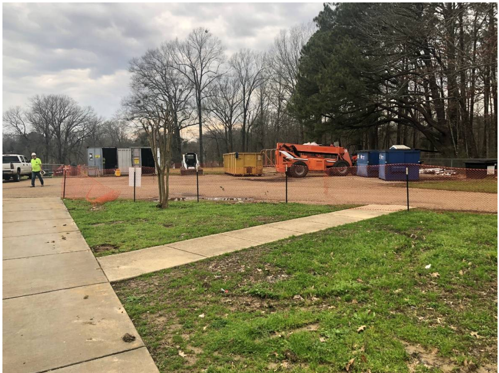
Figure 18 – Construction Trailer & Staging at North West Section of Site
