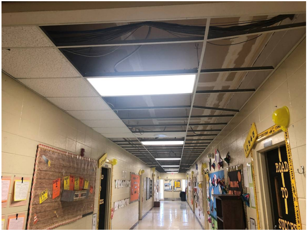
Figure 17 – North Corridor Partial Demo
