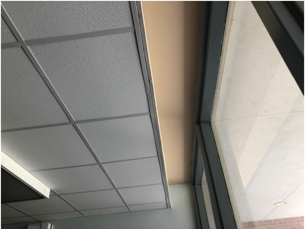
Figure 14 – Missing Paint
