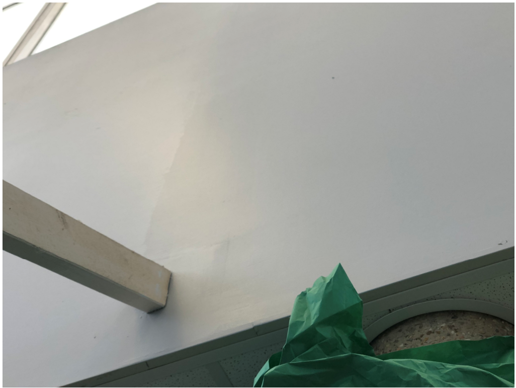
Figure 17 – Uneven/unmatching paint
