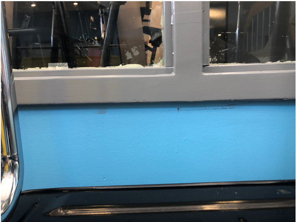
Figure 8 – General Paint Touchups throughout
