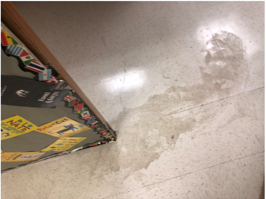
Figure 20 – Dirt Collected at Unwaxed/reworked Tiles
