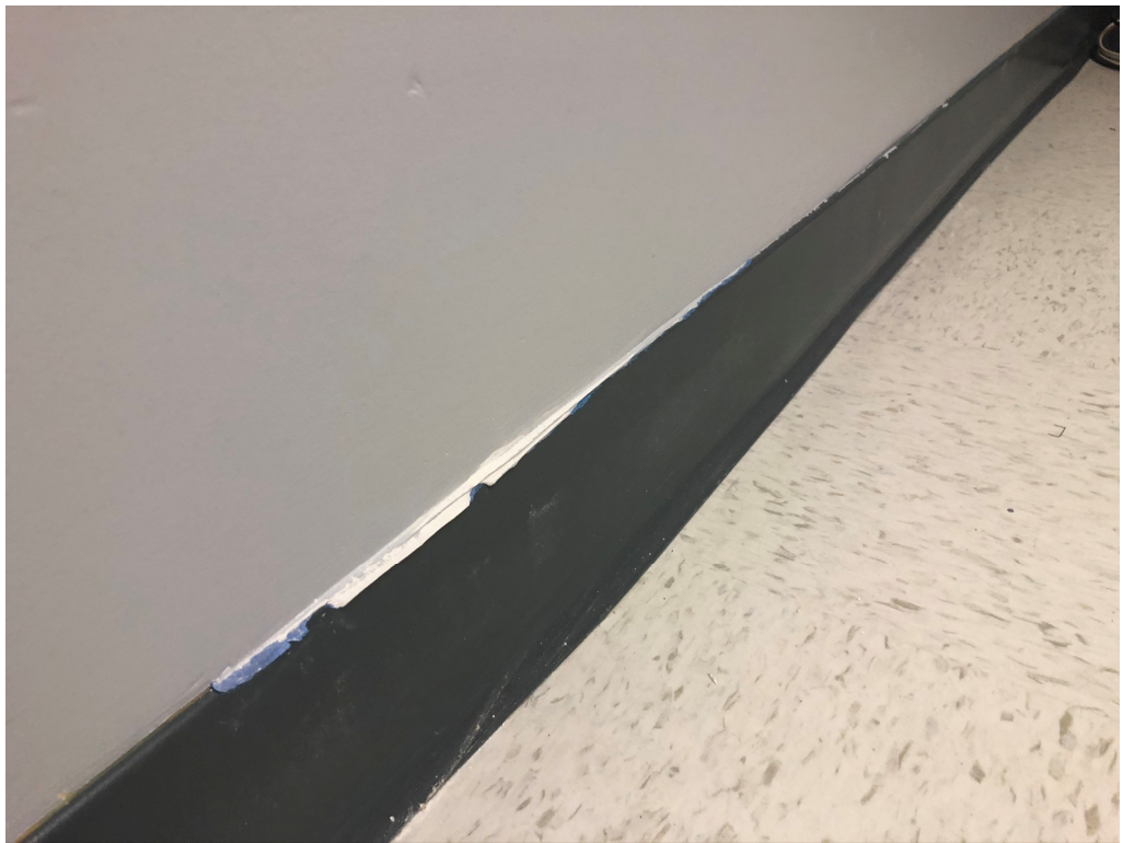
Figure 24 – Base with Tape Still Adhered
