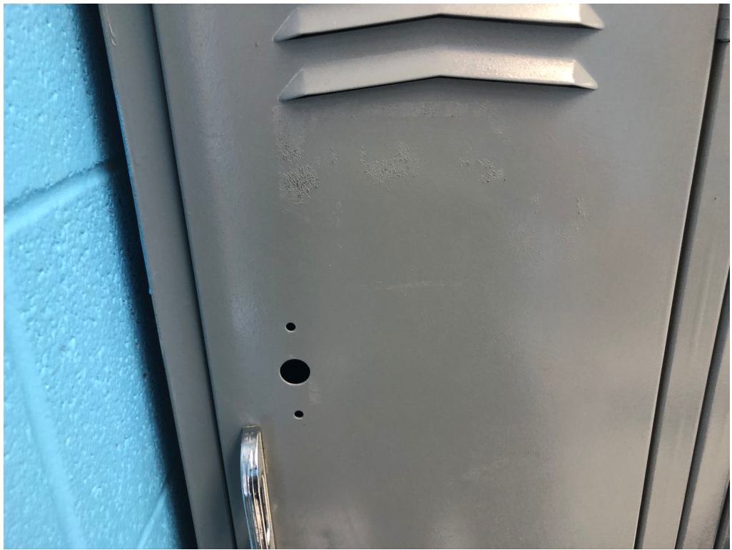
Figure 3 – Rough surfaces at lockers that should be prepped more thoroughly
