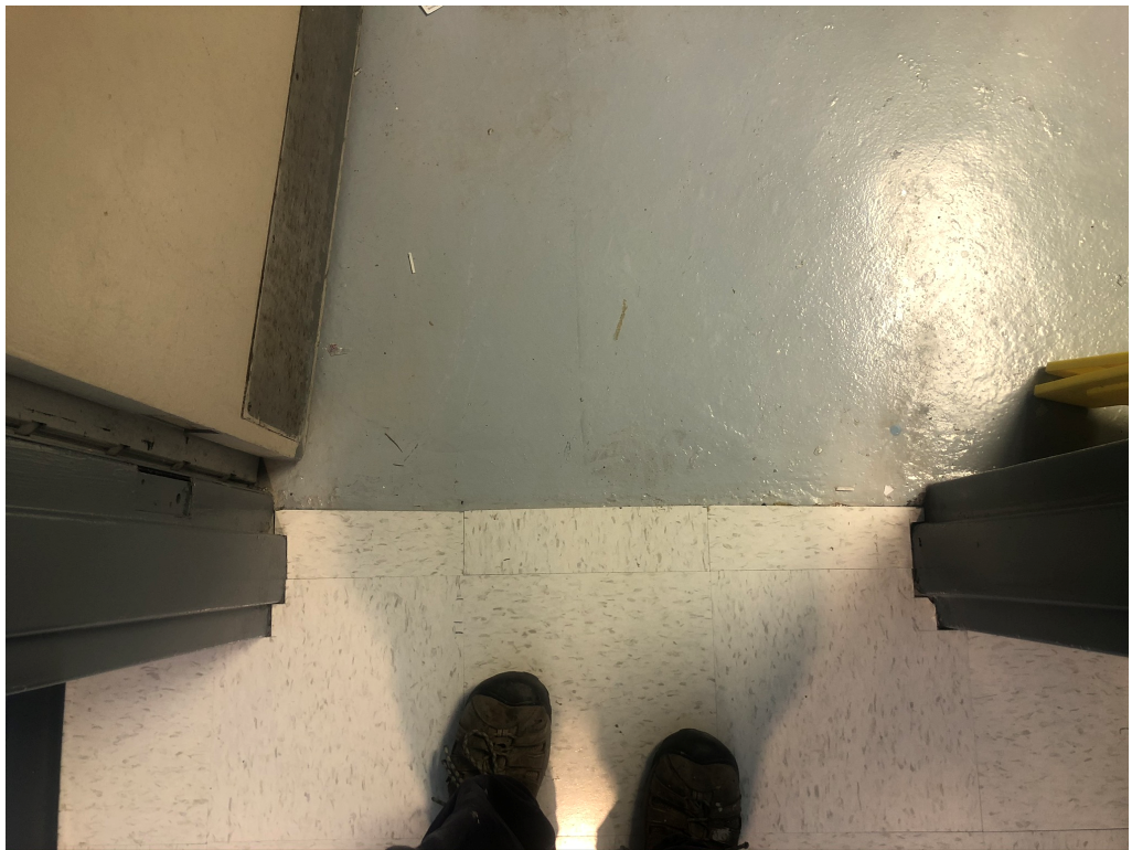
Figure 10 – Rubber Threshold Required at Unfinished VCT Edges in Doorways
