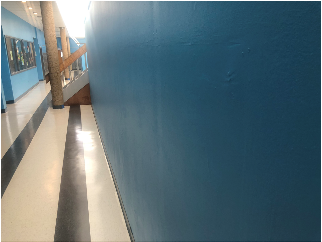
Figure 3 – Wall Prep still needed at this wall
