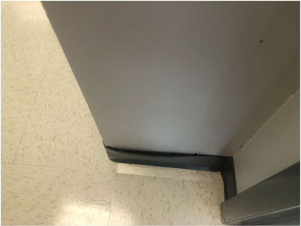
Figure 11 – Rubber Base Lacking adhesion
