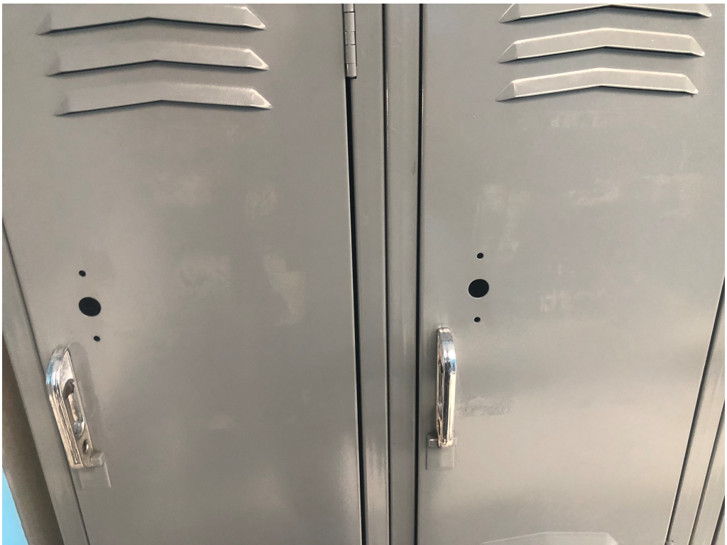
Figure 4 – Some Locker Finishes are uneven
