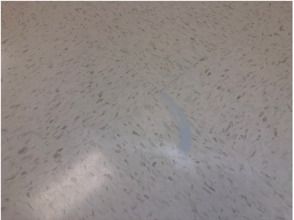
Figure 8 – Paint Under Floor Wax
