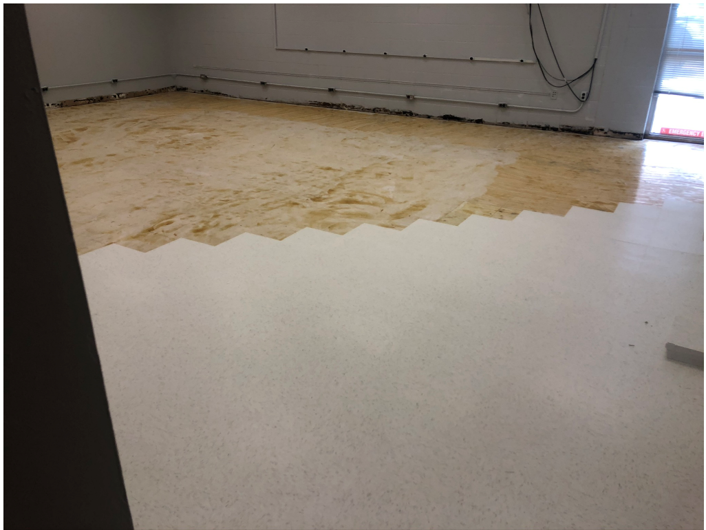
Figure 2 – Northwest Classroom in Building 100
