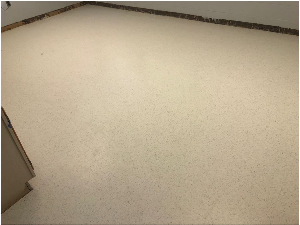
Figure 11 – VCT at South Classrooms in Building 100
