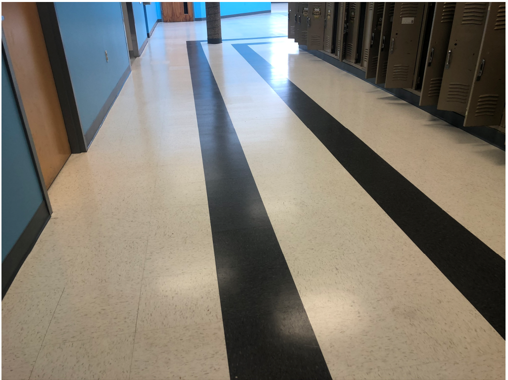
Figure 18 – Building 300 Wax is Ongoing
