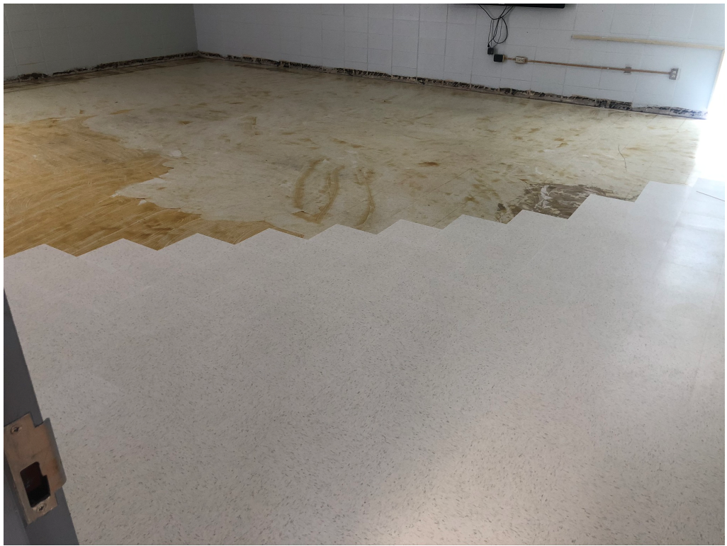
Figure 3 – Northwest Classroom in Building 100
