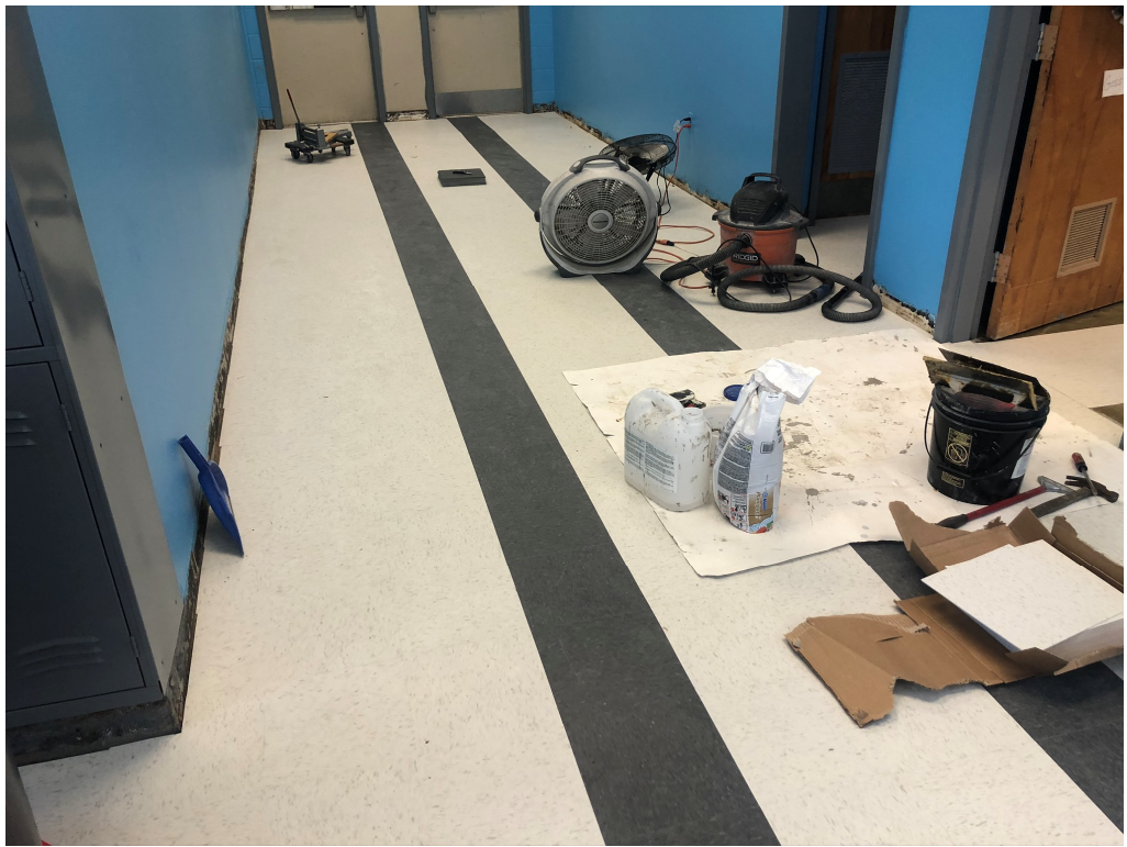
Figure 9 – VCT in Corridor
