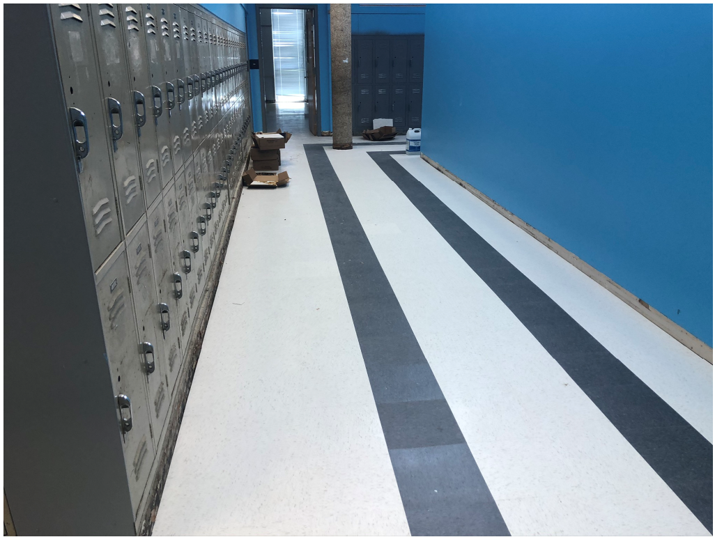
Figure 1 – VCT in Building 100
