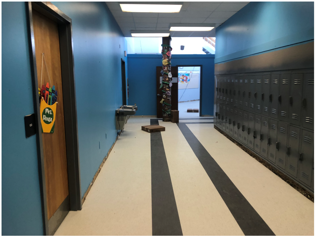
Figure 15 – VCT at Building 100
