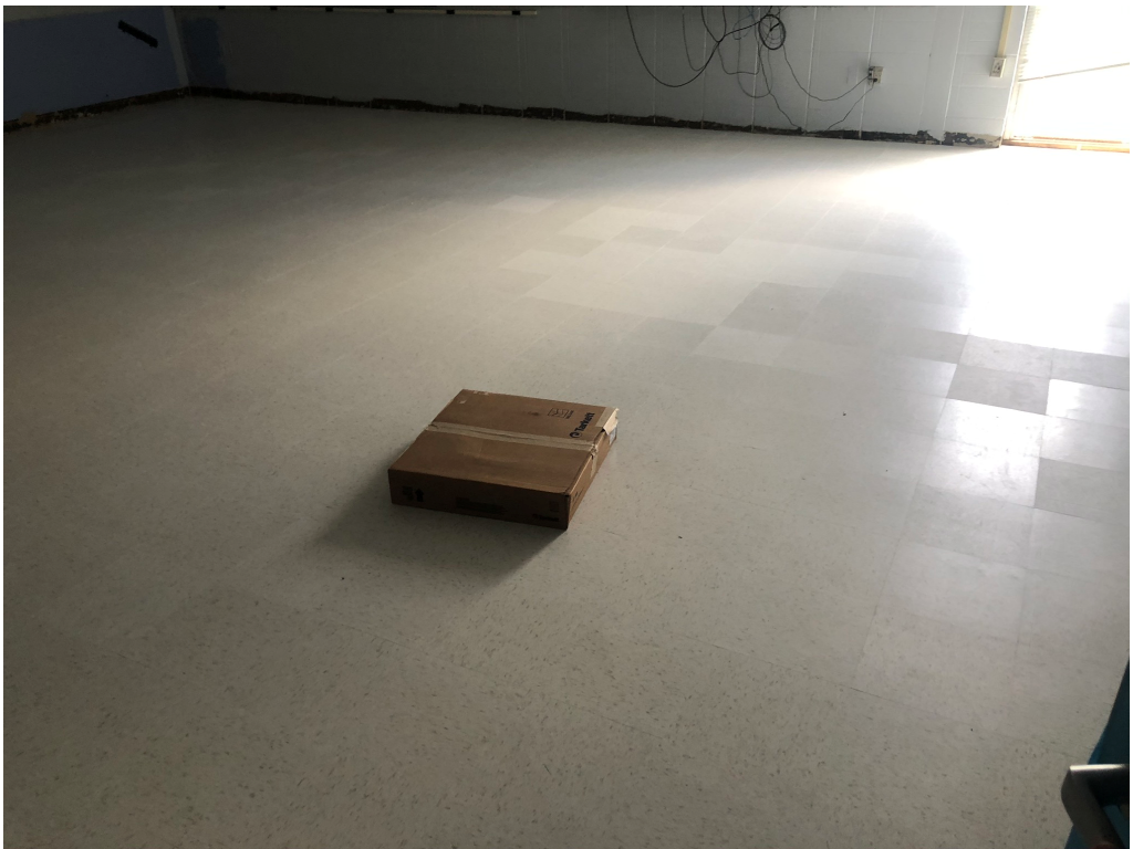
Figure 12 – VCT at South Classrooms in Building 100
