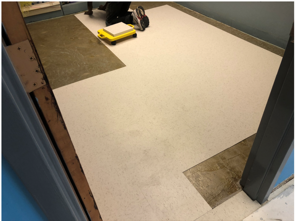
Figure 10 – VCT at Building 100 Work Room
