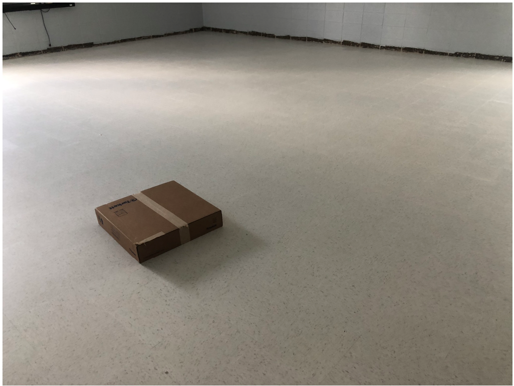
Figure 13 – VCT at South Classrooms in Building 100
