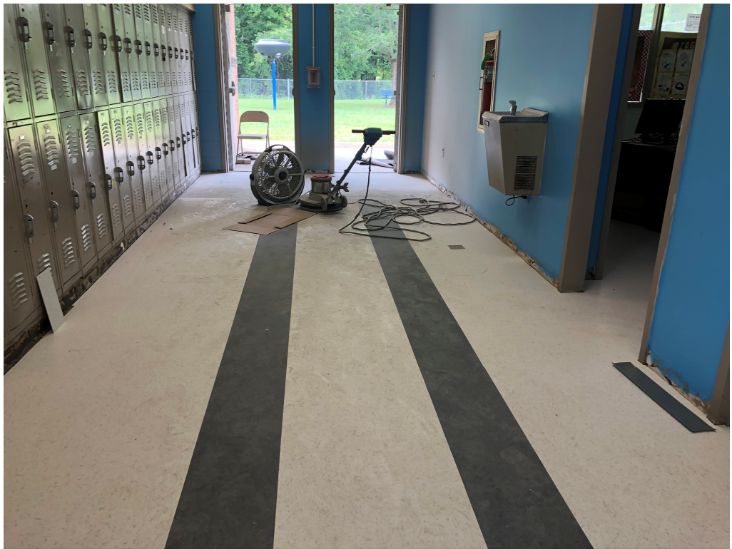
Figure 8 – Corridor Flooring in Building 300 is Ongoing
