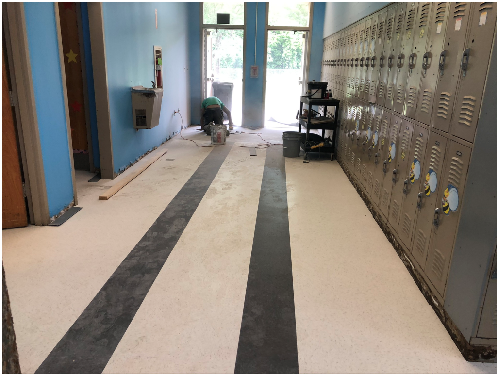
Figure 7 – Corridor Flooring in Building 300 is Ongoing
