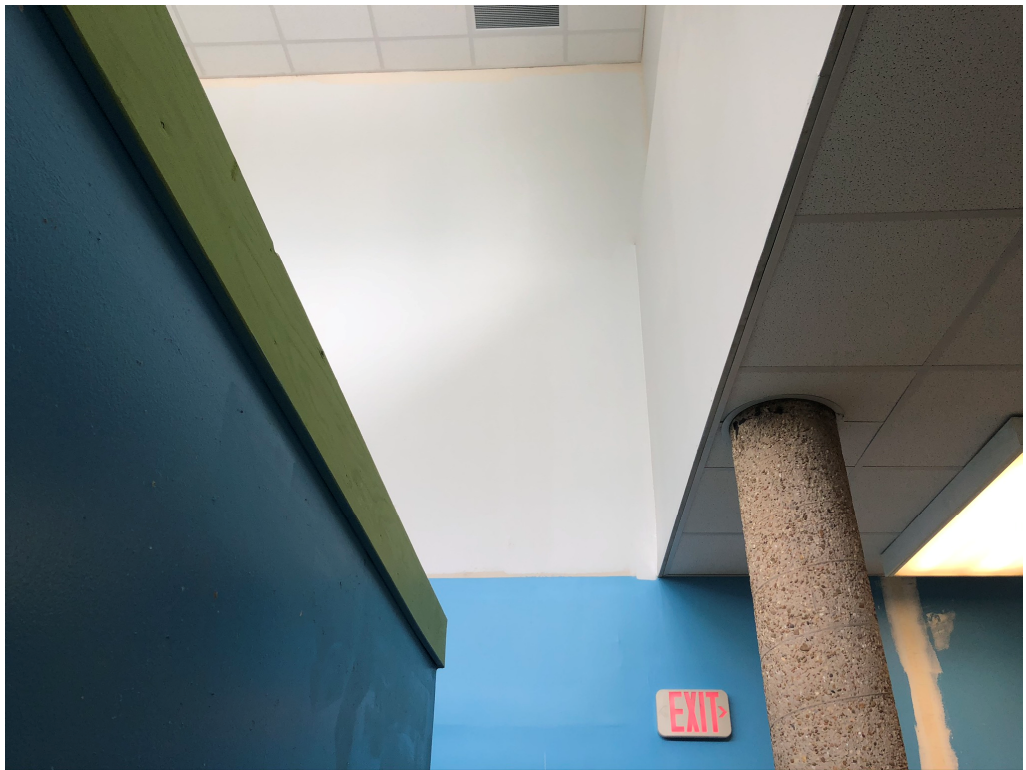
Figure 2 – Paint Work in Main Corridor Space for Building 100
