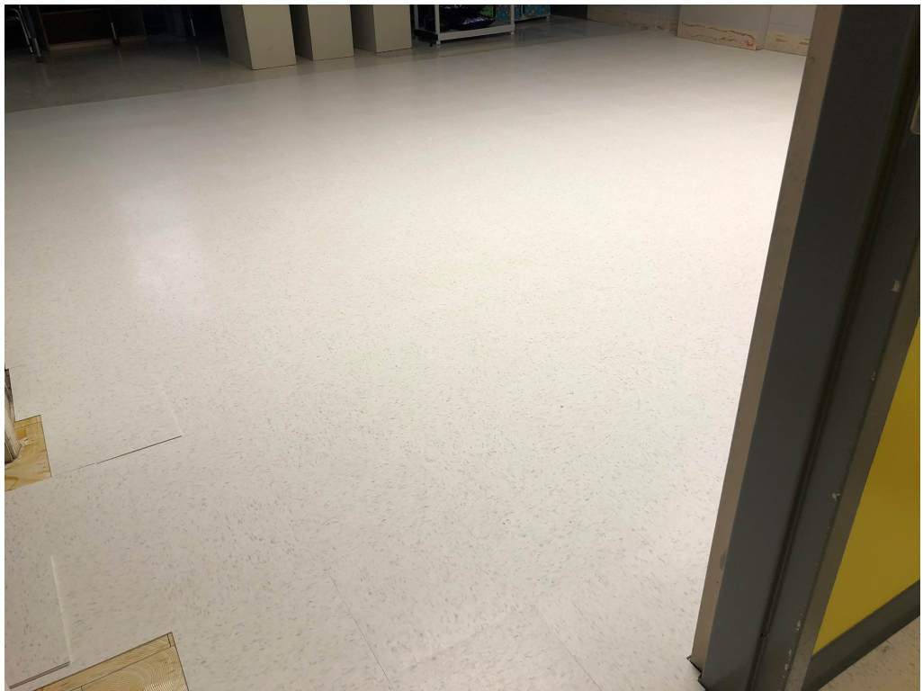
Figure 4 – Floor Installation at Building 200
