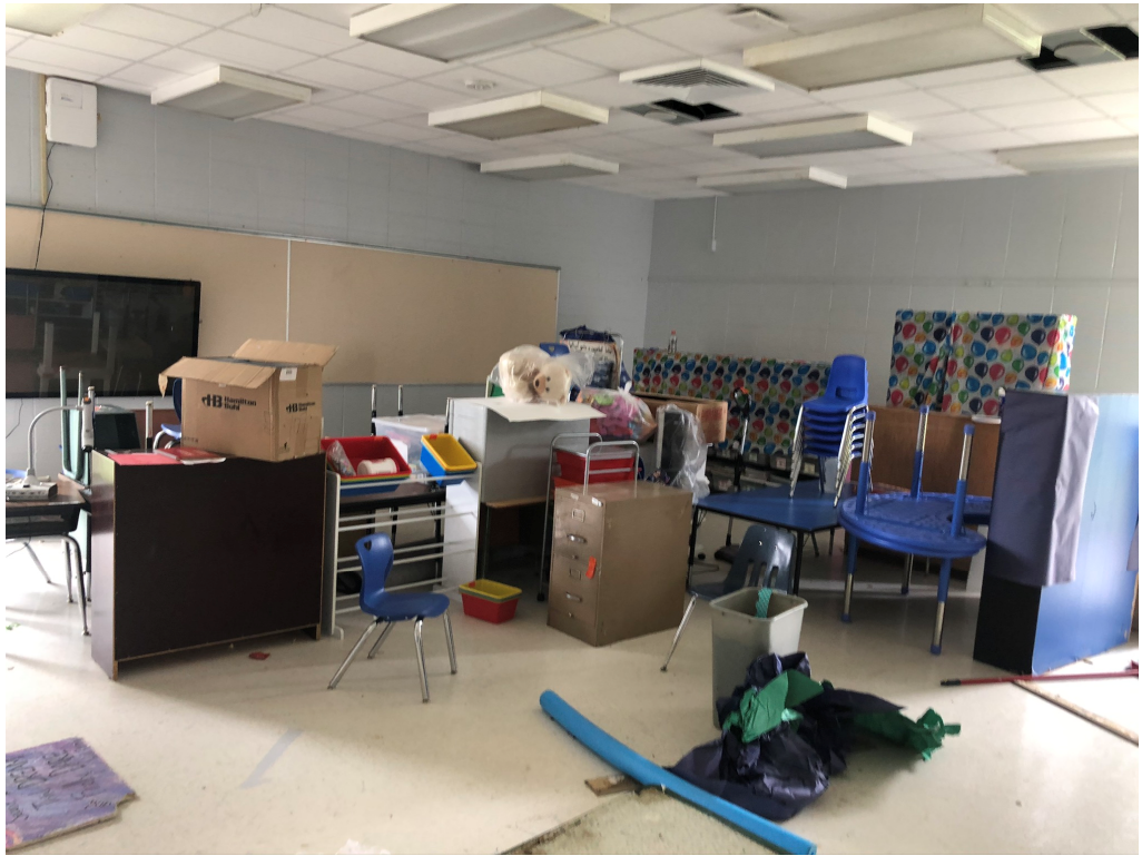
Figure 1 – Paint is Ongoing in Building 100
