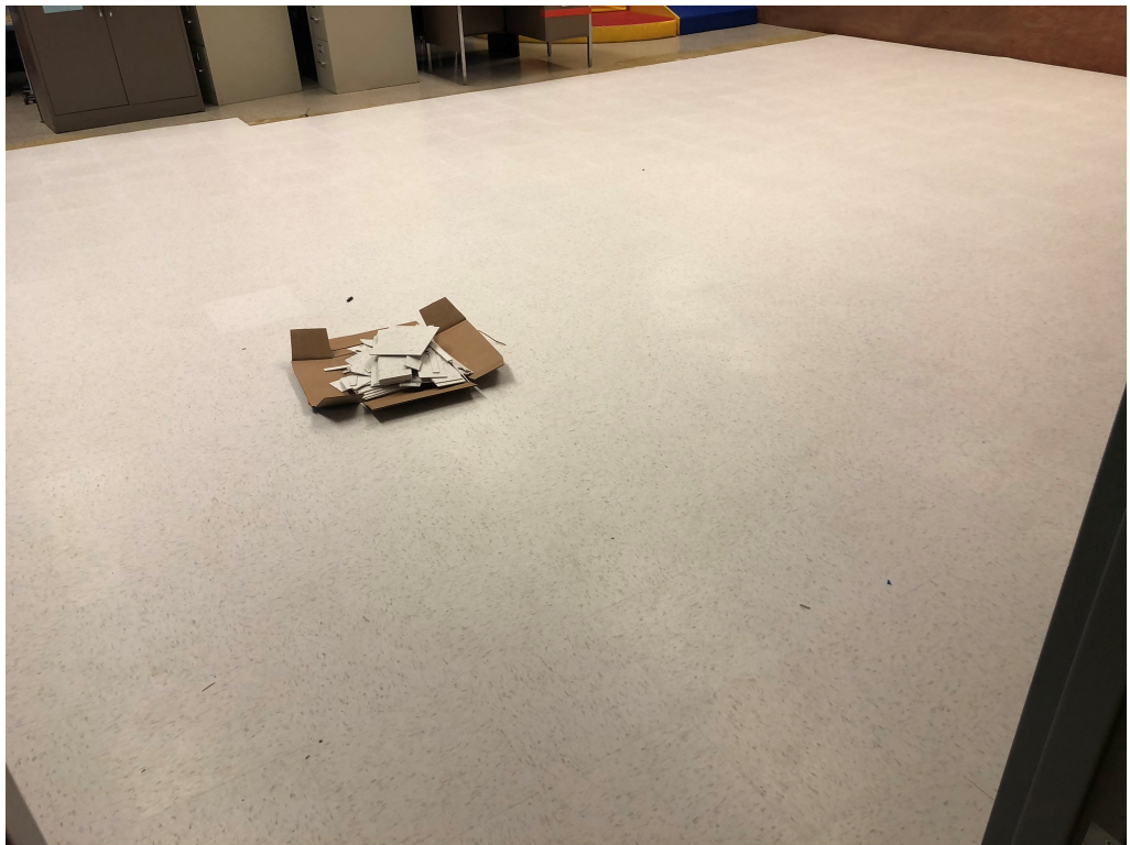
Figure 6 – Contractor Taking Care to Work around School Property
