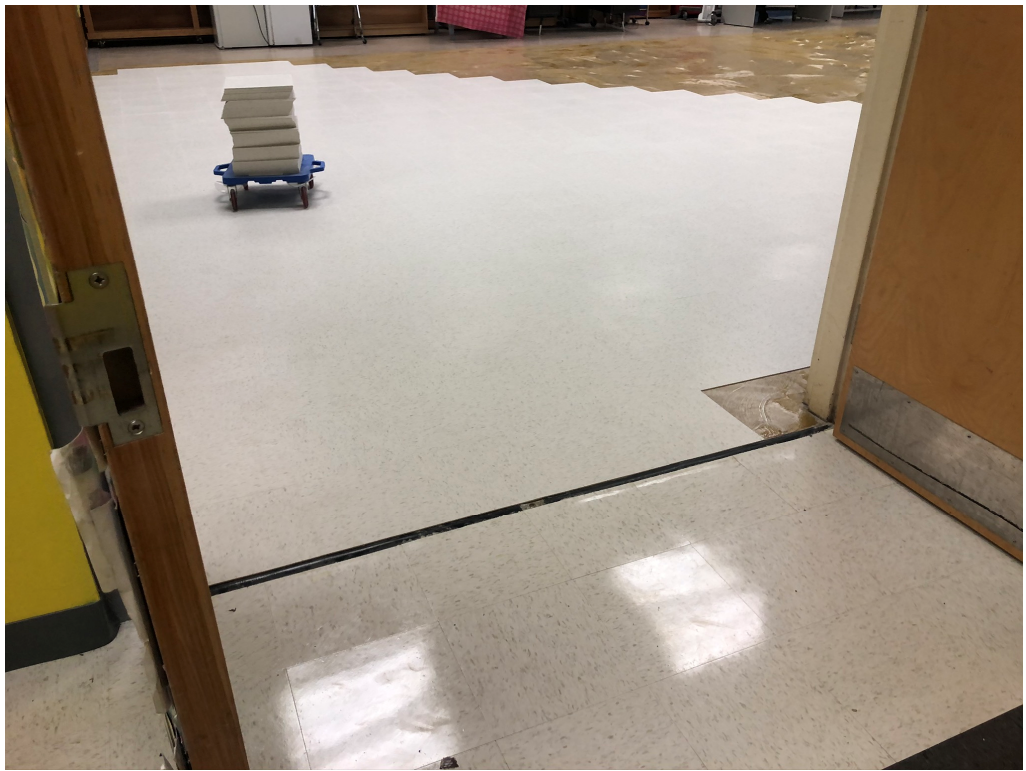
Figure 5 – Floor Installation at Building 200 in Library
