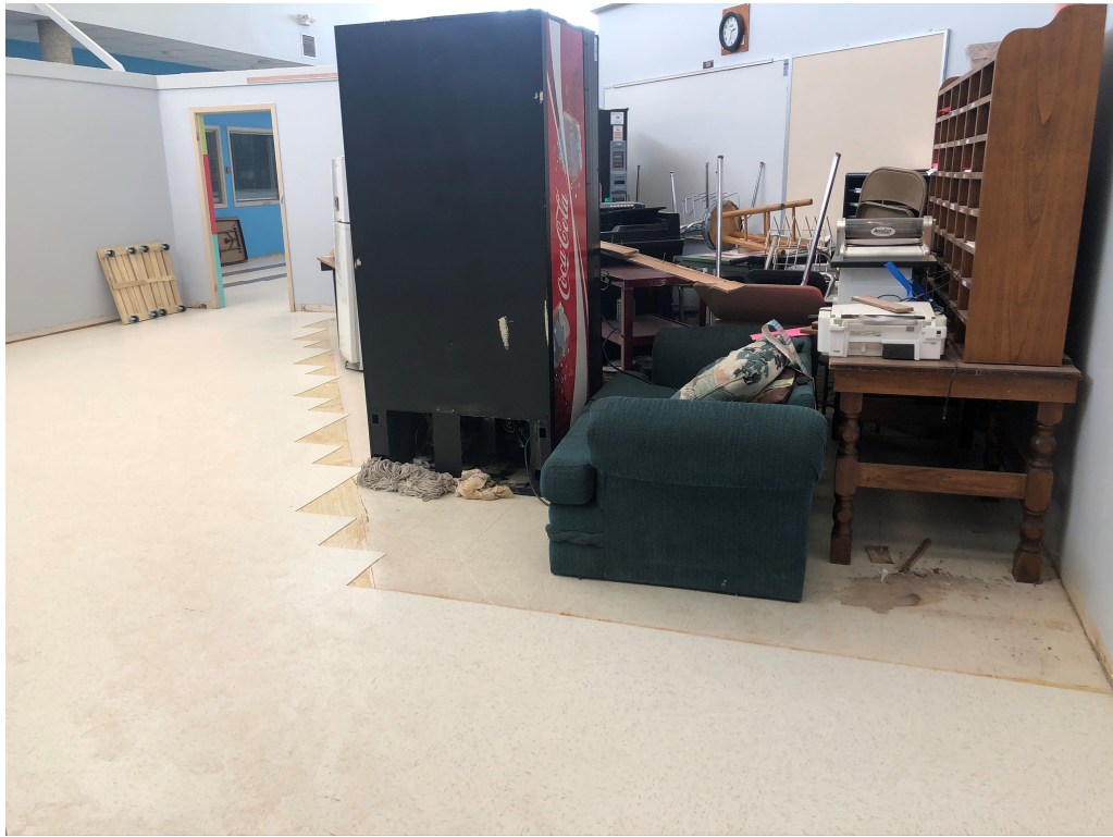
Figure 5 – Contractor Making an Effort to work around School Property
