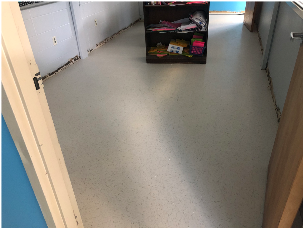
Figure 2 – Flooring Installation at 300 Wing is Ongoing
