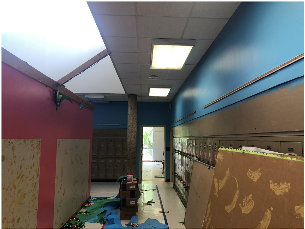
Figure 7 – Paint work is Ongoing in 100 Wing
