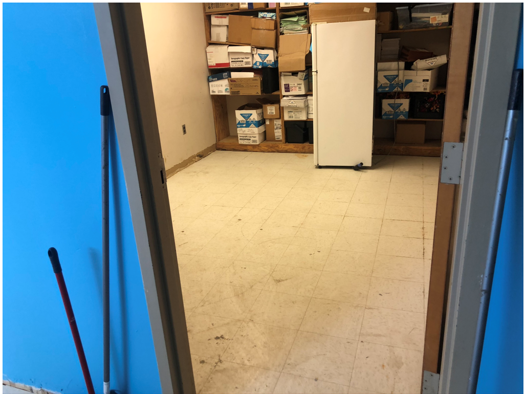
Figure 4 – Floor Prep is Ongoing in 300 Wing Also
