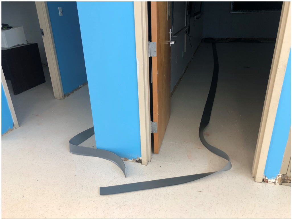
Figure 1 – Base Installation Ongoing in 300 Building
