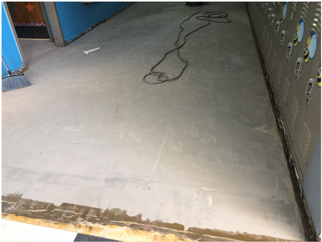
Figure 3 – Prep at Entry Vestibules in 300 Building
