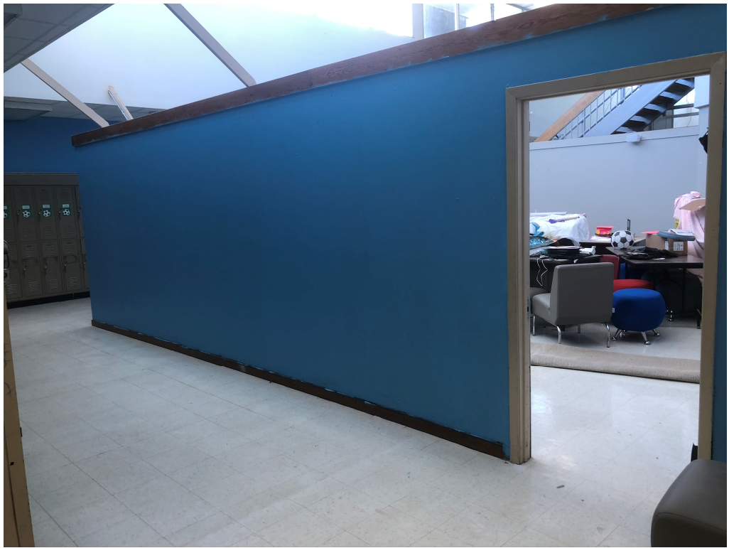
Figure 1 – Building 3 Paint Ongoing
