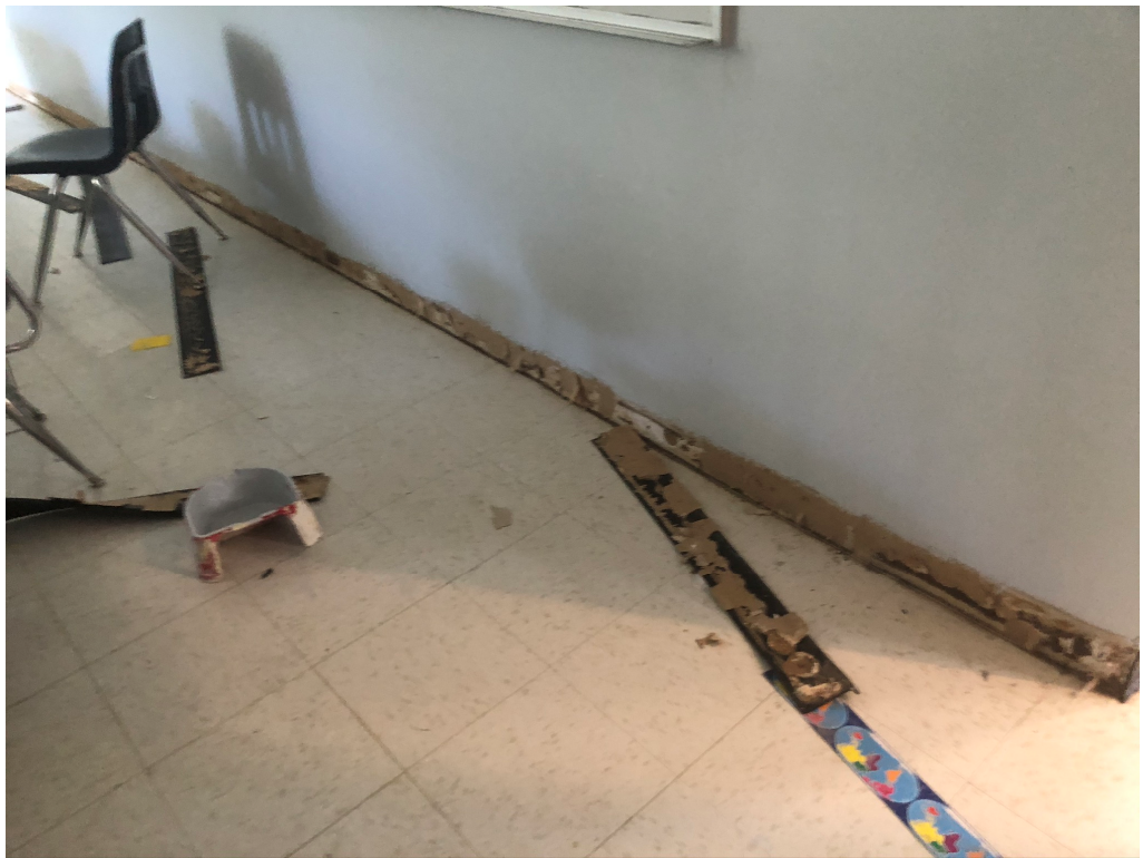
Figure 4 –Base Removal is ongoing
