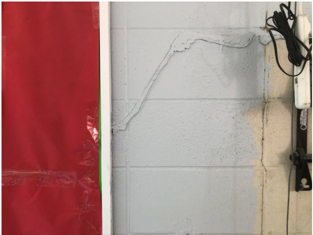
Figure 2 – Glues and adhesives should be removed prior to painting
