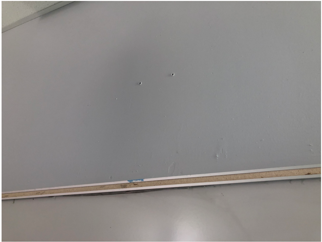
Figure 3 – Holes should be filled prior to painting
