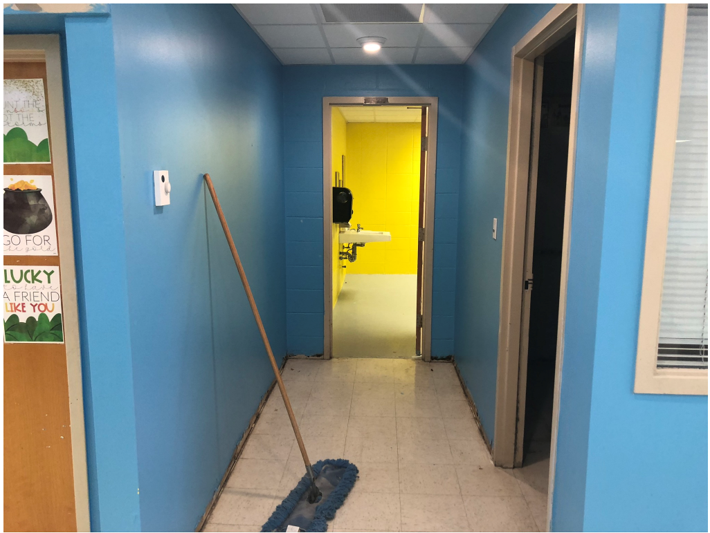
Figure 5 – North Side of Building 3 Bathroom Hall
