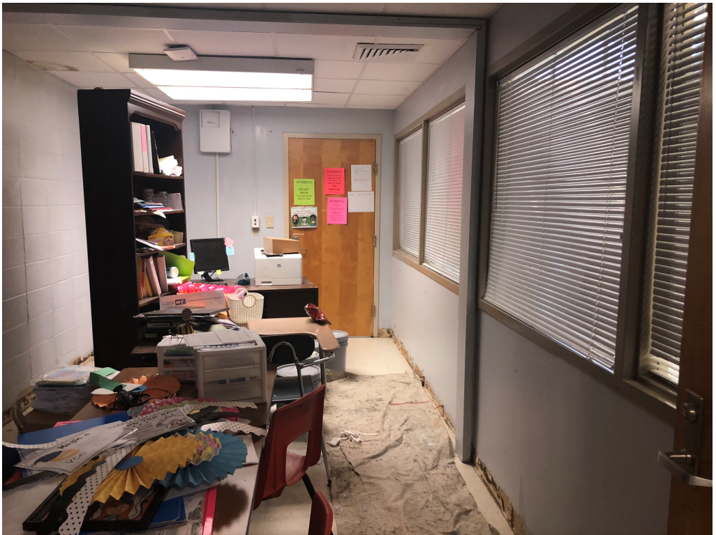
Figure 8 – North Admin Rooms
