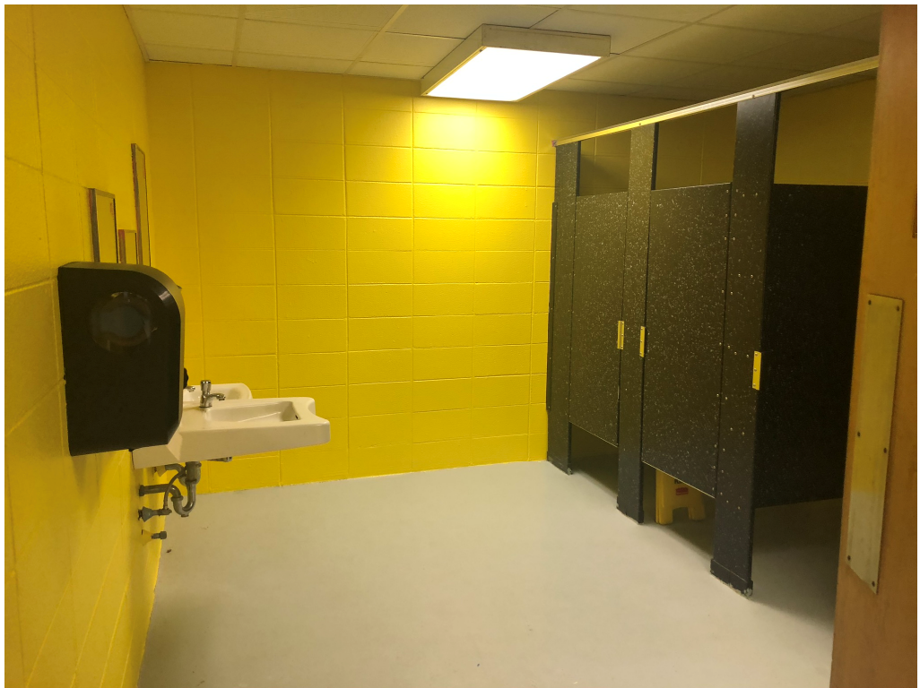
Figure 6 – North Bathroom Painted
