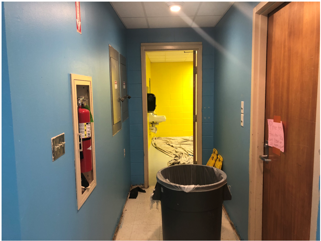
Figure 11 – South Bathroom Area
