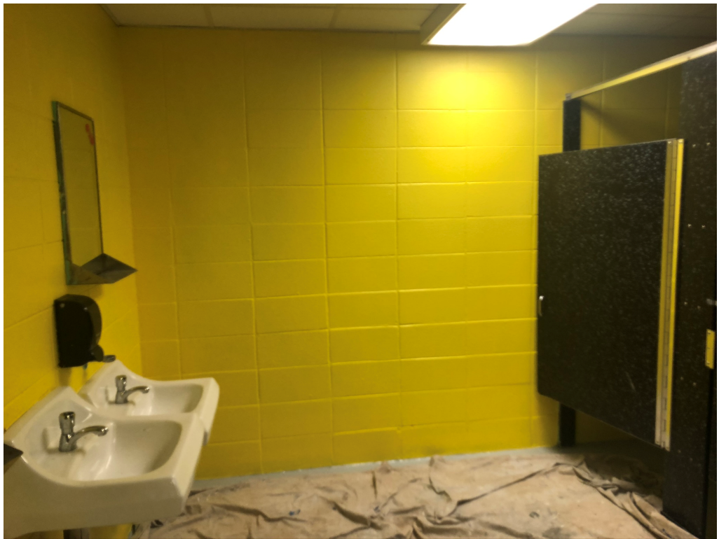
Figure 12 – Bathroom Painting Ongoing
