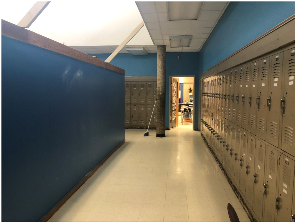
Figure 9 – SW Section of Building 3
