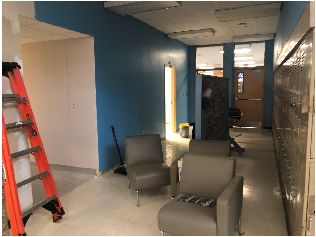
Figure 13 – East Section of Building 3
