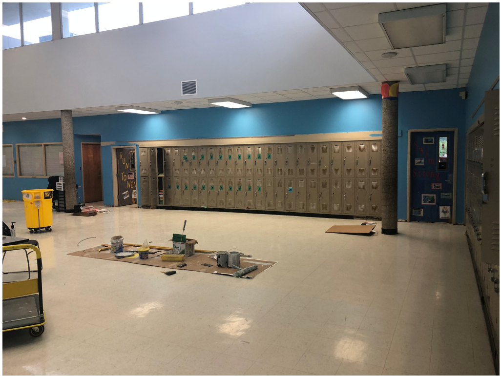
Figure 1 – Building 3 North Space
