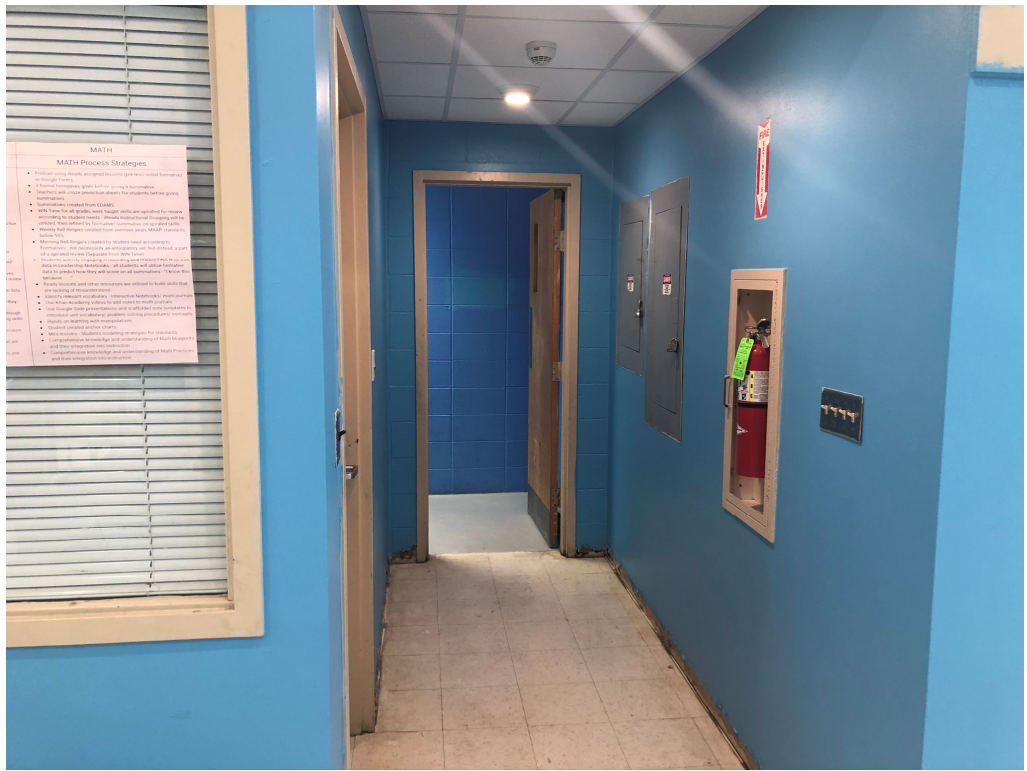
Figure 3 – North Side of Building 3 Bathroom Hall
