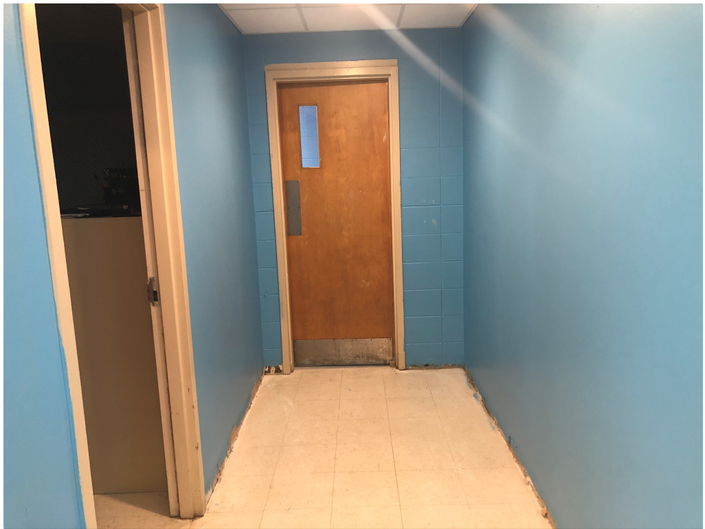
Figure 10 – South Bathroom Area
