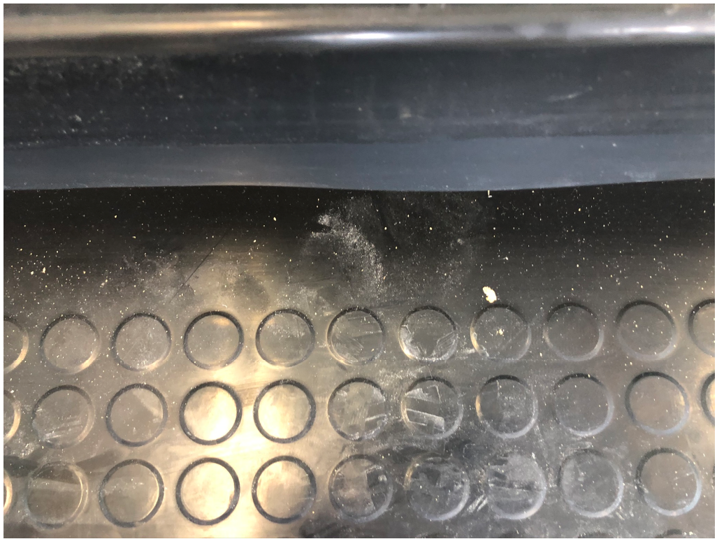
Figure 1 – Rubber Face is Not fully adhered to Step and appears wavy
