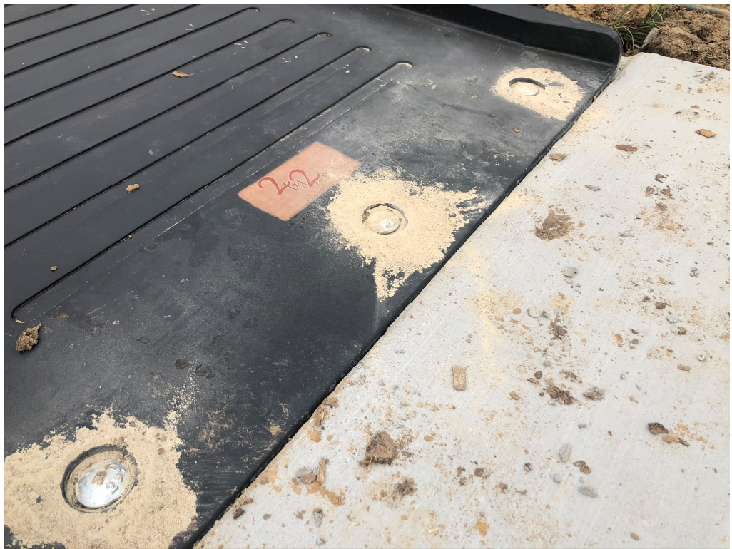
Figure 6 – Ramps Secured
