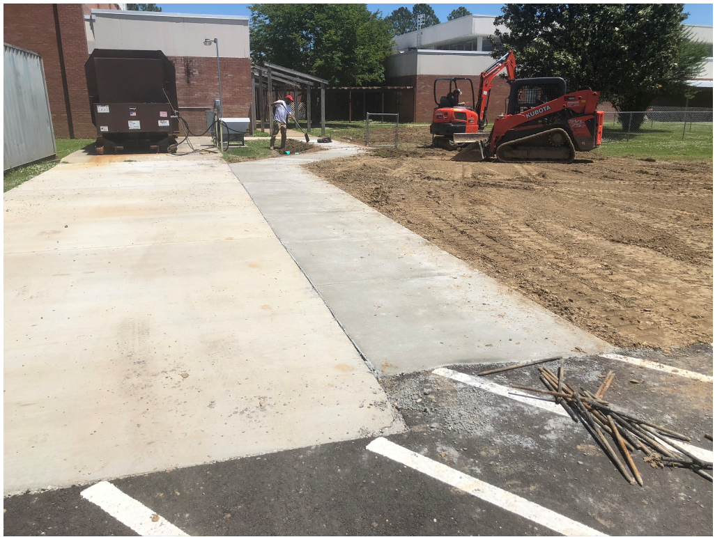
Figure 5 – New Concrete at Dumpster to Building 1
