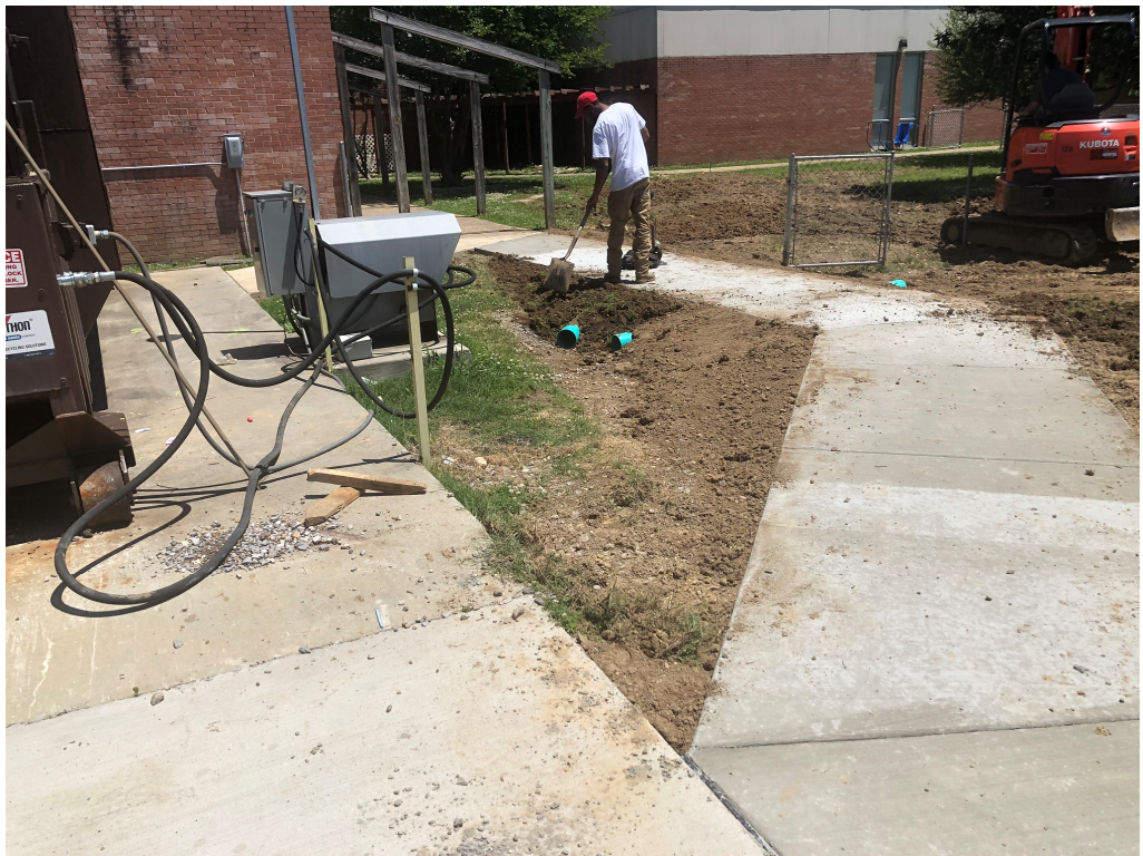
Figure 6 – Drain Pipe Installed Here
