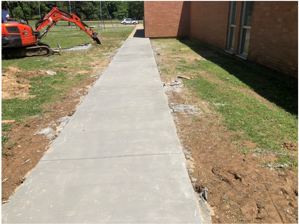
Figure 7 – New Concrete at Building 3 West End
