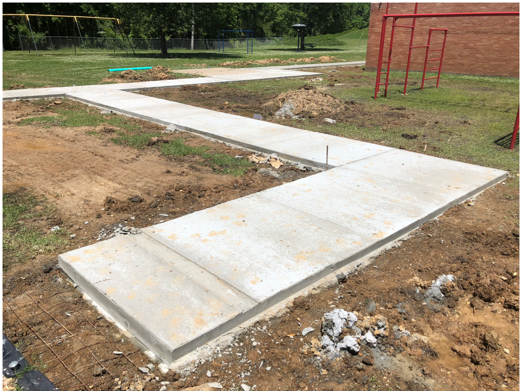
Figure 8 – New Walk Configured for Intersection of plastic ramp to be installed
