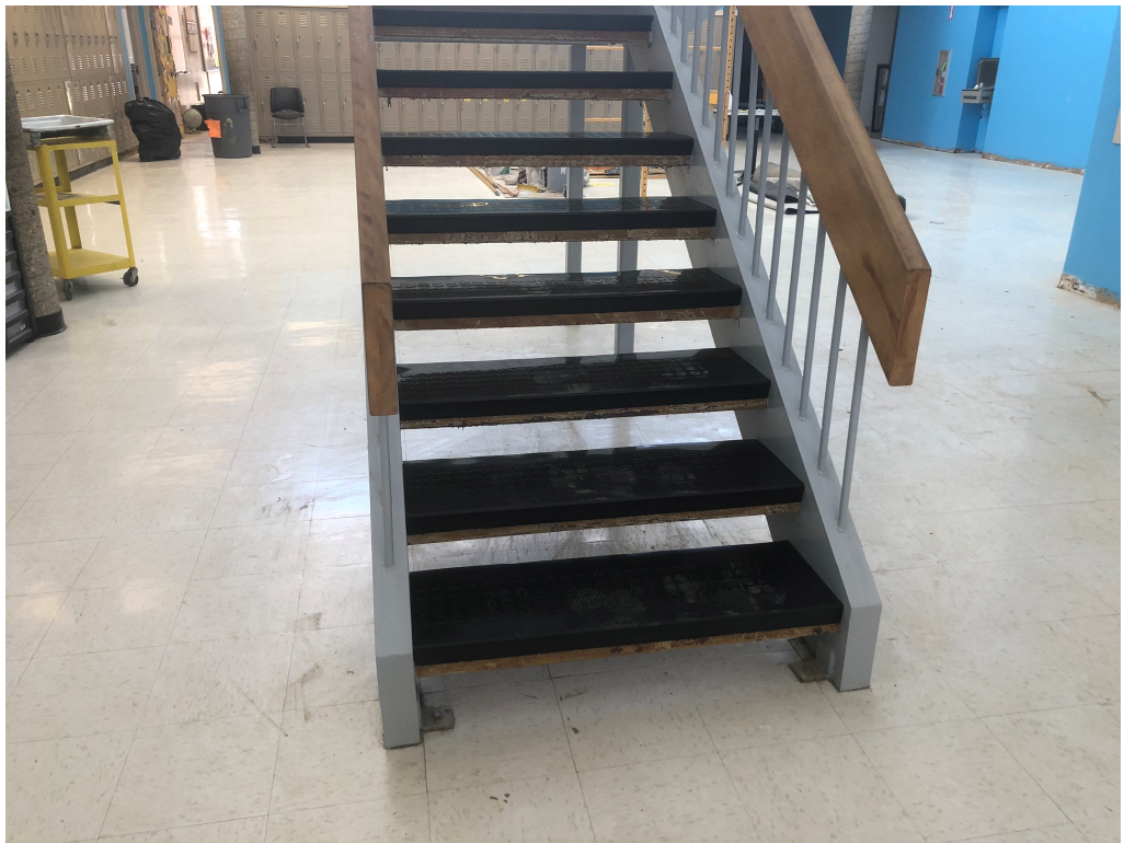
Figure 1 – Stair Treads Installed
