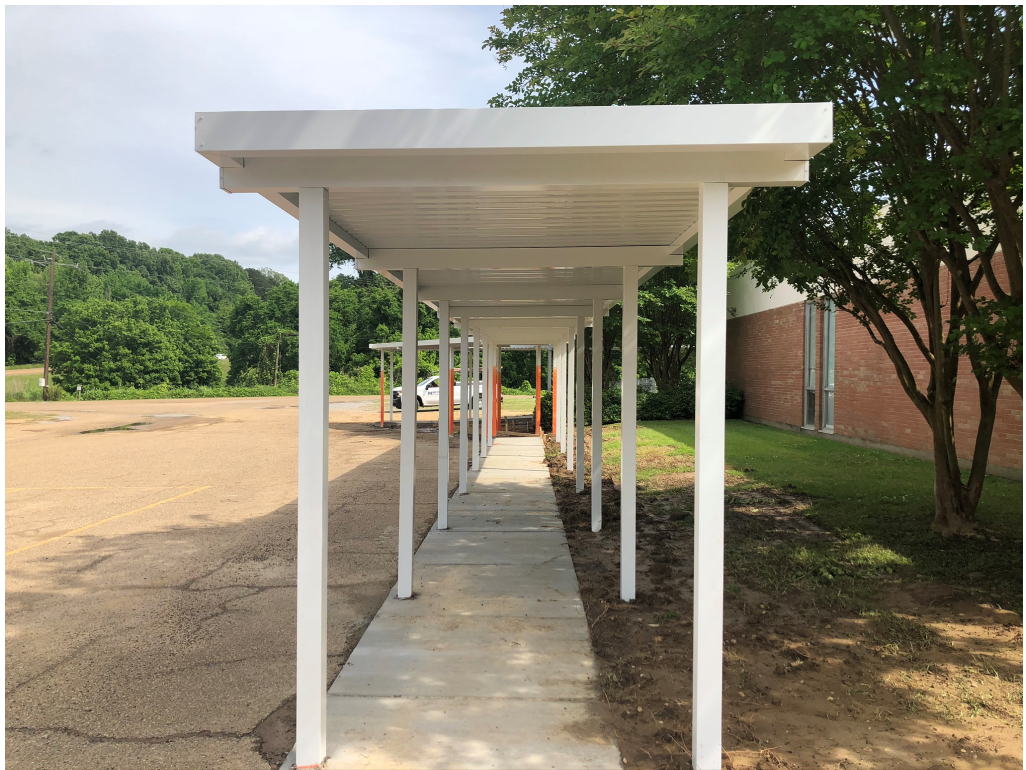
Figure 2 – Extent of Metal Awning
