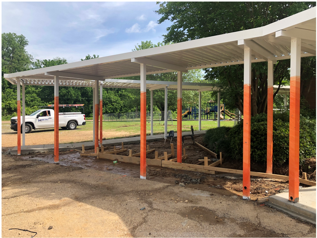
Figure 3 – Concrete Forming
