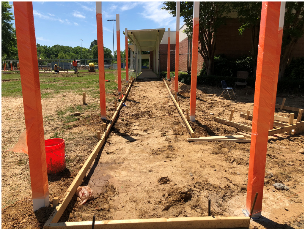
Figure 5 – Concrete Formwork
