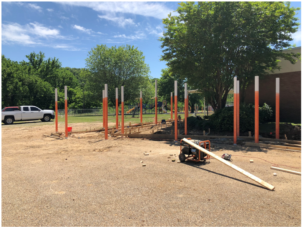
Figure 1 – Columns set and protected
