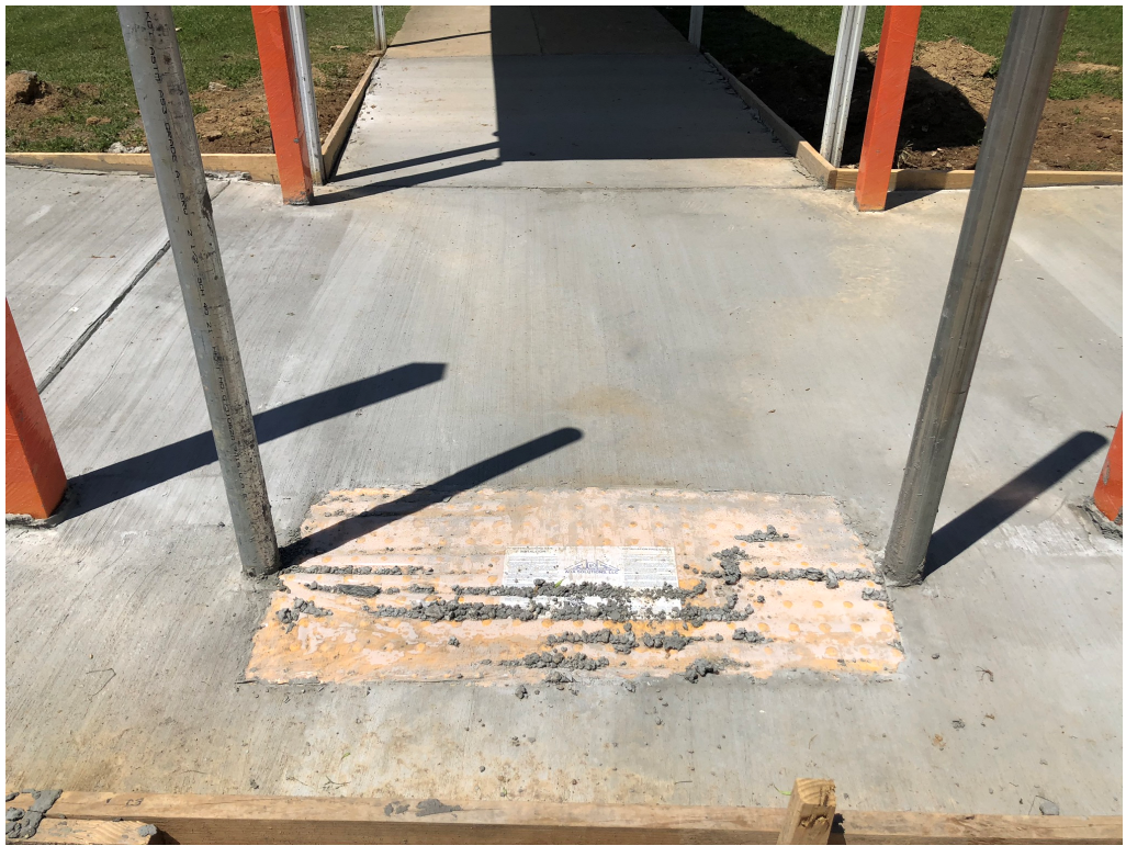
Figure 7 – Tread Inset to concrete and Protected
