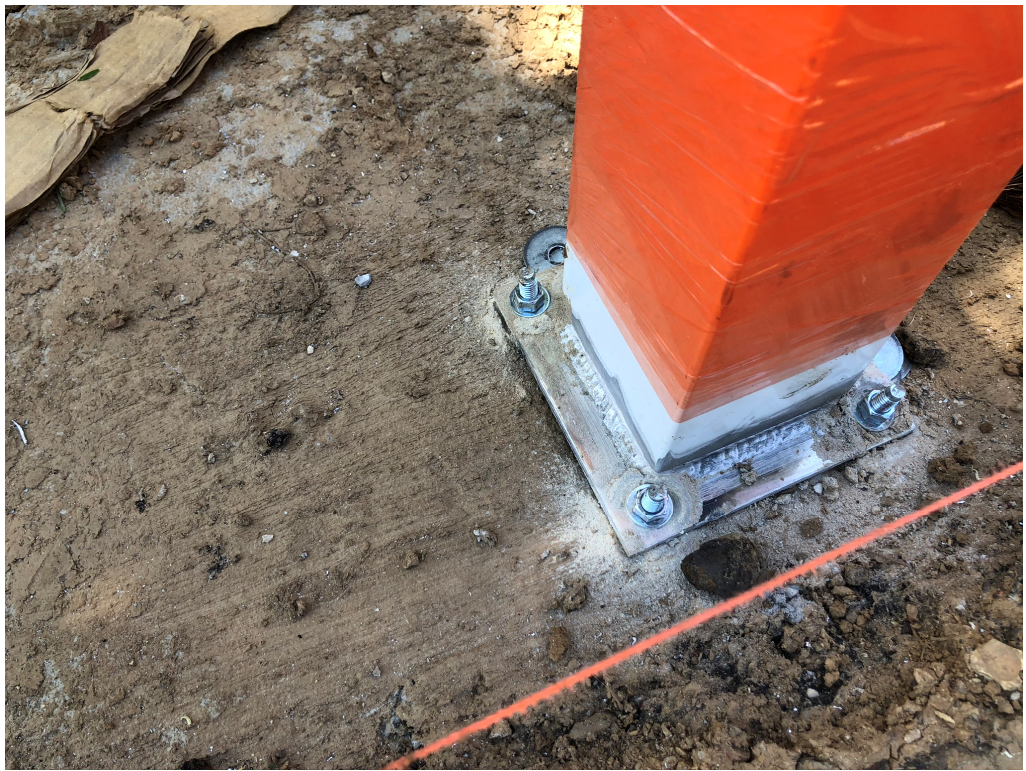
Figure 3 – Columns Base Attachment detail
