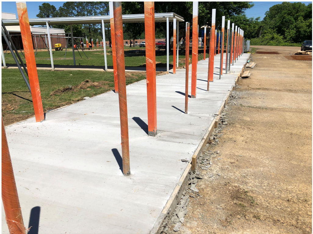
Figure 8 – Concrete with brushed finish poured
