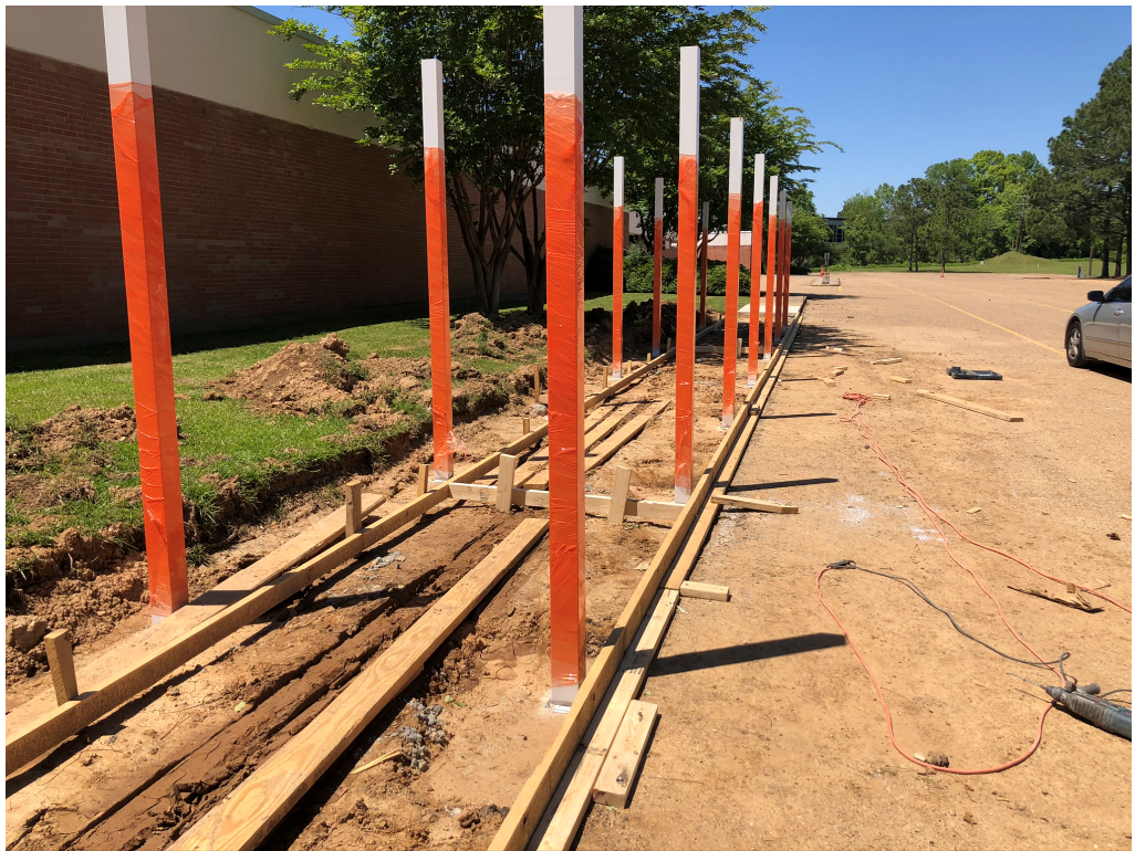
Figure 2 – Columns set and protected
