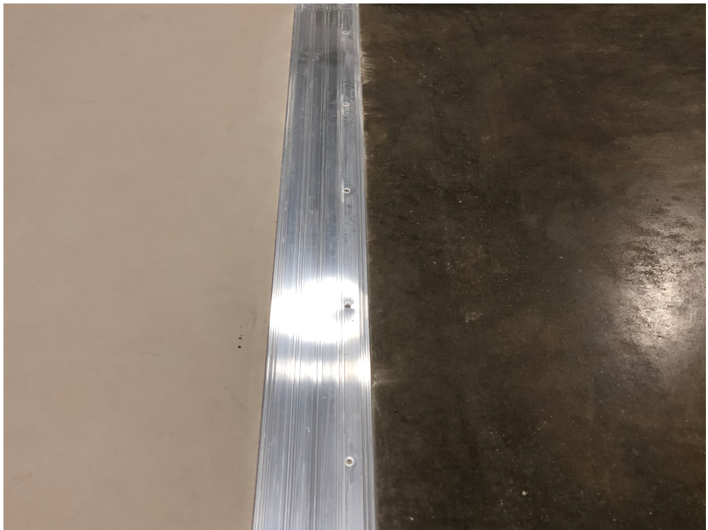
Figure 4 – Threshold Installed at Gym Floor
