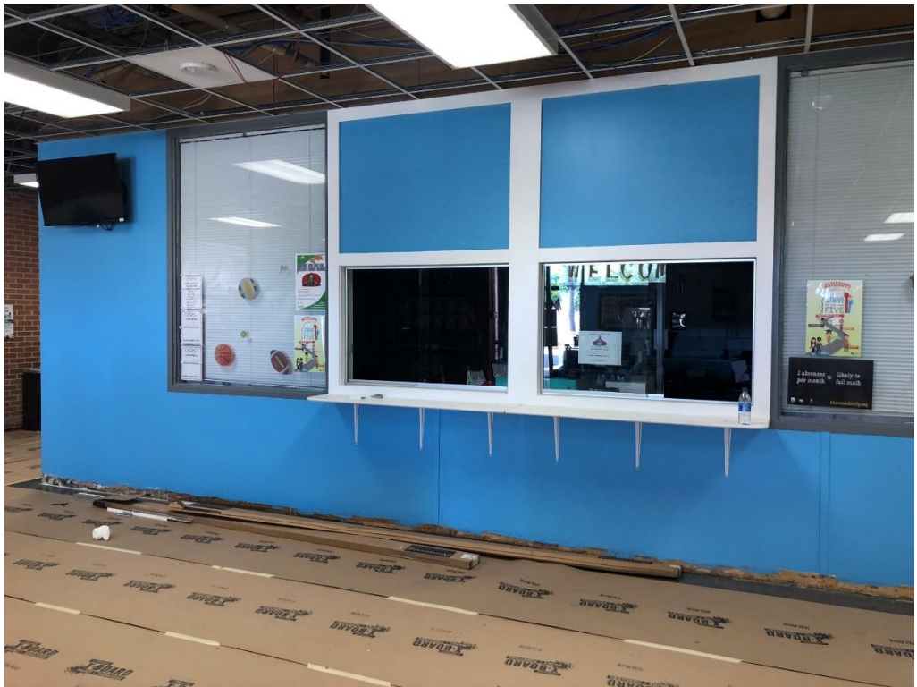
Figure 4 – Main Lobby Paint Complete
