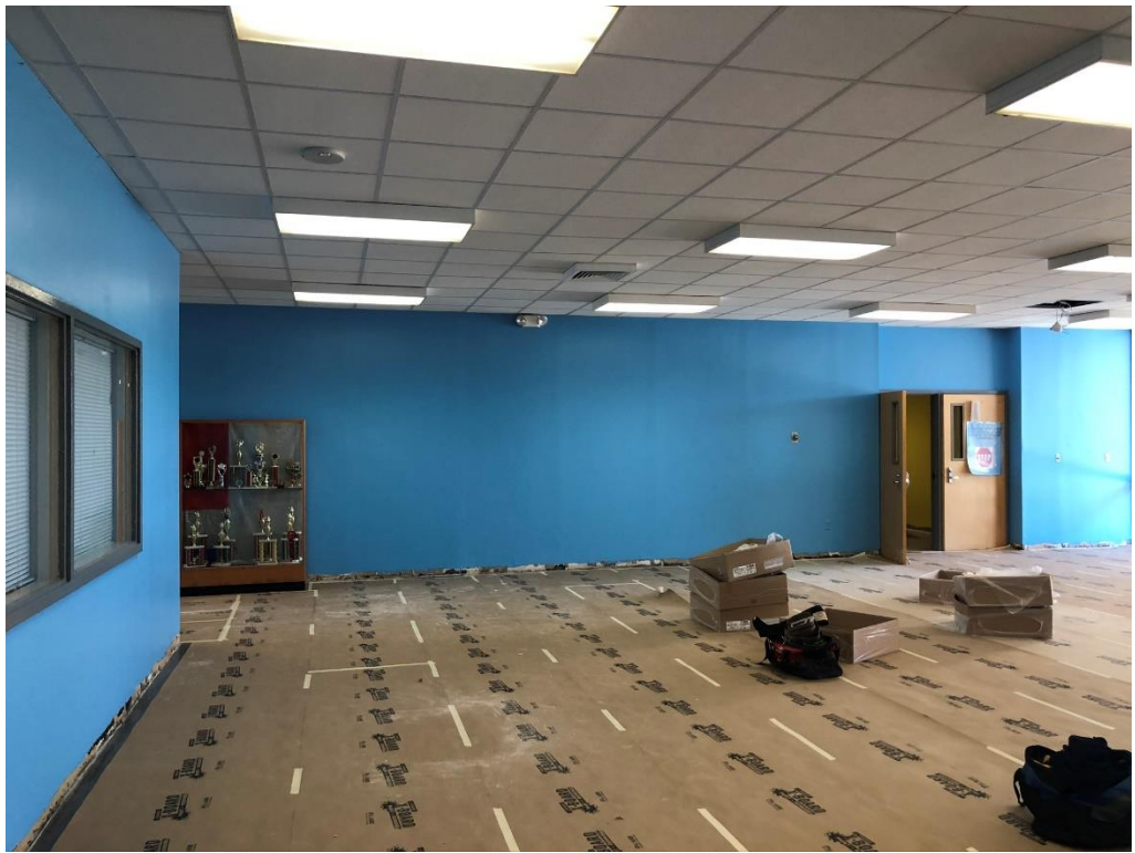
Figure 9 – East Lobby Ceiling Complete (S Corner Looking NW)
