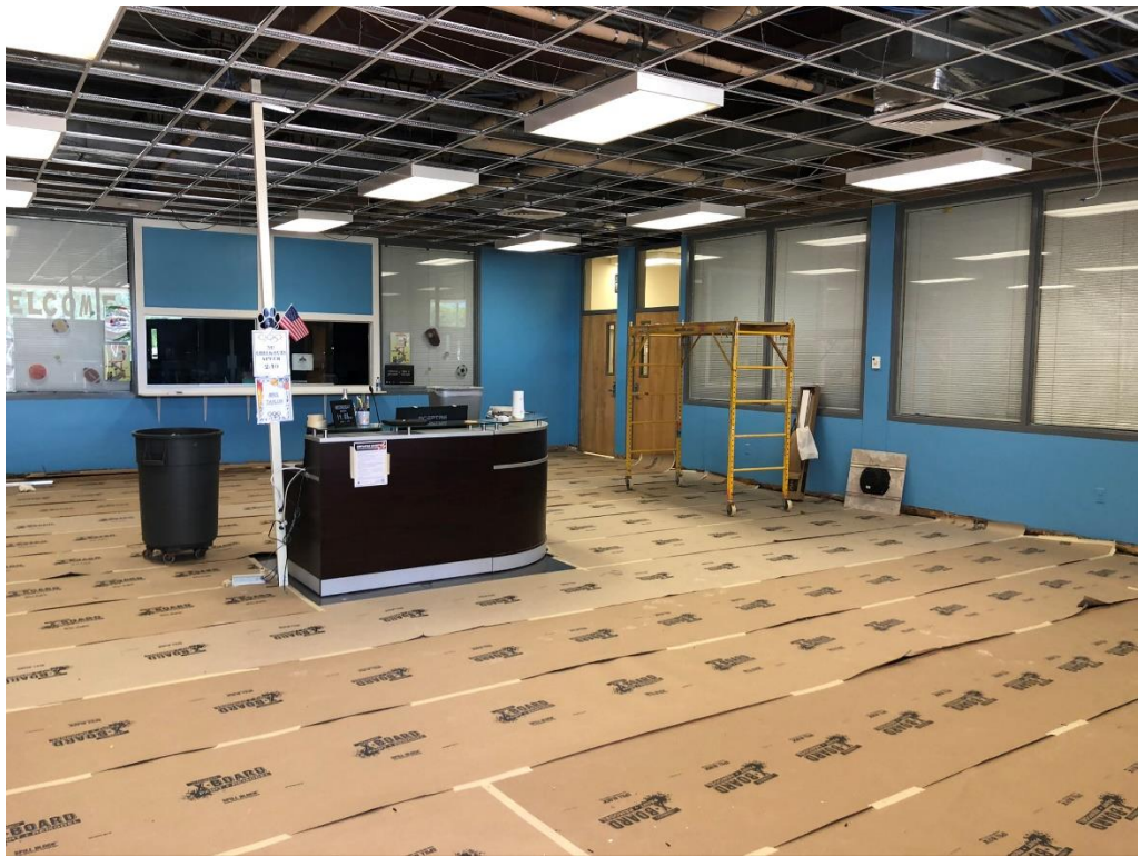
Figure 1 – Main Lobby Ceiling Grid
