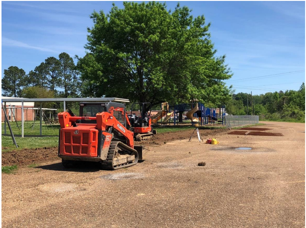
Figure 14 – Demo and Layout Work At SE Covered Drop Off
