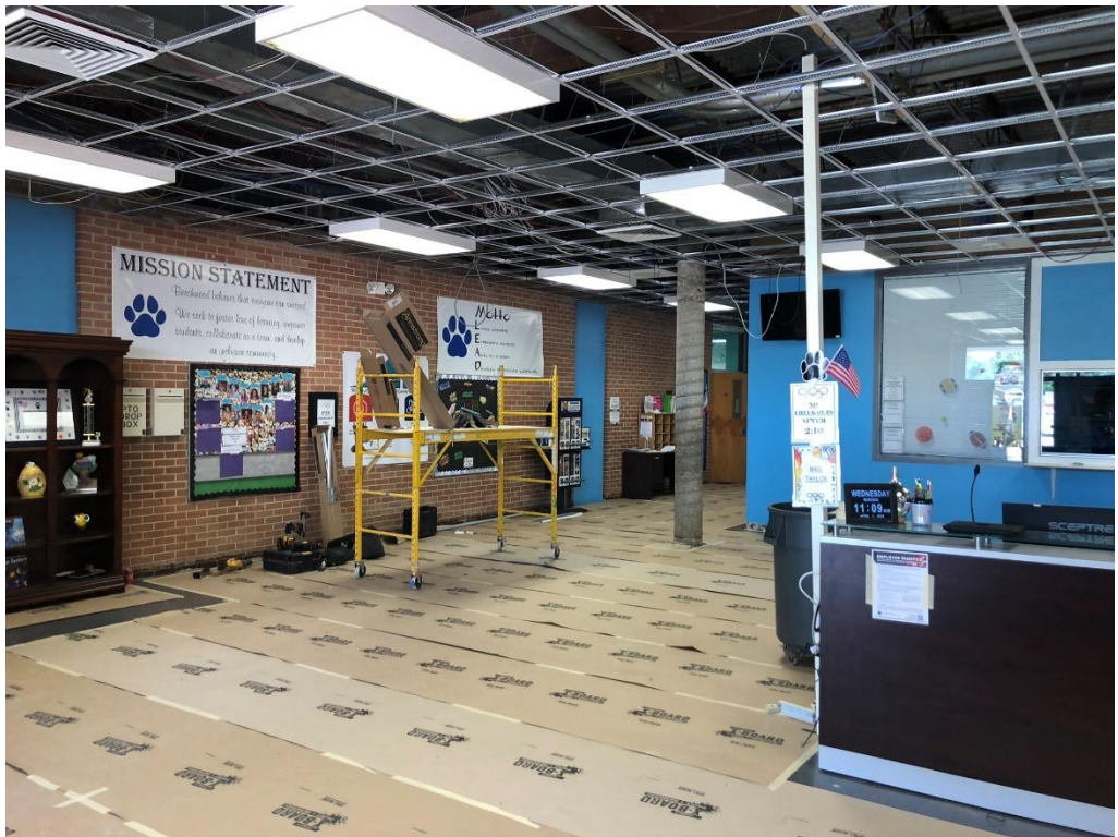
Figure 2 – Main Lobby Ceiling Grid
