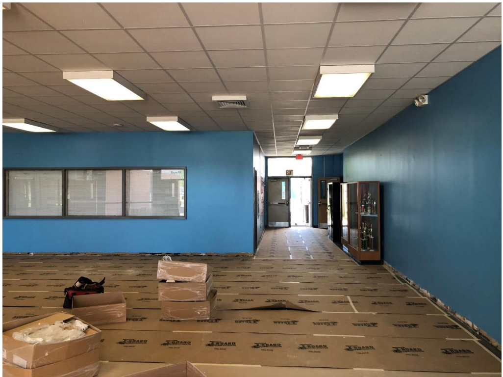
Figure 8 – East Lobby Ceiling Complete (N Corner Looking SW)
