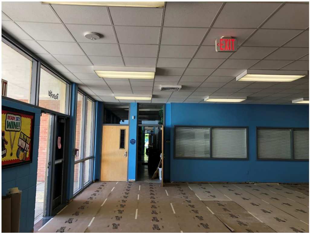
Figure 7 – East Lobby Ceiling Complete (N Corner Looking SE)
