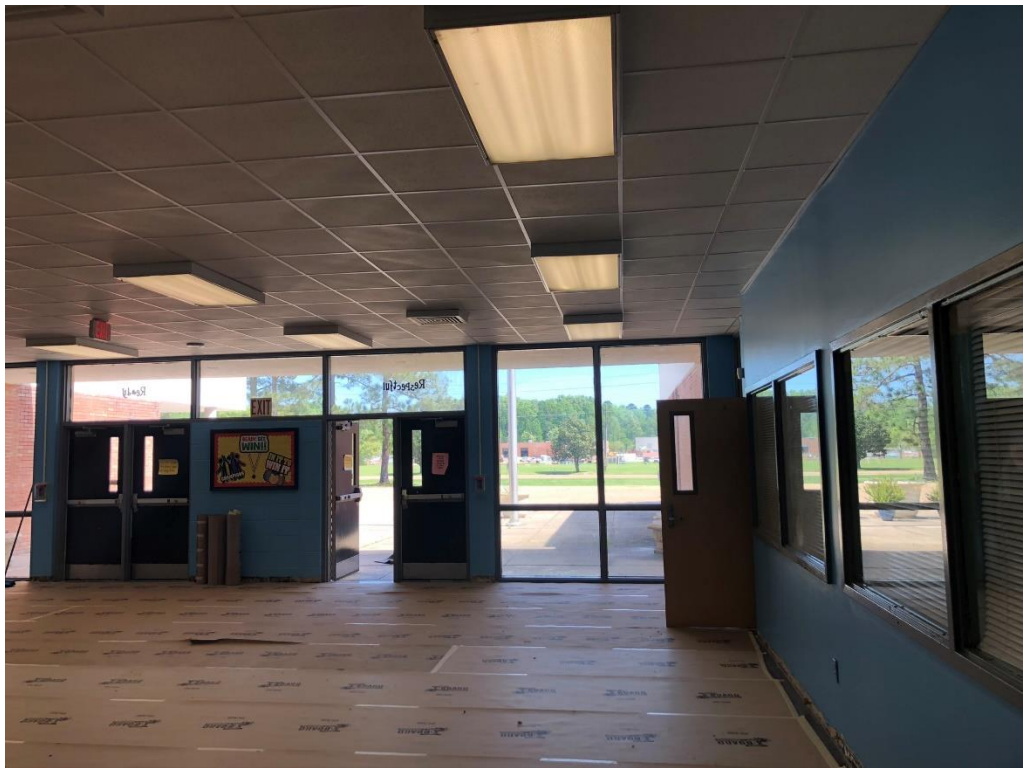
Figure 10 – East Lobby Ceiling Complete (S Corner Looking NE)
